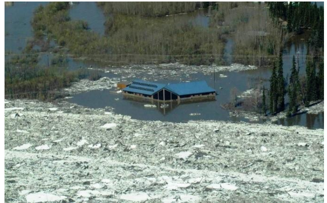
Figure 1. Flooding in Galena in 2013.
