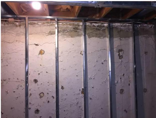
*Figure 2. A crumbling foundation due to pyrrhotite in the concrete.*
