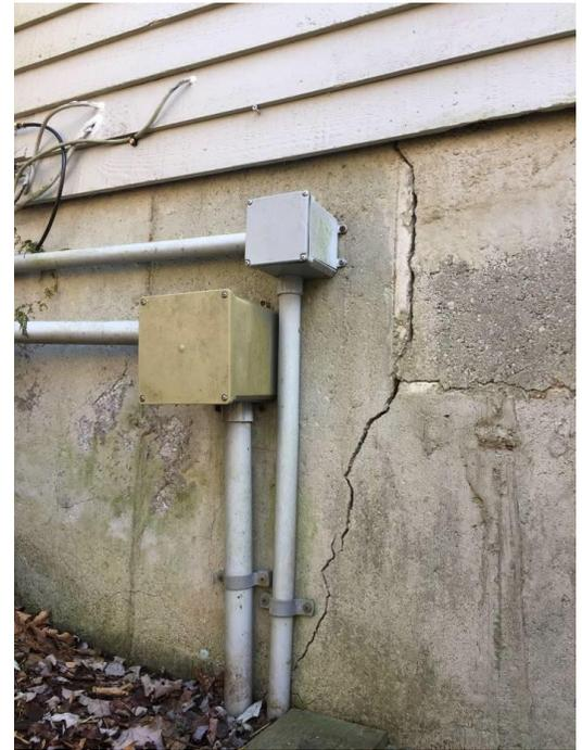
Figure 1. A crack in a home's foundation caused by pyrrhotite in the concrete.
