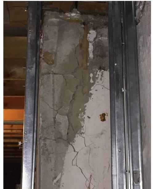
*Figure 3. A crumbling foundation caused by the presence of pyrrhotite.*
