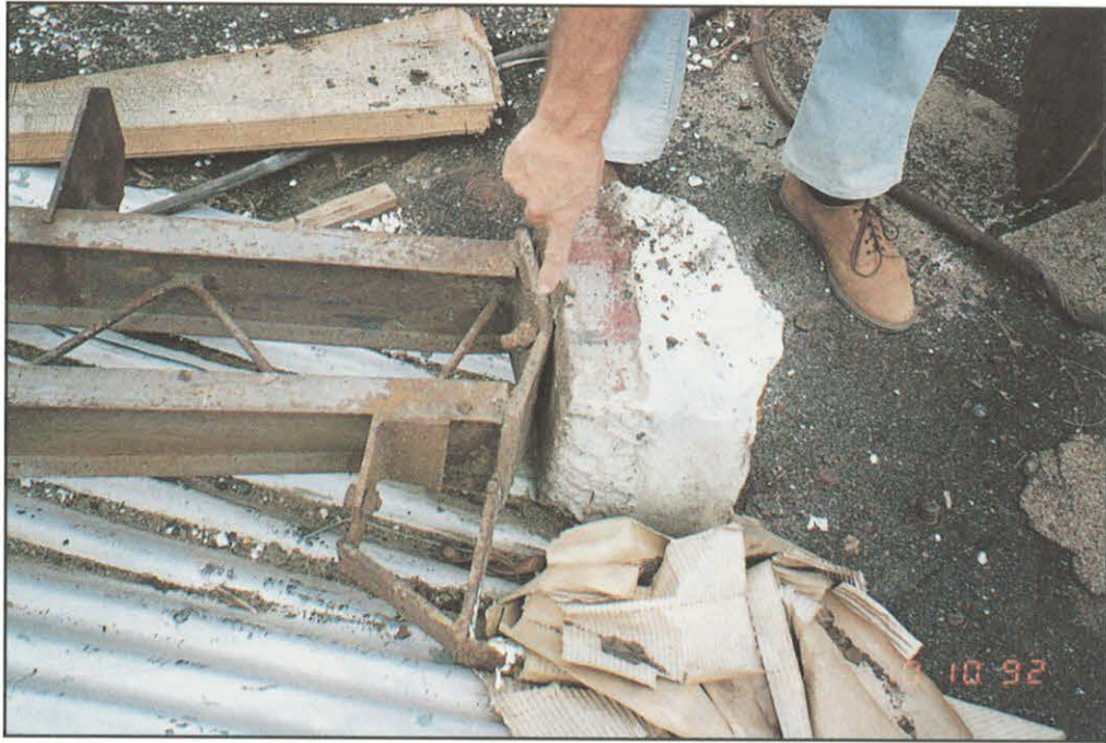
FIGURE 58. Failure of steel warehouse due to age and weatherization and insufficient anchorage to resist uplift.
