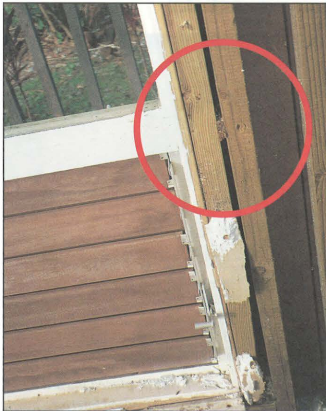
FIGURE 50. Improper attachment of window unit. Note only one connection (nailing) point between unit and wall structure at the single shim.
