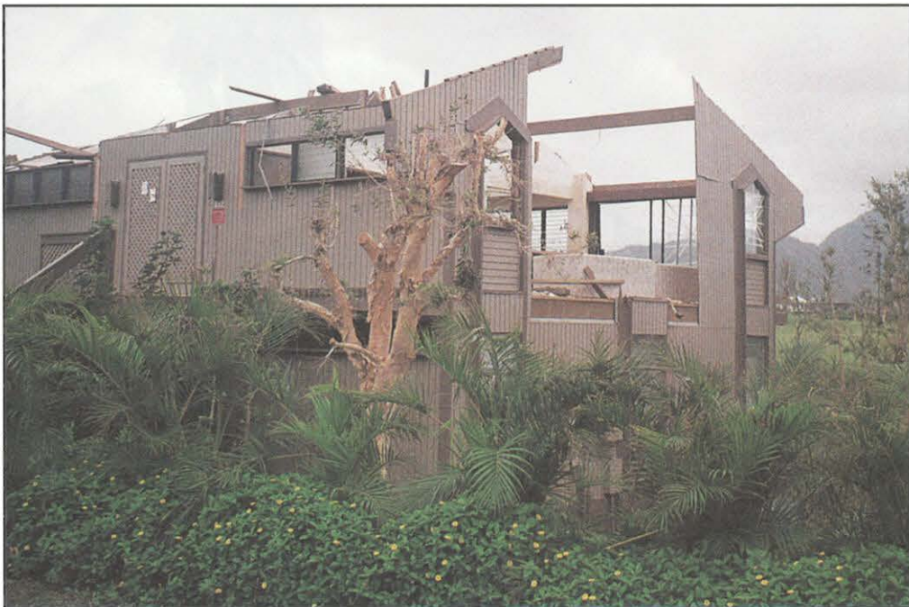
FIGURE 31. Gable-end roof designs tended to be more failure-prone.
