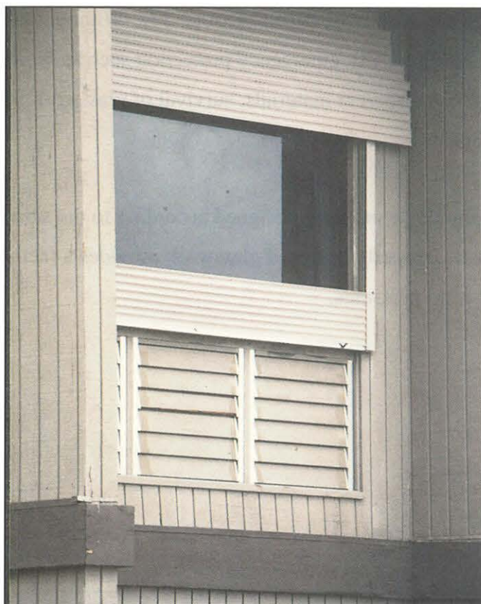
FIGURE 54. In-place protective devices for glazing reduced the occurrence of building envelope failures.
