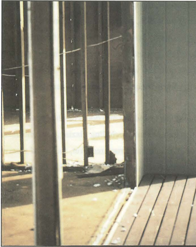
FIGURE 51. Improper connection of sliding glass door. Track attached with only three screws in vertical member. Sliding track on floor attached with caulk only.
