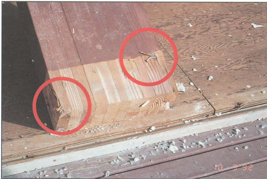
FIGURE 23. Toenailing of ridge beam to gable-end support. Roof failure from uplift.
