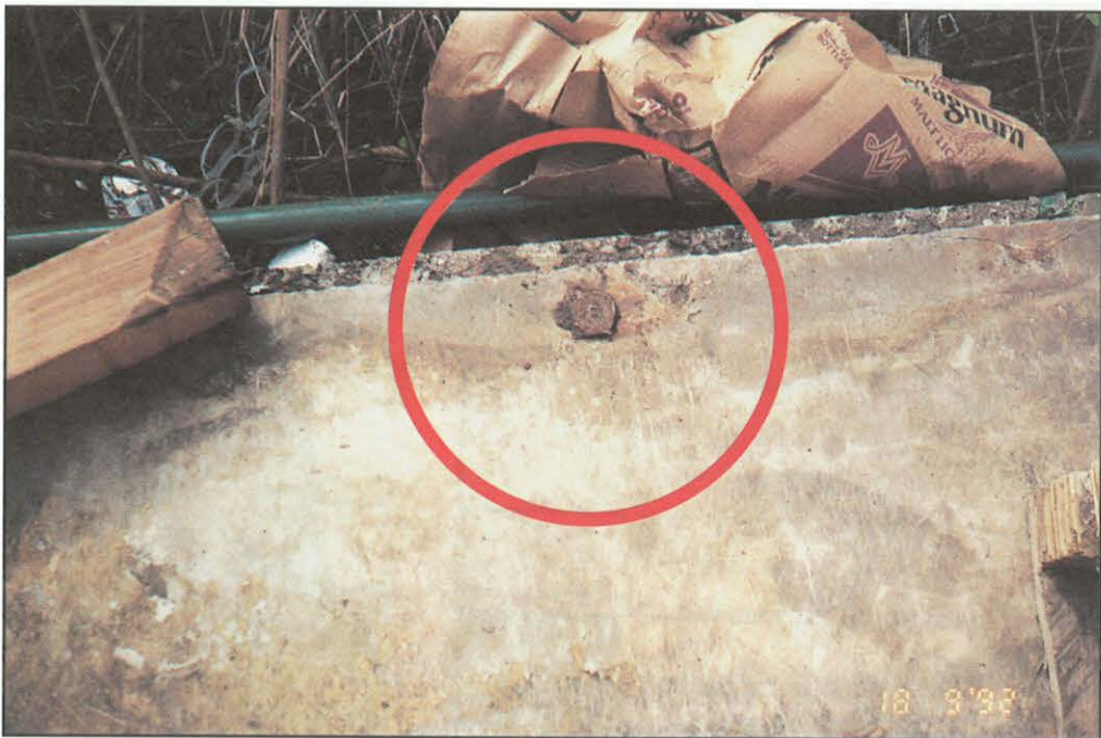
FIGURE 59. Steel warehouse, sill-to-concrete-foundation failure at anchoring points.
