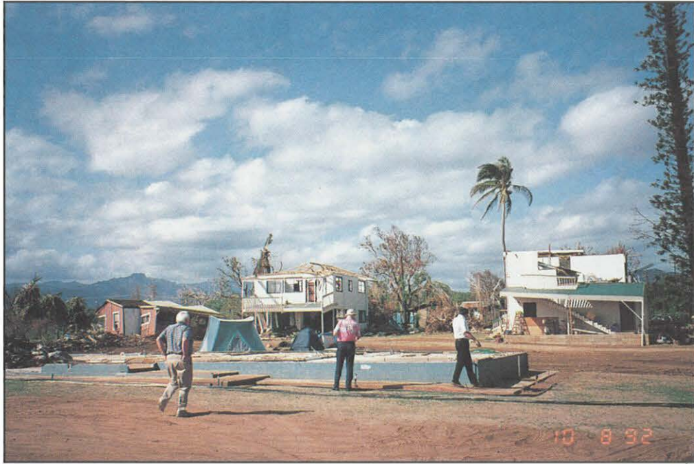
FIGURE 8. Typical example of residential construction along Poipu Beach that was destroyed because it was not elevated above the flood hazard.
