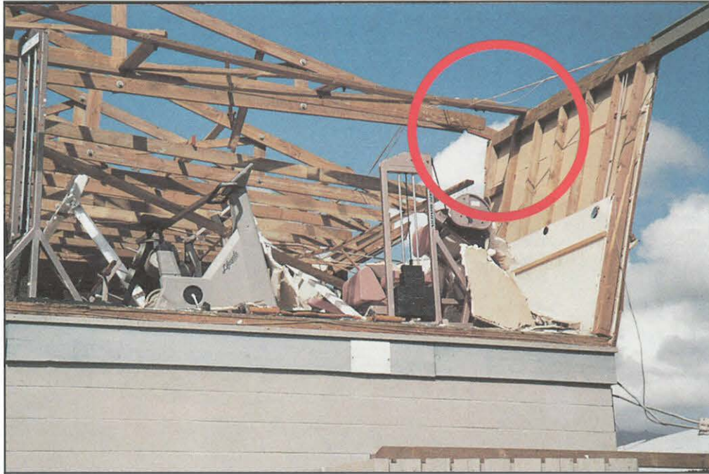
FIGURE 30. Improper connection (toenailing) between roof trusses and wall systems. When roof sheathing was blown off by wind, unbridged trusses failed, as did the exterior wall.
