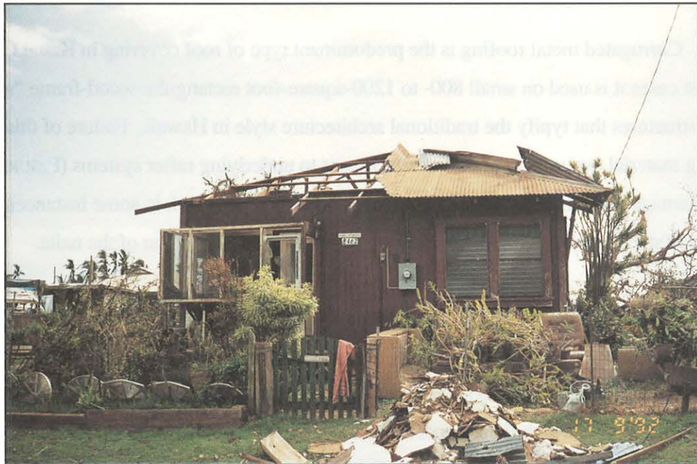
FIGURE 42. Failure of corrugated metal roof at attachment points. These small, geometrically stable, “single wall,” rectangular structures with numerous interior partition walls often remained structurally intact after loss of metal coverings.
