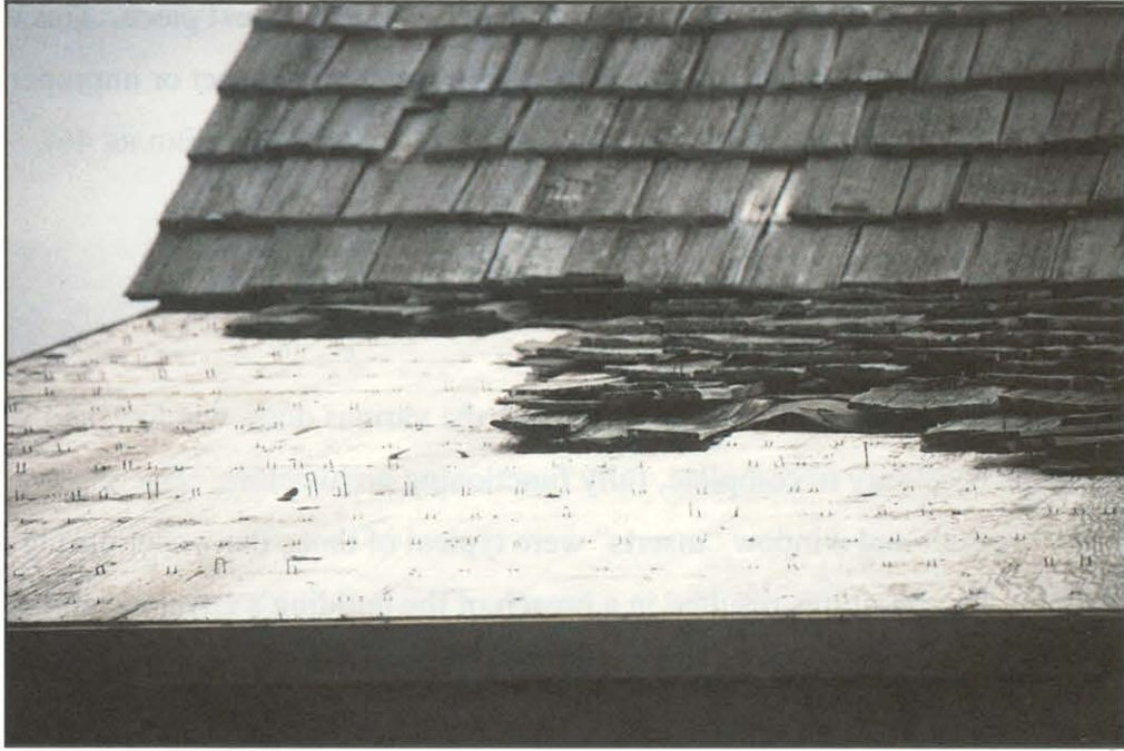
FIGURE 44. Loss of roof cladding due to failure at attachment points. Notice that many staple crowns have corroded away on staples used to attach wood shake roofing to plywood roof sheathing.
