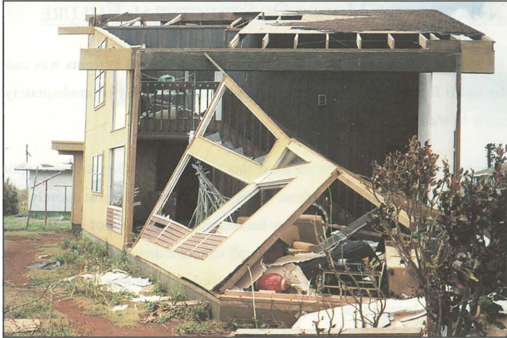
FIGURE 21. Once the roof system is compromised, the ability of the wood-frame exterior walls to withstand external wind pressure is greatly diminished.
