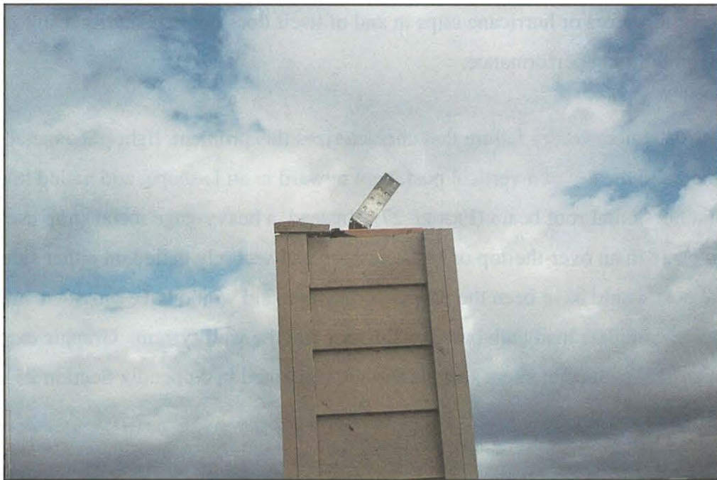
FIGURE 26. Example of improperly sized and placed metal fastener, which led to roof failure from wind uplift forces.
