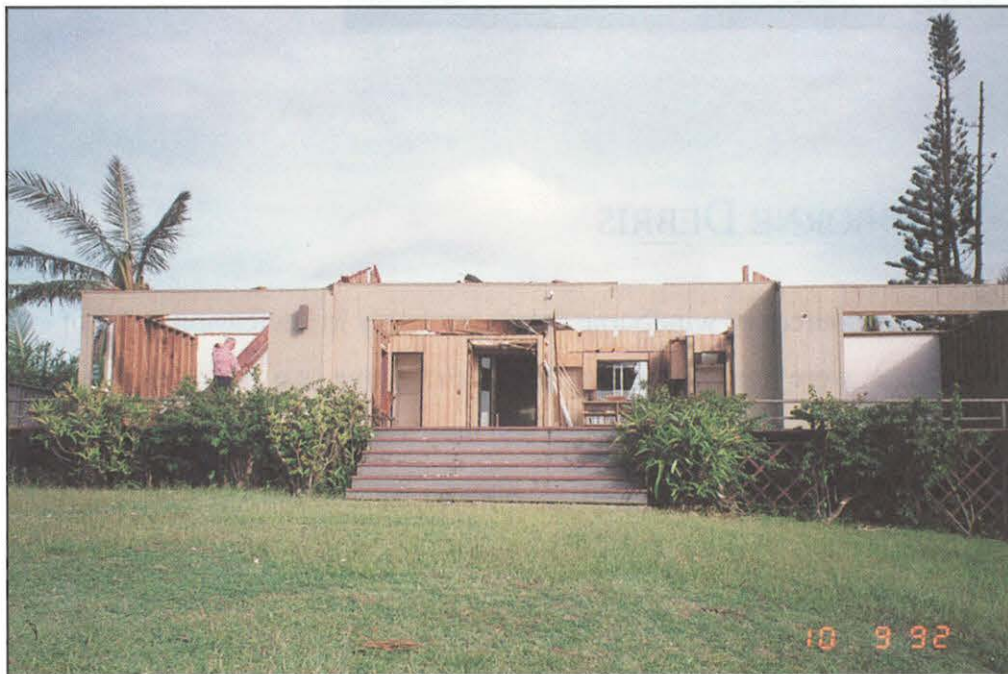
FIGURE 53. Extensive use of glazing on windward side can significantly compromise a building's envelope and lead to roof failure.
