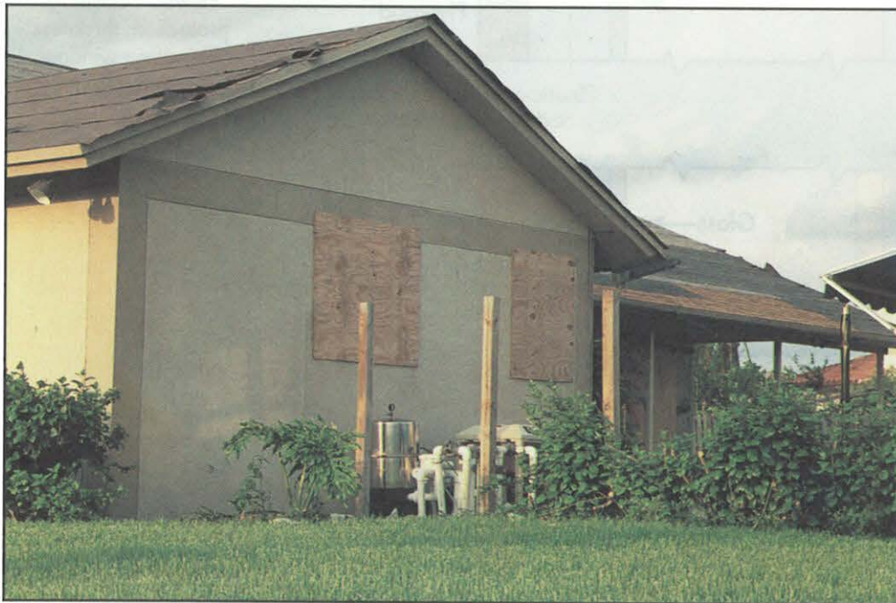
FIGURE 90. Plywood used as openings protection installed. See Figure 91 for details.
