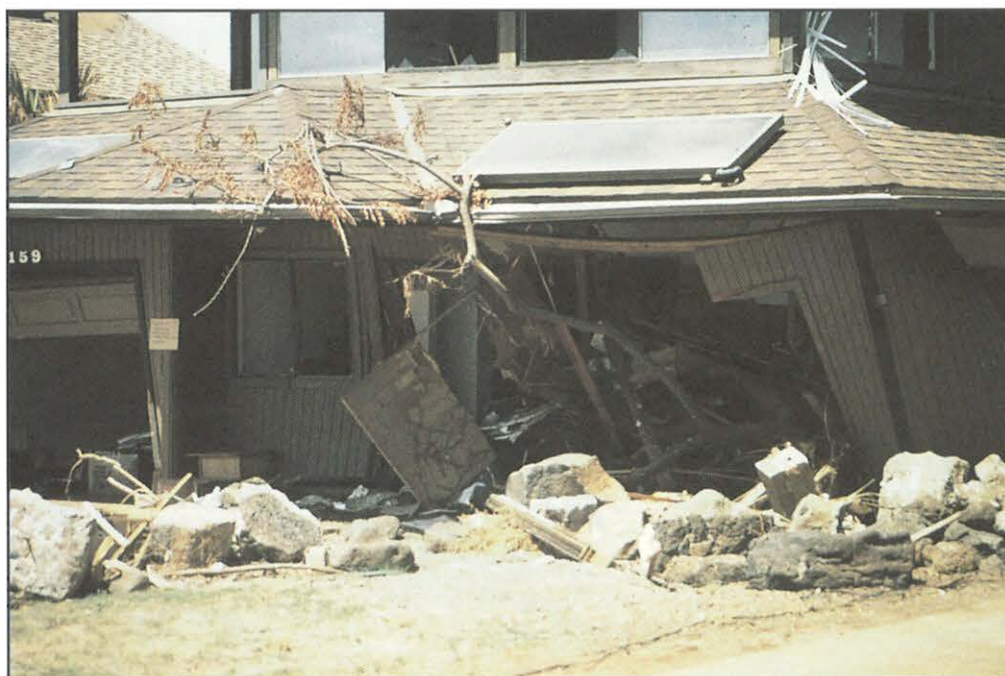
FIGURE 18. Waterborne lava rock projectiles at Poipu Beach increased damage to non-elevated buildings.
