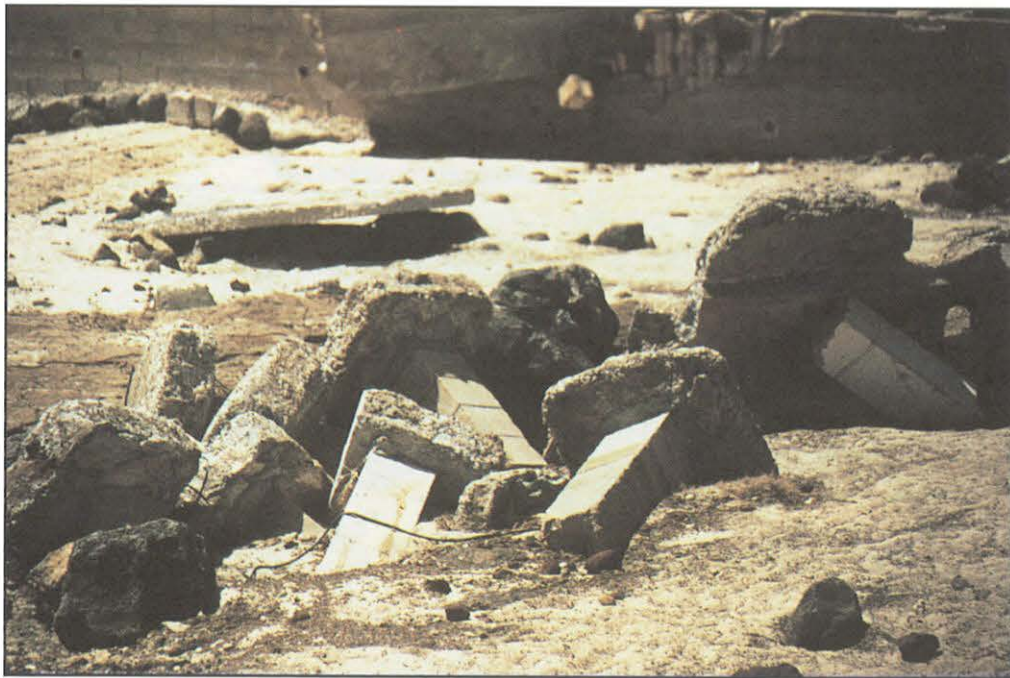
FIGURE 16. Undermining of shallow pier foundation at Poipu Beach due to lack of sufficient embedment below erosion depth.
