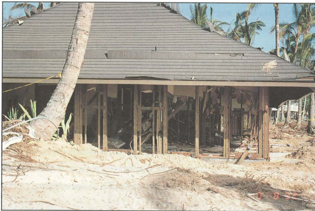
FIGURE 14. Interior of non-elevated building at Poipu Beach destroyed by coastal flooding.
