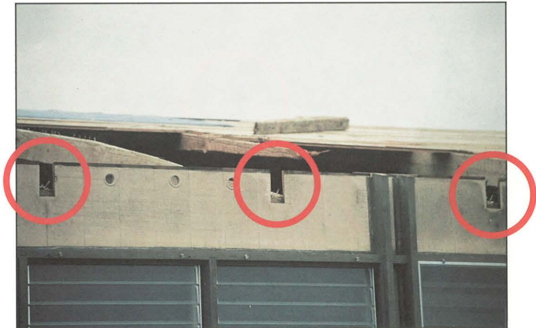
FIGURE 25. Toenailing of roof rafters to wall system. At this critical connection, toenailing does not provide the load transfer path necessary to withstand uplift forces.
