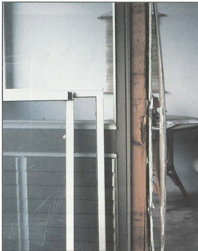
FIGURE 49. Implosion of transparent shatter-resistant sliding door. Failure of door frame due to improper attachment to structural elements.
