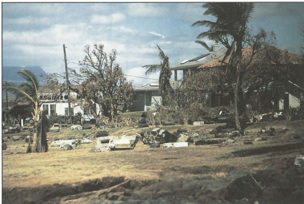
FIGURE 17. Breakup of grouted lava rock walls at Poipu Beach generated waterborne projectiles.
