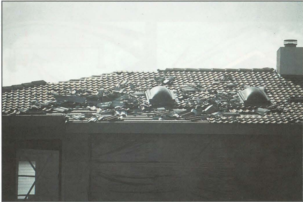
FIGURE 46. Roof cladding system composed of interdependent elements. Failure of one tile led to failure of adjacent tiles in a “chain reaction” effect.
