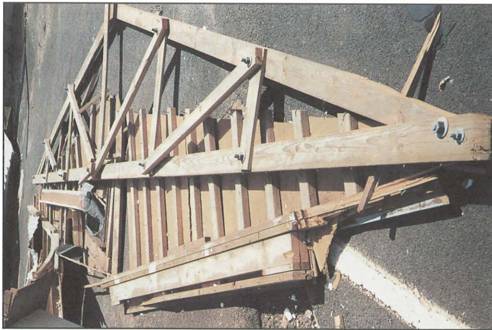
FIGURE 29. Gable-end roof failure due to loss of roof sheathing and lack of gable bracing.
