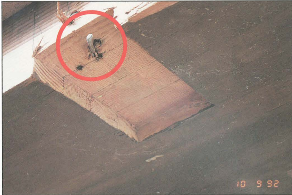
FIGURE 24. Toenailing of rafter to ridge beam. Roof failure from uplift.
