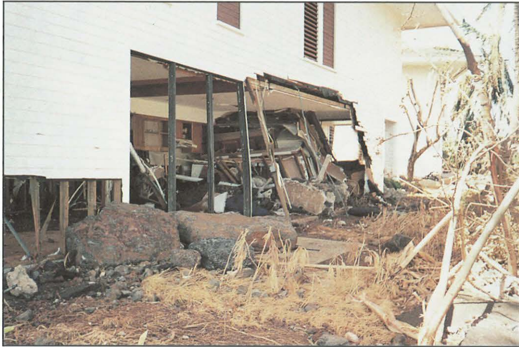
FIGURE 7. Waterborne debris resulted in significant damage to non-elevated buildings along Poipu Beach.
