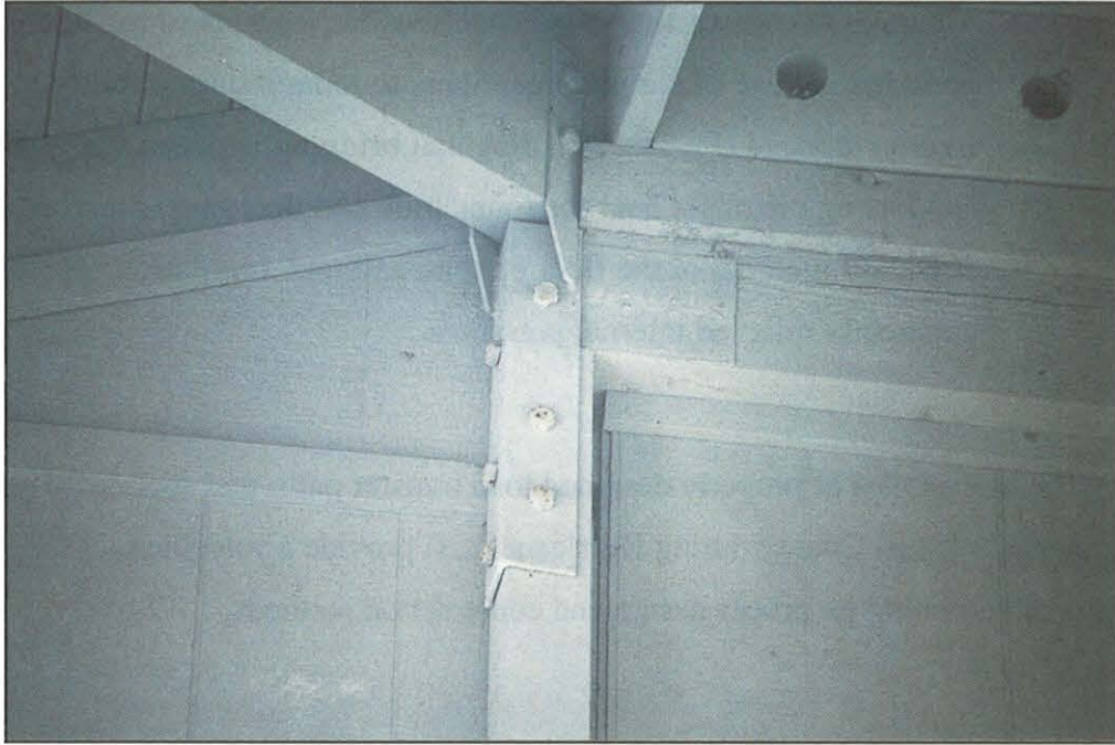
FIGURE 35. Example of very successful heavy-gauge metal fastener connecting roof and wall systems. Note the over the top application and the number and size of lag bolts used for attachment.
