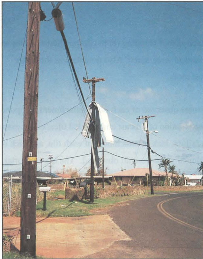
FIGURE 43. Metal roof loss generates large airborne projectiles, which often cause additional damage.
