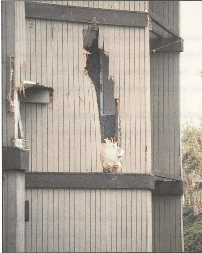
FIGURE 55. Windborne debris impact can puncture building and allow buildup of internal wind pressure.
