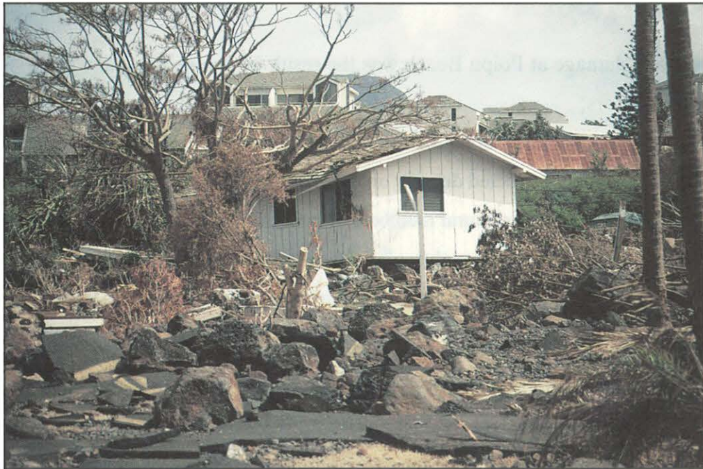
FIGURE 9. Non-elevated house at Poipu Beach that floated off its foundation and was transported well inland.
