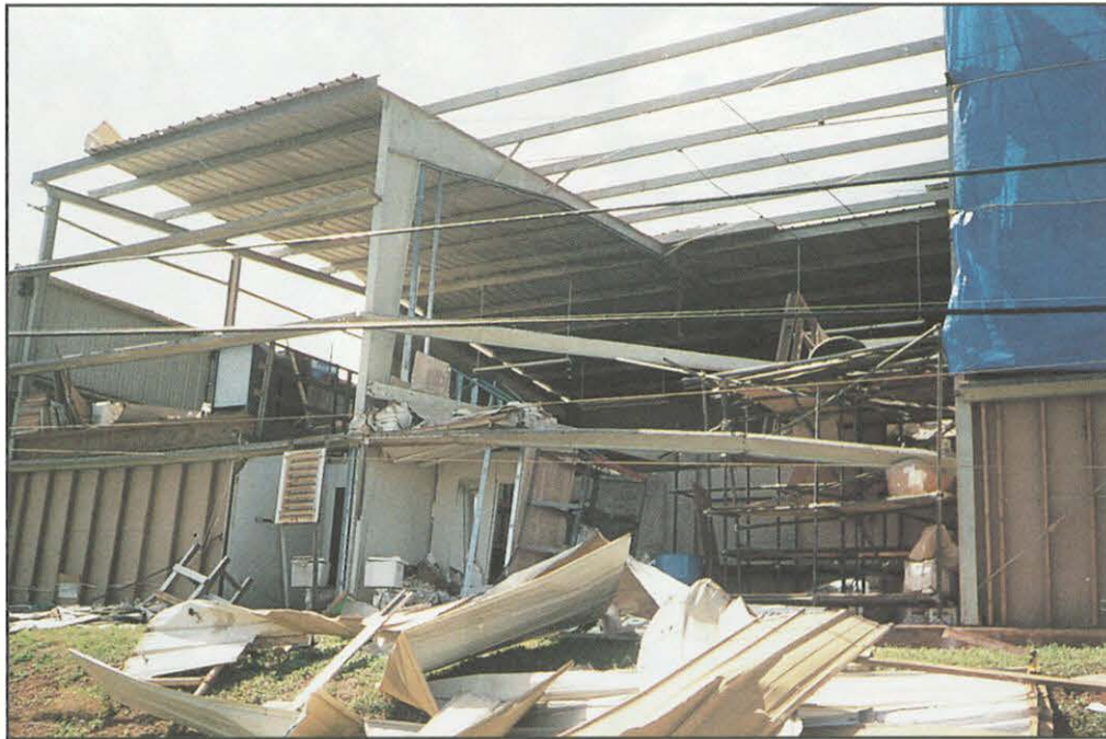
FIGURE 56. Steel warehouse failure commonly was due to loss of light-gauge metal sheet cladding.
