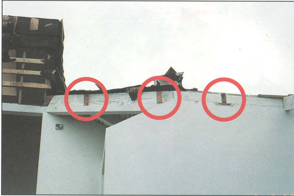
FIGURE 22. Roof rafter construction with simple nailing or toenailing failed under uplift forces. Note two nails used to connect each rafter to hip beam.
