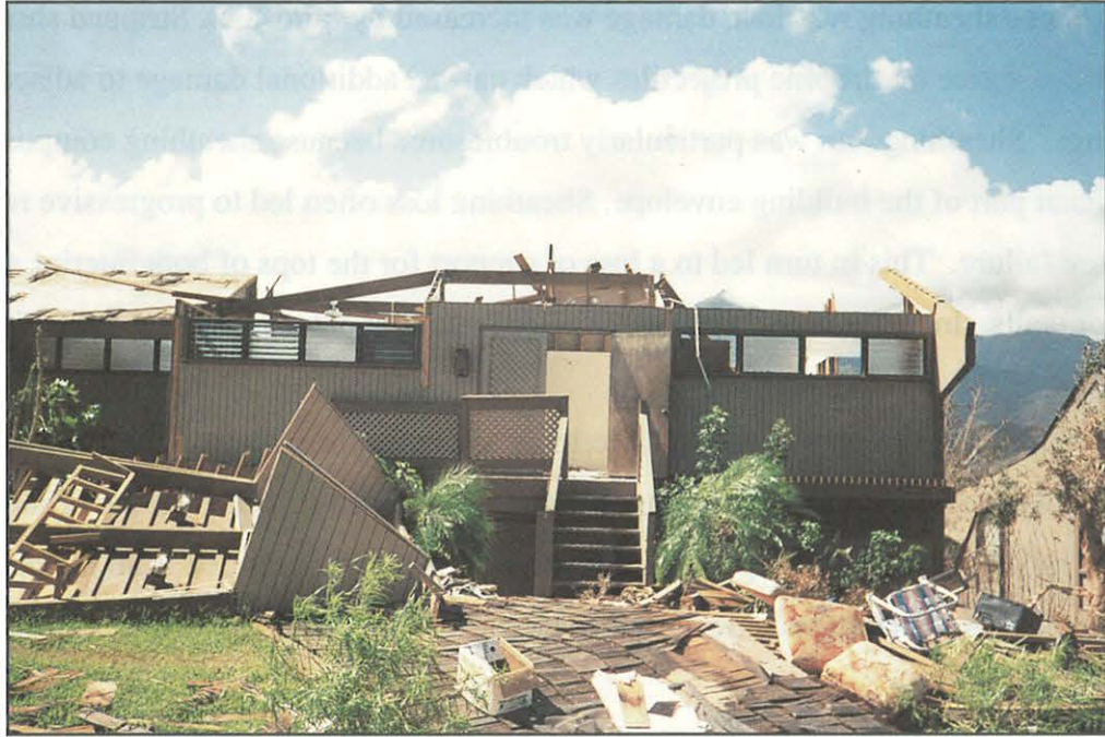
FIGURE 41. Total roof failure due to loss of sheathing.
