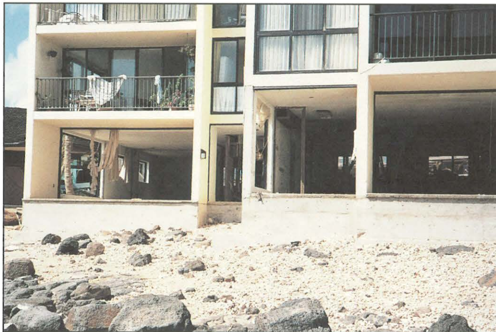
FIGURE 20. Typical non-elevated condominium or hotel. Interiors of lower units destroyed; upper units suffered considerably less flood damage. Elevating a building's lowest floor and keeping lower areas clear to allow passage of velocity water can significantly reduce future flood damage.
