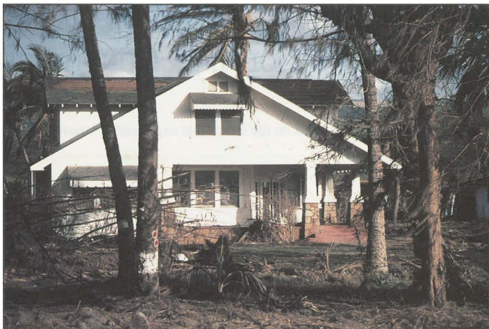
FIGURE 5. Flood damage to this coastal house in Kekaha was minimized because the house is elevated 2 to 3 feet off the ground and is located a considerable distance from the shoreline.
