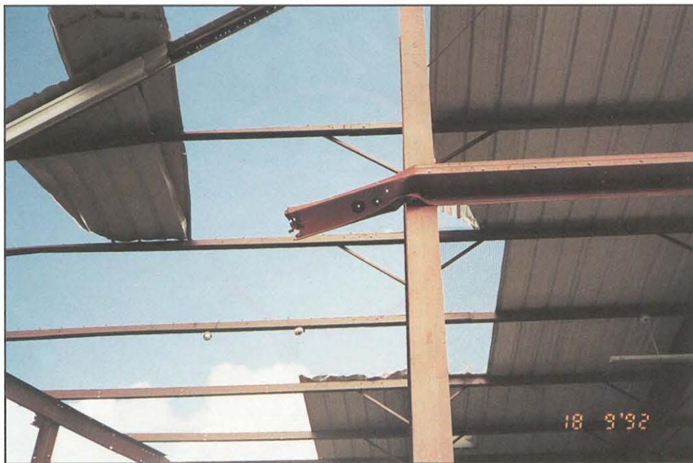
FIGURE 57. Steel warehouse failure was also due to failure of structural steel members.
