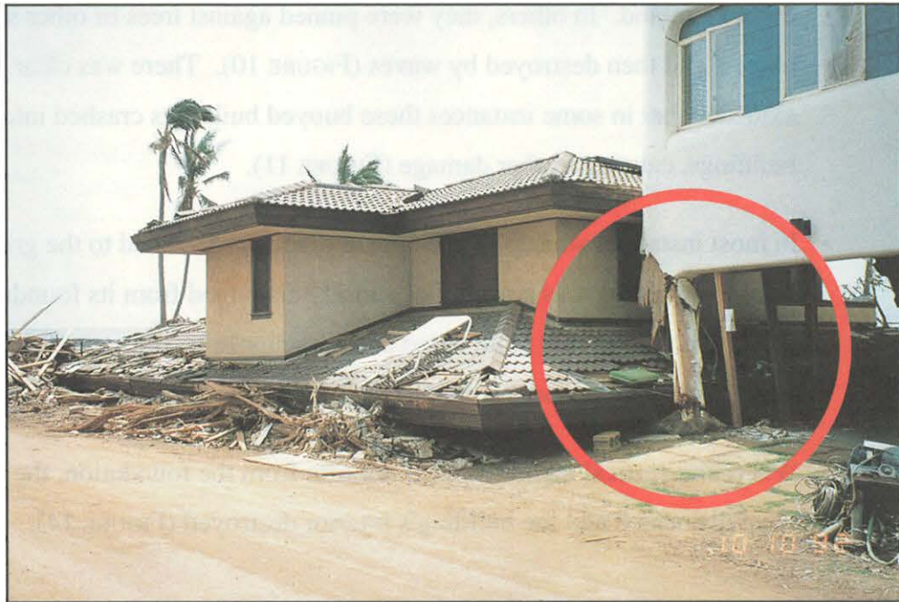
FIGURE 11. Non-elevated building at Poipu Beach that rammed and increased damage to an adjacent building.
