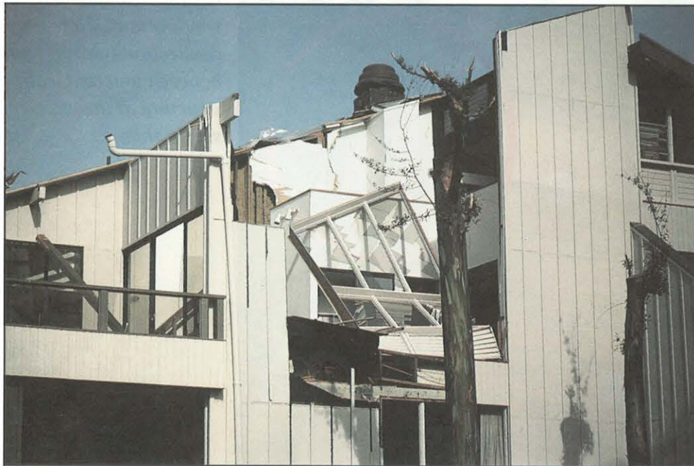
FIGURE 52. Gable-end window unit as a whole was displaced inward by wind pressure. Apparently, this allowed wind entry, increased interior pressure, and caused roof uplift.
