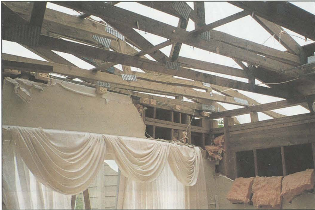
FIGURE 28. Individual prefabricated wood roof trusses performed relatively well.
