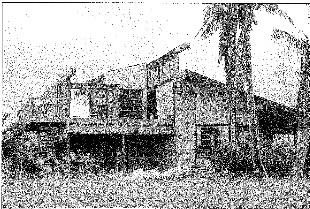
FIGURE 33. Offset roof peak provides geometric discontinuity and results in greater localized wind-induced pressure, which can lead to roof and then wall failure.
