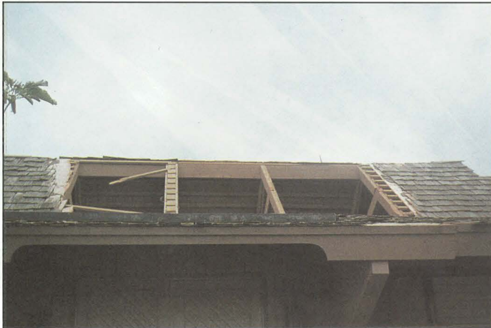
FIGURE 40. Loss of roof sheathing due to improper nailing design and schedule.
