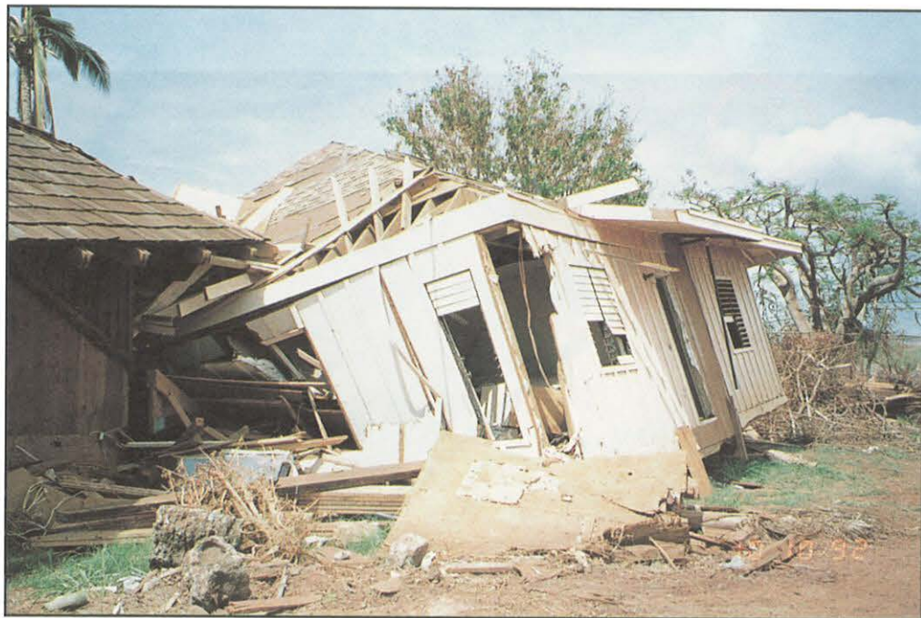
FIGURE 10. Non-elevated house at Poipu Beach that floated off its foundation was pinned against another house and destroyed by waves.
