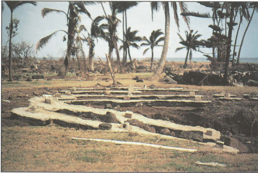
FIGURE 15. Foundation at Poipu Beach undermined by erosion.
