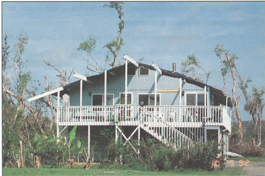
FIGURE 34. Excessive roof overhang and poor connections in many instances led to roof failure.
