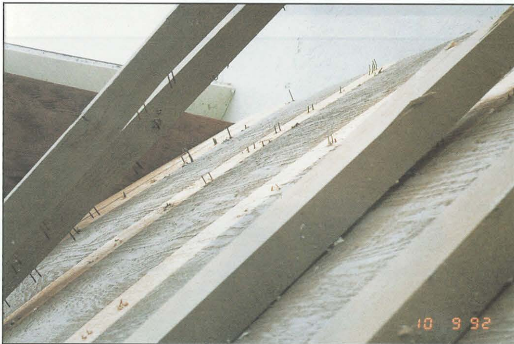
FIGURE 38. Improper attachment of sheathing to purlins. Note wide spacing, shallow penetration, misalignment, and corrosion of staples.
