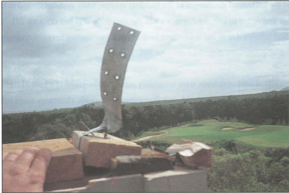
FIGURE 27. Undersized and improperly attached metal fasteners led to roof damage from uplift forces.
