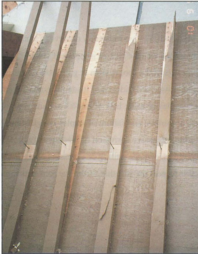
FIGURE 39. Improper nailing design and schedule for purlin-to-rafter attachment. Note infrequency of nails for large surface area. Nowhere is the plywood sheathing directly nailed to the rafter system.
