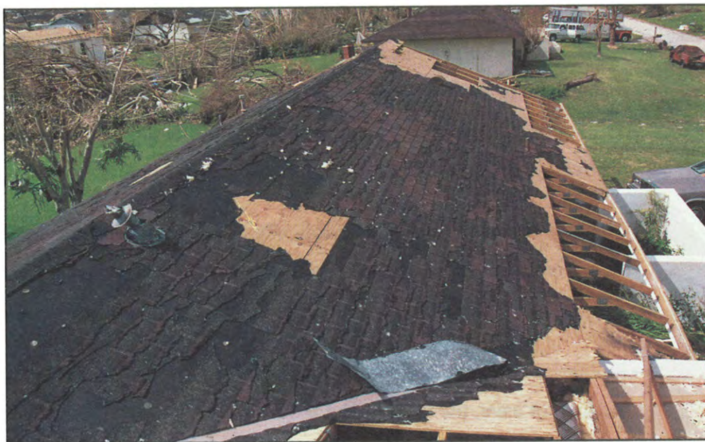
FIGURE 30. Composition shingle and underlayment failure.
