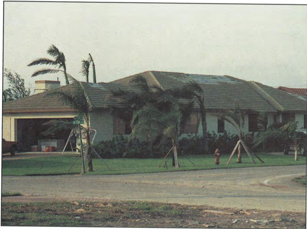
FIGURE 38. Hip roof.
