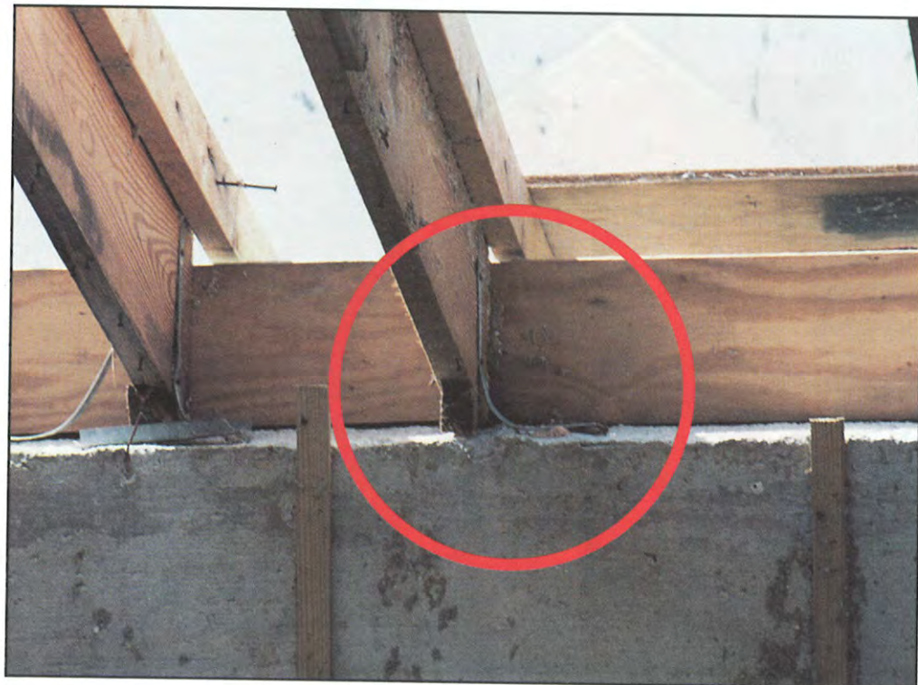
FIGURE 70. Improperly located masonry-wall-to-wood-frame straps.
