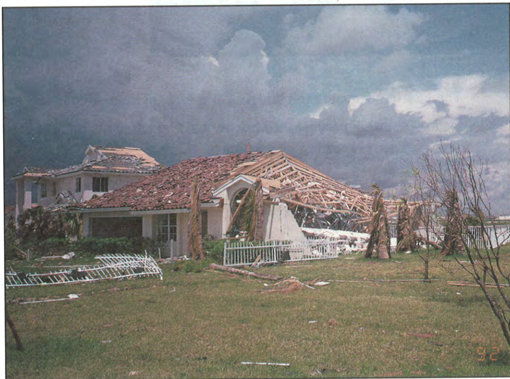
FIGURE 13. Roof structure failure due to inadequate bracing.
