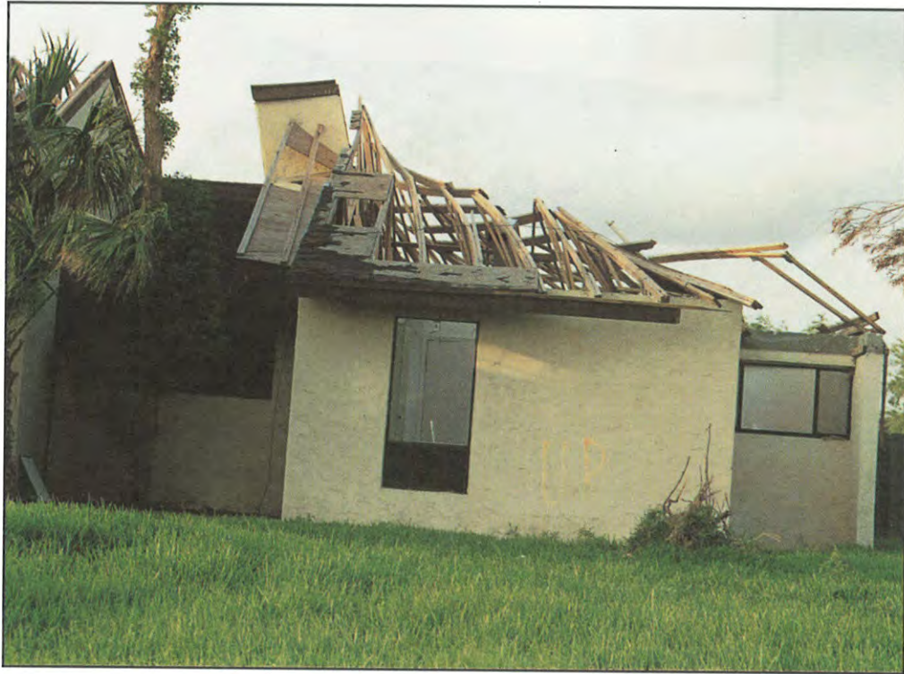
FIGURE 14. Roof structure failure due to inadequate bracing.
