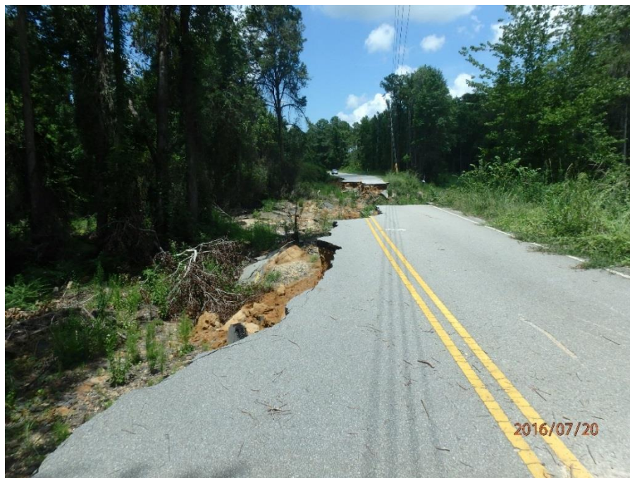
Figure 12: Head-Cutting of the Embankment at SCNONAME 14008 (Source: FEMA 2016)
