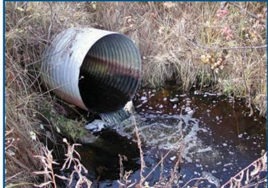
Figure 48 – A scour hole at an outlet resulting in erosion of the toe of the slope.
