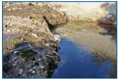
Figure 56 – Erosion of the spillway channel may lead to slumps or slides of the spillway sides, or large, uncontrolled, unintended releases in the event erosional headcutting in the spillway channel breaches the 55 spillway crest.
