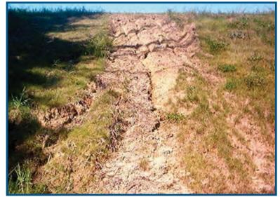
Figure 38 – Erosion on the downstream face of a dam.
