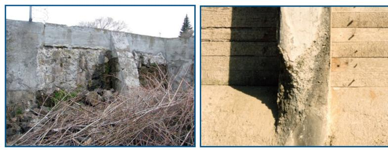
Figure 51 – Concrete deterioration on the downstream face of a dam.
