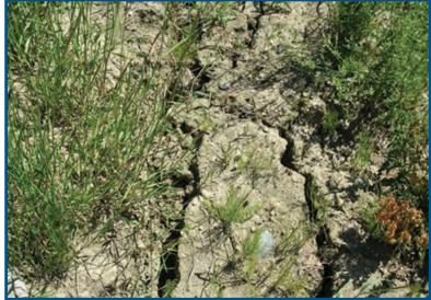
Figure 30 – Transverse cracks may provide open seepage paths through an embankment dam. 29
