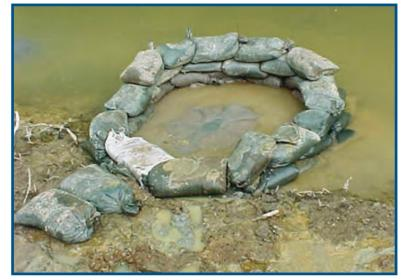
Figure 22 – Sandbags surrounding a boil on the downstream side of the dam (note the mound of material forming in the center of the sand-21 bagged area.
