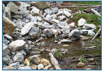
Figure 18 – Excessive seepage water exiting at the toe of the embankment.
