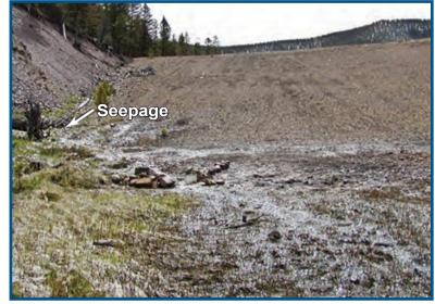
Figure 24 – Seepage at the abutment contact (groin) can lead to dam failure.
