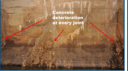
Figure 49 – Concrete deterioration, leakage and staining.
