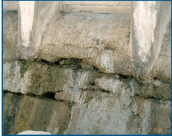
Figure 50 – Open joints.
