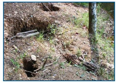
Figure 34 – Rodent holes in the dam face can cause seepage issues that could lead to dam failure.
