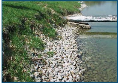
Figure 40 – Wave erosion on the unprotected face of a dam.
