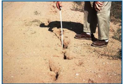
Figure 32 – Longitudinal cracks can be an indication of dam instability.
