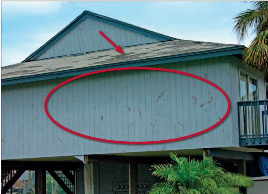
**Figure 11-2.** Numerous wind-borne debris scars on the wall of this house and several missing asphalt shingles. Estimated wind speed: 140 to 150 mph. Hurricane Charley (Florida, 2004)
