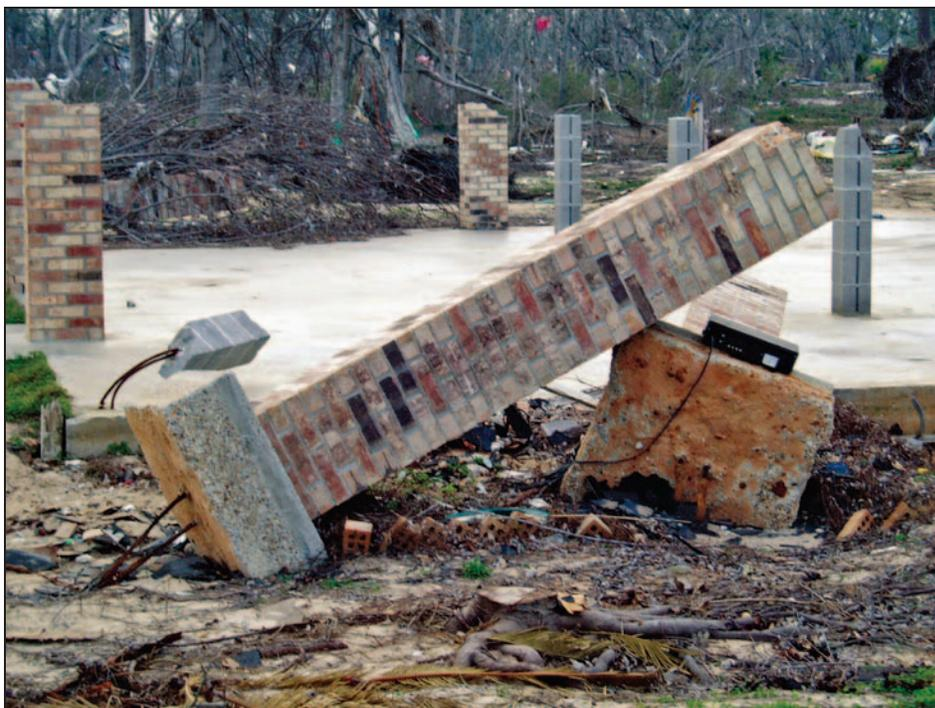
Figure 10-17. Performance comparison of pier foundations: piers on discrete footings (foreground) failed by rotating and overturning while piers on more substantial footings (in this case a concrete mat) survived Hurricane Katrina (Pass Christian, MS, 2005)
