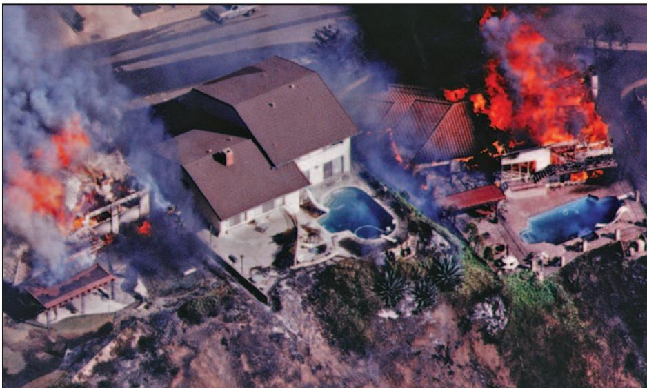
**Figure 11-3.** House that survived a wildfire due in part to fire-resistant walls and roof while surrounding houses were destroyed
