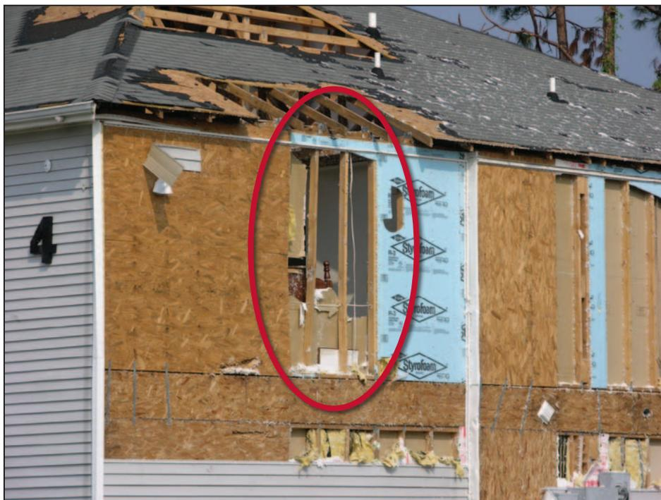
**Figure 11-15.** Blown-off vinyl siding and foam sheathing; some blow-off of interior gypsum board (circle). Estimated wind speed: 130 mph. Hurricane Katrina (Mississippi, 2006)
