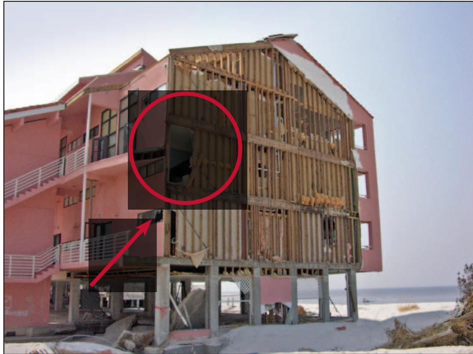
Several of the studs shown in Figure 11-19 were severely rotted, indicating long-term moisture intrusion behind the MEPS insulation. The residence shown in Figure 11-19 had a barrier EIFS design, rather than the newer drainable EIFS design (for another example of a barrier EIFS design, see Figure 11-21). EIFS should be designed with a drainage system that allows for dissipation of water leaks.
