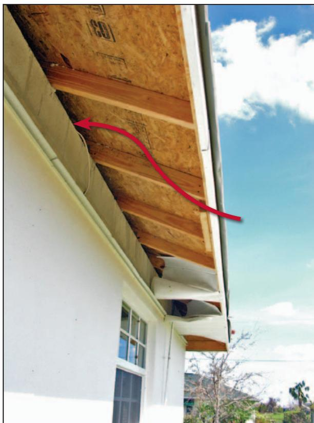
Figure 11-22. Blown-away soffit (arrow), which allowed wind-driven rain to enter the attic. Estimated wind speed: 140 to 160 mph. Hurricane Charley (Florida, 2004)
