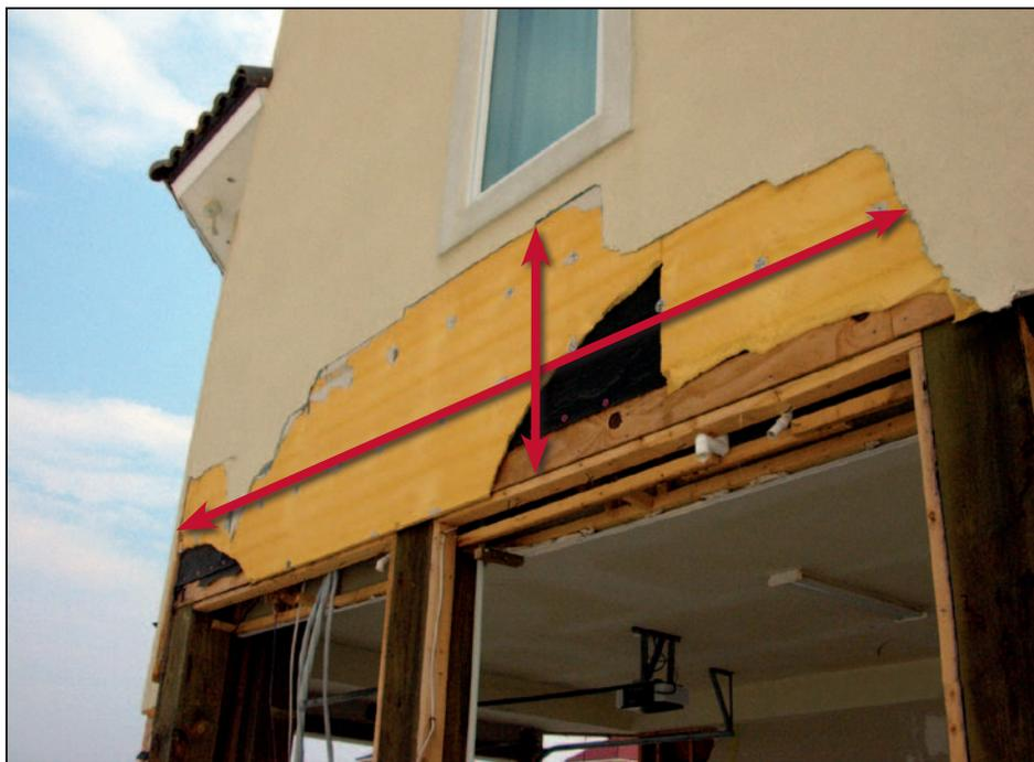
**Figure 11-20.** Collapse of the breakaway wall, resulting in EIFS peeling. A suitable transition detail at the top of breakaway walls avoids the type of peeling damage shown by the arrows. Estimated wind speed: 105 to 115 mph. Hurricane Ivan (Alabama, 2004)
