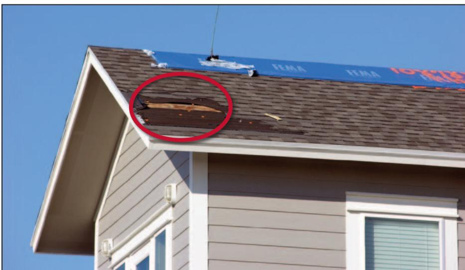
Figure 11-31. Loss of shingles and underlayment along the rake. Estimated wind speed: 110 mph. Hurricane Ike (Texas, 2008)
