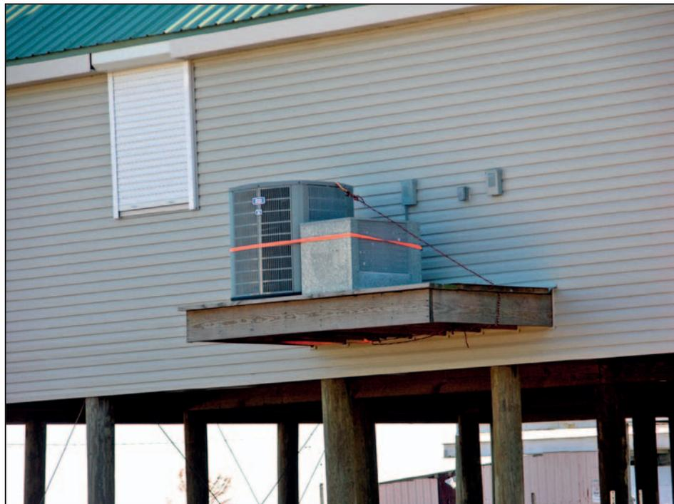
systems. Mechanical equipment can also be damaged or destroyed when inundated by floodwaters, especially saltwater. Although a short period of inundation may not destroy some types of mechanical equipment, any inundation of electric equipment causes, at a minimum, significant damage to wiring and other elements.
