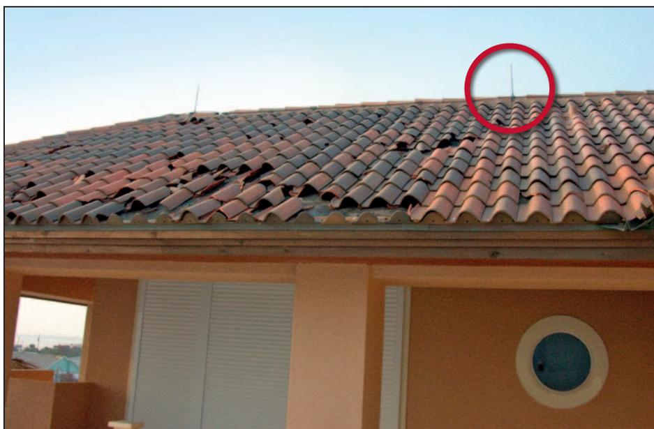
Figure 11-48. The fastener heads on this mechanically attached tile roof had corroded; air terminals (lightning rods) in a lightning protection system (circle). Hurricane Ivan (Alabama, 2004)
