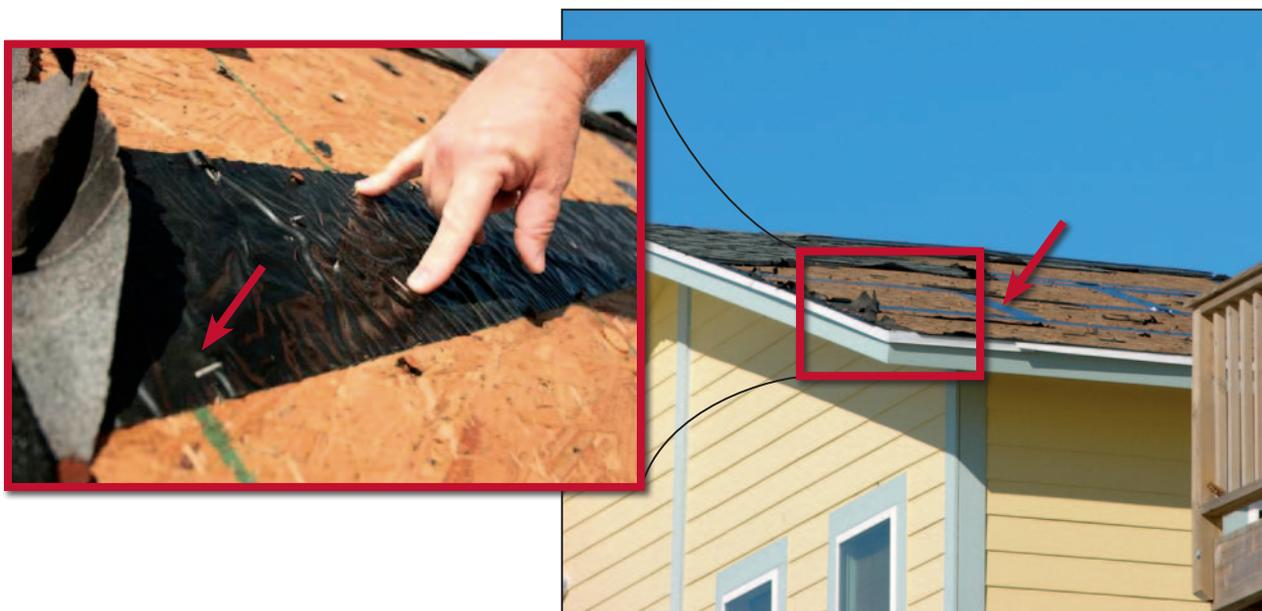
**Figure 11-28.** House that used enhanced underlayment Option 3 with taped sheathing joints (arrow). The self-adhering modified bitumen tape (inset) was stapled because of bonding problems. Estimated wind speed: 110 mph. Hurricane Ike (Texas, 2008)
