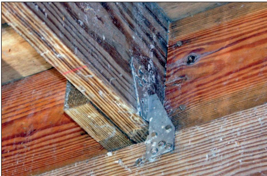
**Figure 9-17.** Metal joist-to-beam connector
