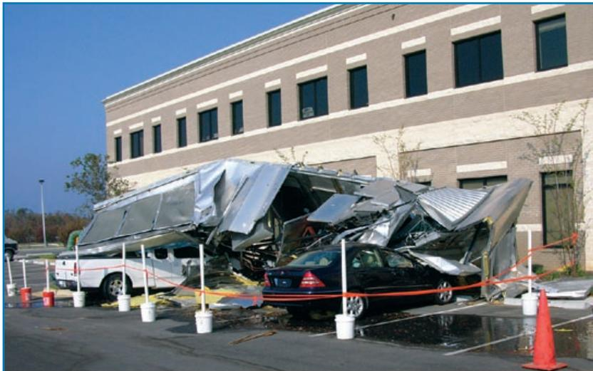
Figure 3-69: Although this 18,000-pound HVAC unit was attached to its curb with 16 straps, it blew off during Hurricane Ivan. (Florida, 2004)
