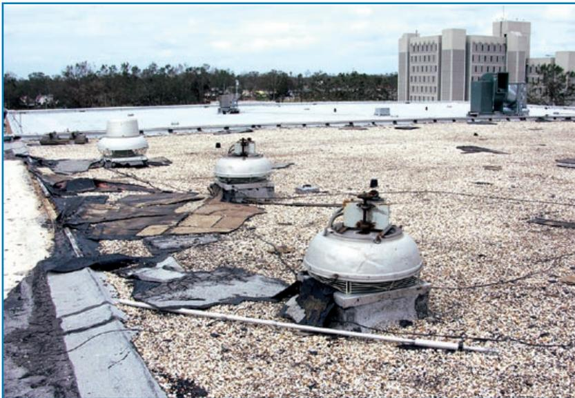
Figure 3-70: Cowlings blew off two of the fans on a police building that housed the county's EOC. Hurricane Ivan (Florida, 2004)
