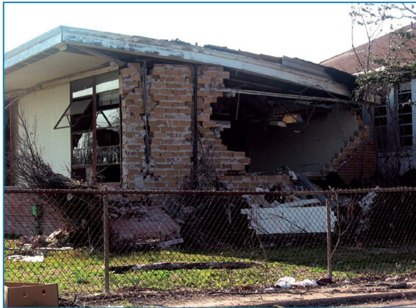
Designing the connections between structural components according to loads is critical to maintaining the load path and the structural integrity of school buildings in hurricane-prone regions.
