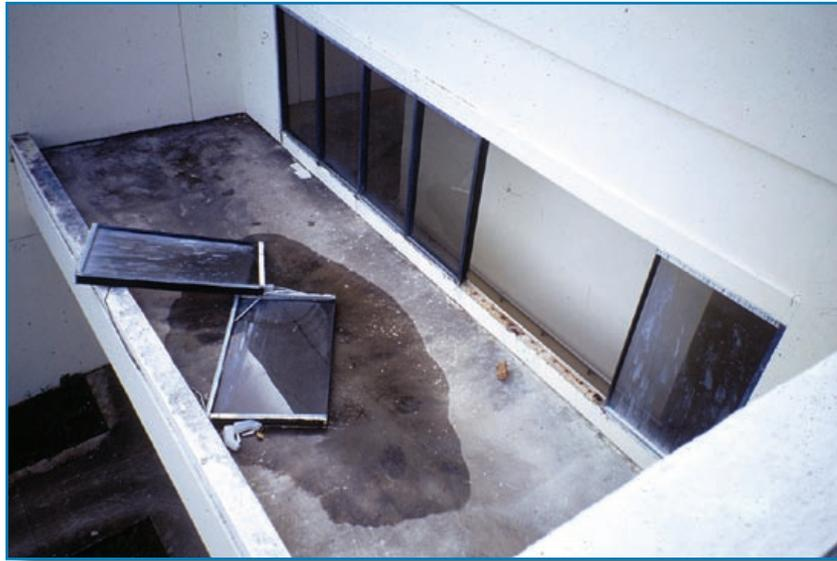
The successful integration of windows and curtain walls into exterior walls is a challenge in protecting against water infiltration. To the extent possible when detailing the interface between the wall and the window or curtain wall units, designers should
