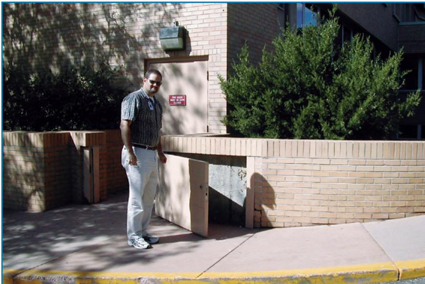
Figure 2-33: Boulder Community Hospital, Boulder, CO installed this permanently mounted floodgate in a low floodwall; the floodgate swings to the left to close off the door that leads to the mechanical equipment room.
