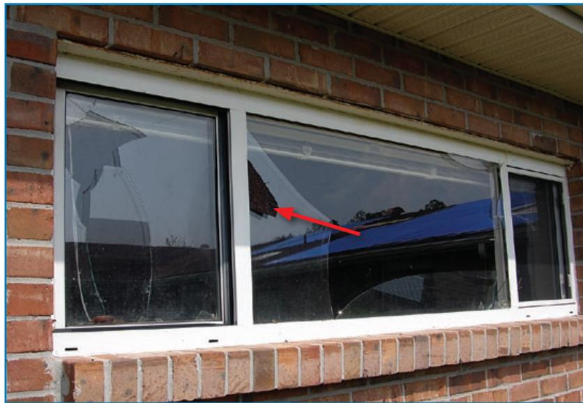
In order to minimize interior damage, the IBC, through ASCE 7, prescribes that exterior glazing in wind-borne debris regions be impact-resistant, or be protected with an impact-resistant covering (shutters). For Category III and IV buildings in areas with a basic wind speed of 130 mph or greater, the glazing is required to resist a larger momentum test missile than would Category II buildings and Category III and IV buildings in areas with wind speeds of less than 130 mph.
