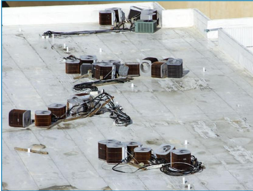
Figure 3-73: Sleeper-mounted condensers displaced by high winds. Hurricane Katrina (Mississippi, 2005)
