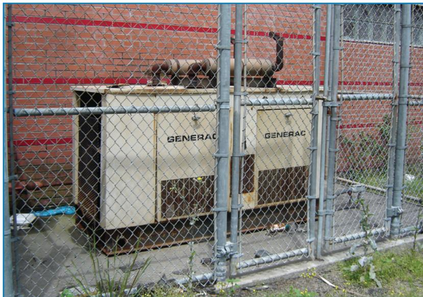
The need to provide a back-up generator at a safe and elevated location is confirmed by the experiences during Hurricane Katrina. Many facilities were without power because of the low elevation and subsequent flooding of their generators. Jackson County EOC had its emergency power station elevated and protected in a separate enclosure, which allowed the facility to operate without interruption (see Figure 4-48).
