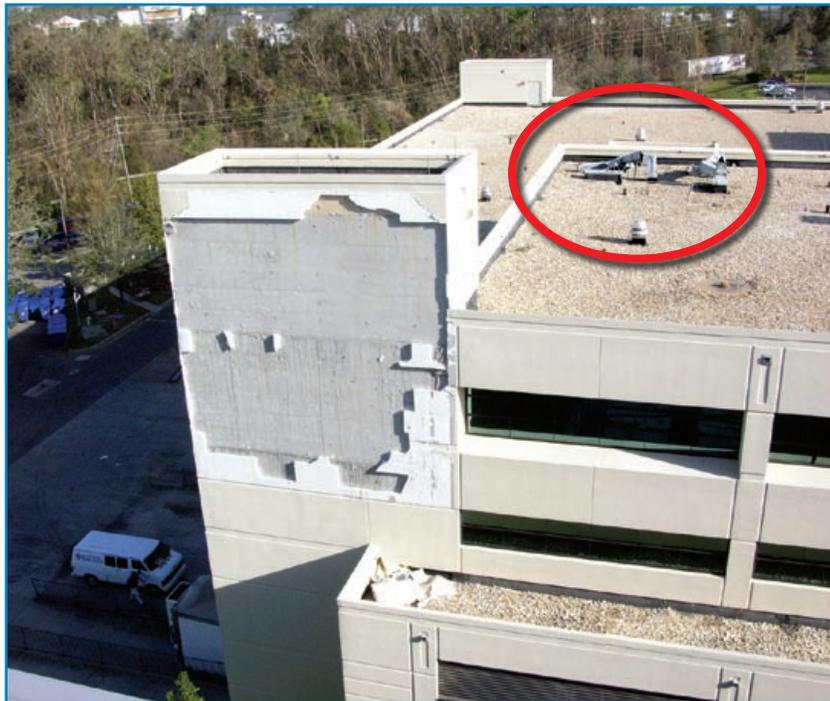
Wind-borne EIFS debris can be devastating to unprotected glazing. At the hospital shown in Figure 3-56, the hospital's original concrete wall panels had been furred with metal hat channels and covered with EIFS. In a large corner area, the EIFS and gypsum board substrate blew off the hat channels and broke a large number of windows in the multi-story connecting walkway
