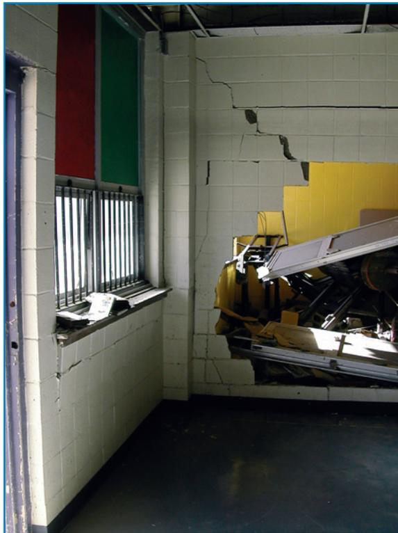
**Buoyancy and uplift:** If below-grade areas are essentially watertight, buoyancy or uplift forces can float a building out of the ground or rupture concrete floors (see Figure 2-15). Buildings that are not adequately anchored can be floated or pushed off foundations. Although rare for large and heavy critical facility buildings, this is a concern for outbuildings and portable (temporary) units.
