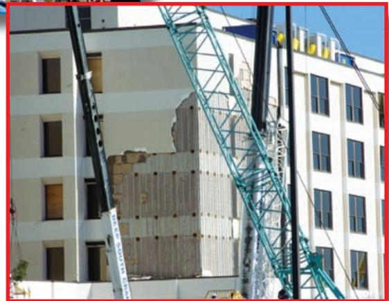
Another issue associated with EIFS is the potential for judgment errors. EIFS applied over studs is sometimes mistaken for a concrete wall, which may lead people to seek shelter behind it. However, instead of being protected by several inches of concrete, only two layers of gypsum board (i.e., one layer on each side of the studs)
