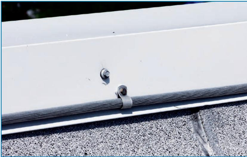
Figure 3-97: This conductor was attached to the coping with a looped connector. Hurricane Katrina (Mississippi, 2005)
