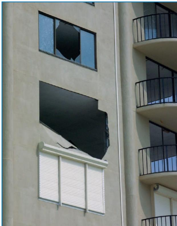
Deploying accordion or panel shutters a few stories above grade is expensive. Although motorized shutters have greater initial cost, their operational cost should be lower. Other options for providing missile protection on upper levels include replacing the existing as-
