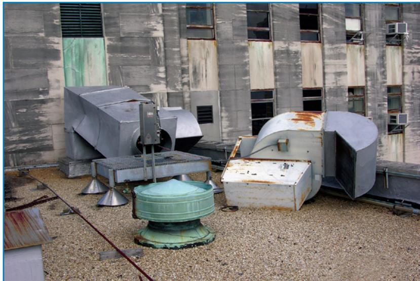
Air-conditioning systems were also disrupted by a lack of water needed for water-cooled chillers, as happened in Garden Park Medical Center in Gulfport when the municipal water service was shut down. Loss of air-conditioning resulted in interior condensation, and warm and humid air interfered with the normal functioning of electronic medical equipment.
