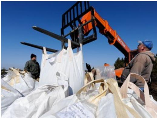
Dam owners should identify borrow sources for sand, gravel, and riprap material or have them stockpiled at the dam site. In some cases, dam owners may want to stockpile sandbags in advance of a storm event. These
