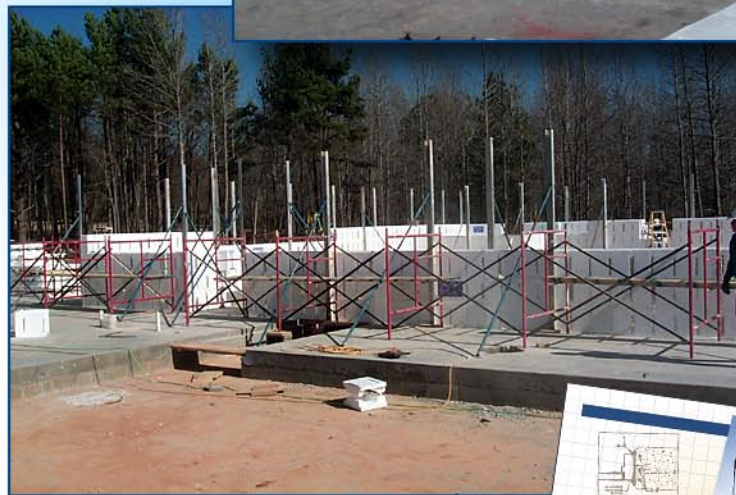
Erection of the reinforced ICF walls.
