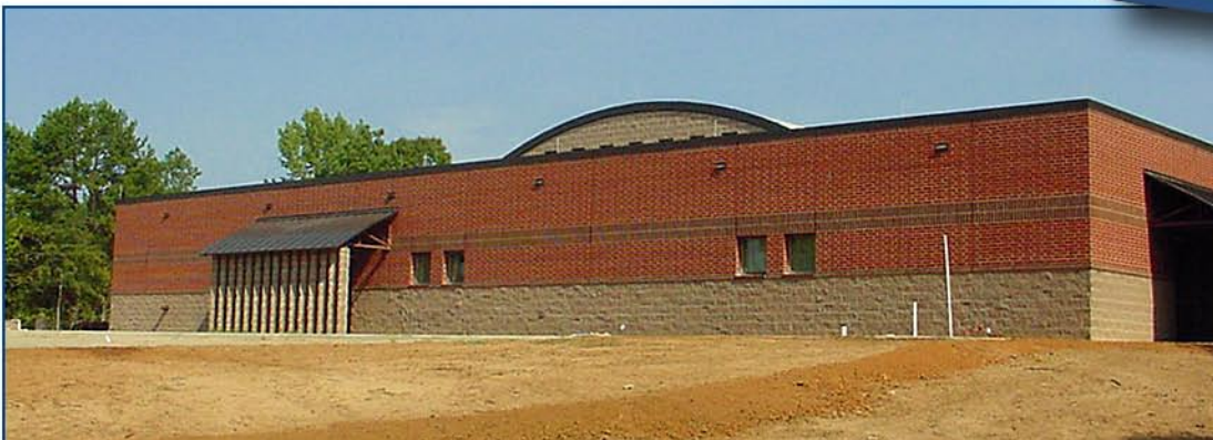
Completed reinforced ICF walls.
