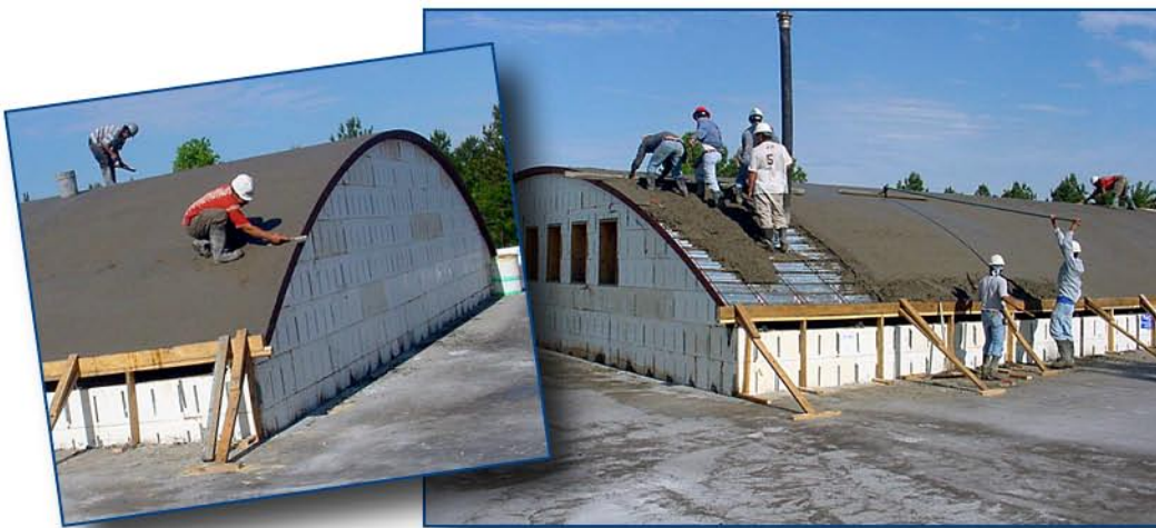
Construction of the steel-truss roof system.
