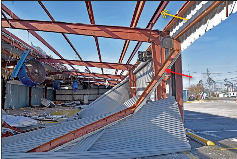
Figure 8: View of the new purlin
