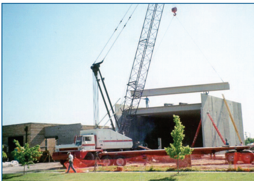
Community safe room being constructed to FEMA 361 criteria in Wichita, KS.
