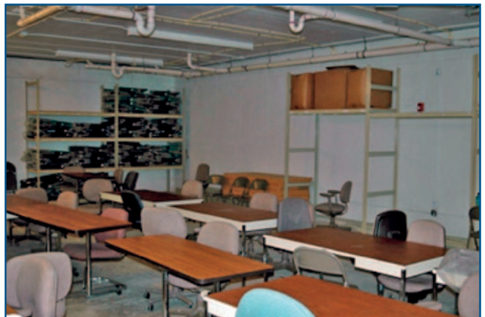
HMGP-funded community safe room constructed in the basement of a new fire station in Brookside, AL.
