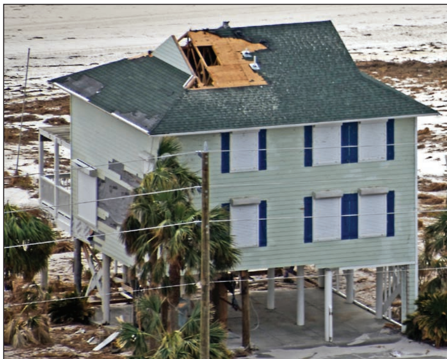
Figure 13: Residence where retrofitted shutters performed well, but significant damage was sustained when rain entered at blown-off roof deck panels (Port St. Joe, FL)
