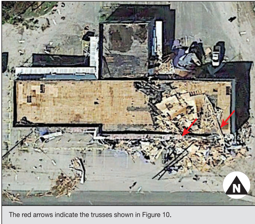
Figure 11: Aerial view of the police station
