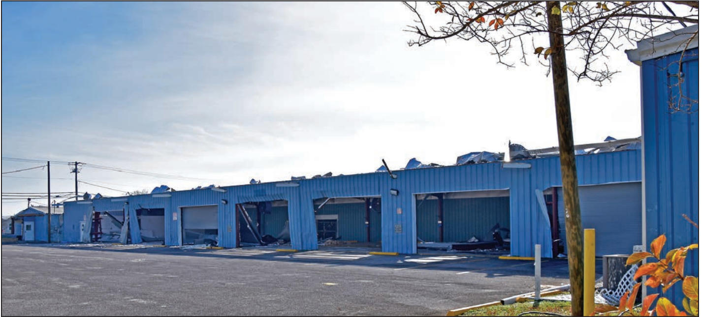
Figure 6: General view of the damaged retrofitted rolling doors and roof panel damage
