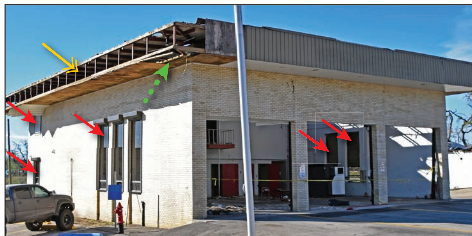
The red arrows indicate the retrofitted storm shutters. Wind-driven rain entered the building at the damaged fascia and soffit (yellow and green arrows).
