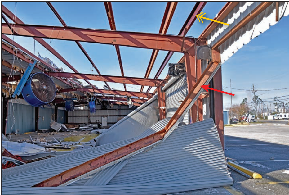
Figure 8: View of the new purlin
