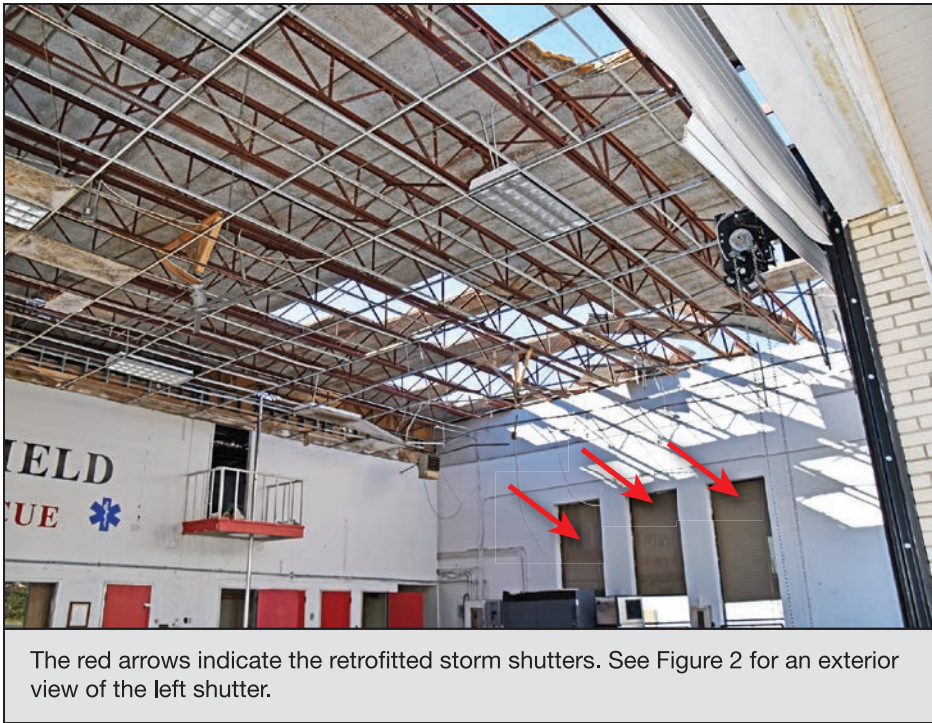
Figure 5: View of damaged roof after roof deck panels were blown off
