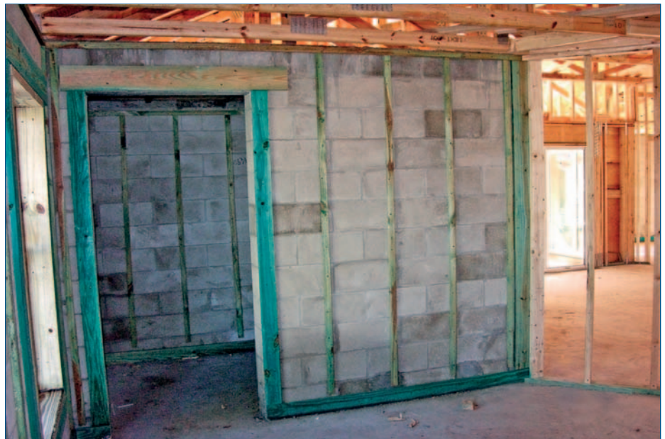
View of an in-residence safe room under construction. Steel reinforced and fully grouted CMU surround the safe room space (New Smyrna Beach, FL).
