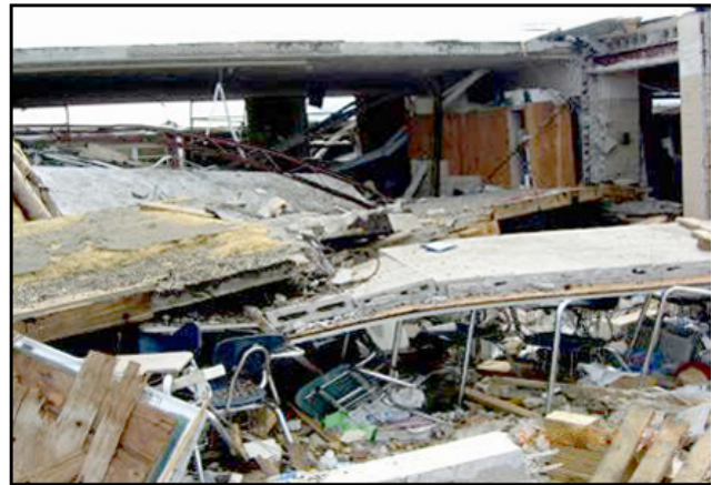
Figure 2. Destroyed tornado refuge area at Enterprise High School, Enterprise, Alabama (2007)
