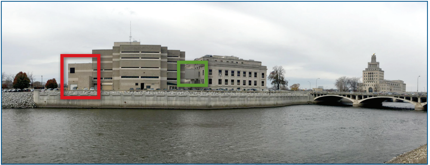
Figure 5: Linn County Correctional Center and Court House located in Cedar Rapids, Iowa. The 2008 flood waters crested over the bridge to the right of the picture inundating the basements, tunnels, and ground floors, where mechanical equipment was located. The red rectangle indicates the 5 story addition that was constructed to hold the critical equipment and gear to maintain operations during and after a flood. The green rectangle shows the new bridge created to move people between the buildings now that the tunnel system is closed.
