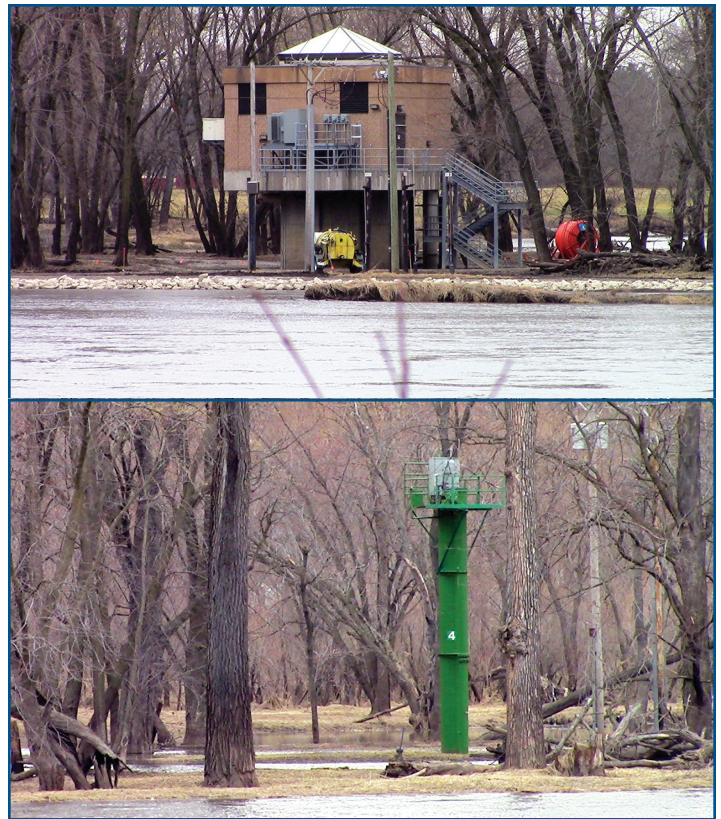
Figure 1: Cedar Rapids wells submerged and critically damaged in the 2008 floods have been raised 10ft. The upper image is a collector well and the lower image is a single point well.
