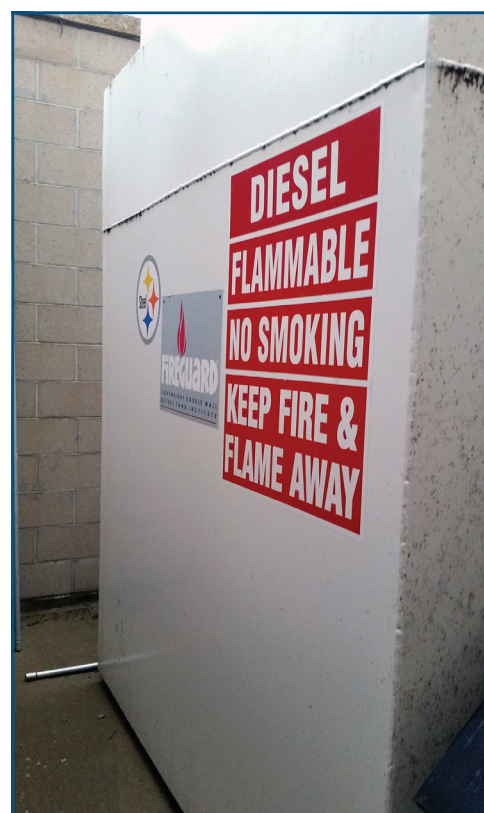
Figure 3: Above ground fuel tank located outside adjacent to a facility in Linn County, Iowa.
