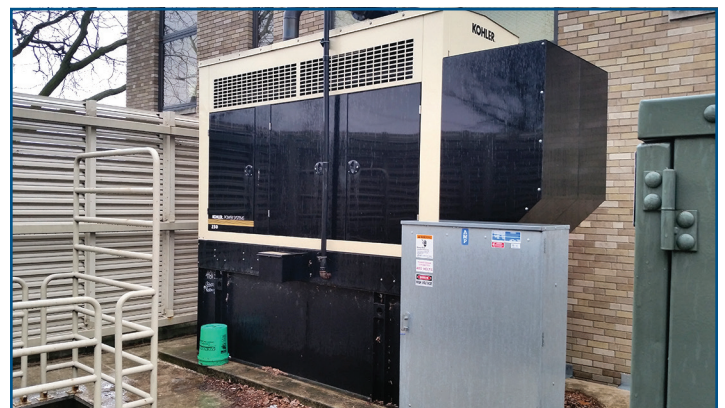
Figure 2: This generator and fuel tank, serving the Linn County Sherriff's office in Cedar Rapids, Iowa, was raised approximately 10 feet above the 500-year flood elevation and above the flood of record in response to the 2008 floods.
