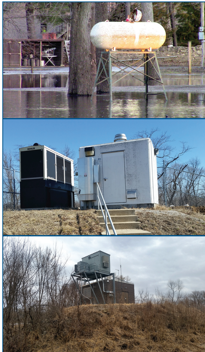
Figure 1: Propane fuel tank for a residence elevated above the flood waters near Cedar Falls, Iowa (top); Elevated generator and fuel tank for a lift station serving Palo, Iowa (middle); Elevated Emergency Power system for a collector well in Cedar Rapids, Iowa (bottom).
