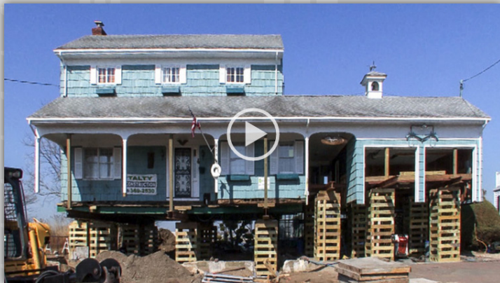
After being flooded by Hurricane Sandy, Long Island homeowner Al Grover decided to raise his home 13 feet in order to mitigate future flood damage.
