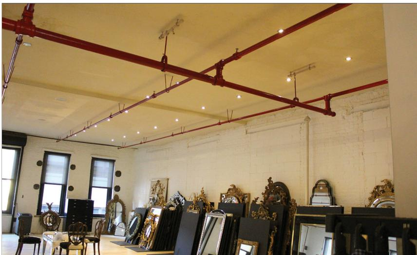
Figure 5-20. Fire protection piping and sprinkler heads installed along the building ceiling.
