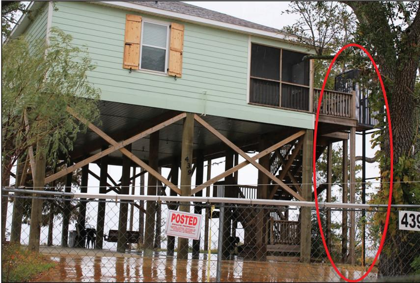
Figure 4-37. Residential coastal building with passenger lift circled in red.
