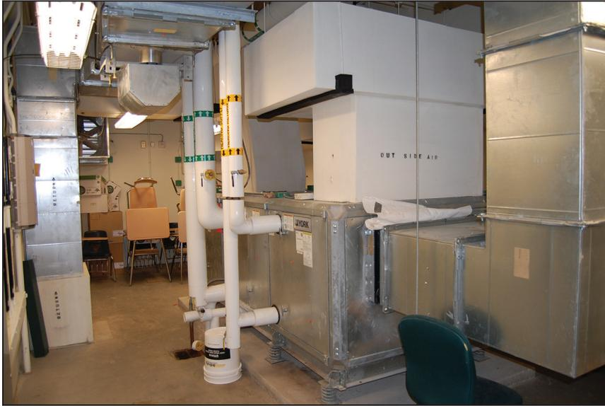
Figure 5-6. AHU with a separate chilled water coil (green labels) and hot water coil (yellow labels). The coils are within the unit and are not visible (Dagsboro, Delaware).
