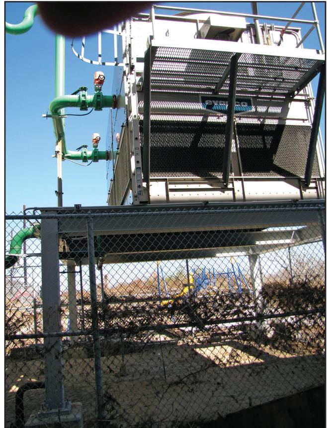
**Figure 5-7. Cooling tower placed on an elevated frame (Hurricane Ike, Port Bolivar, Texas, October 18, 2008).**
