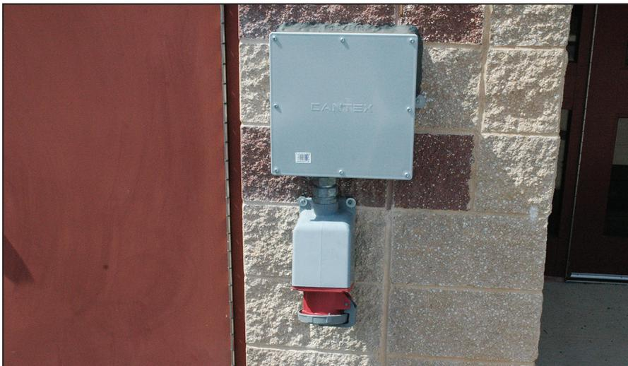
**Figure 4-14.** Flanged connection (quick connect) for connecting temporary generator (Milford, DE).
