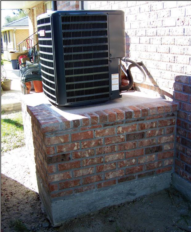
Figure 3-1. Air conditioning compressor elevated on a pedestal.
