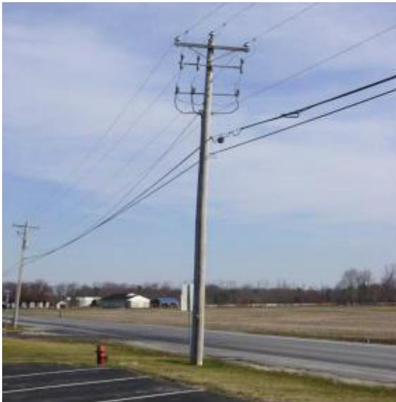
Figure 2-4 Riser pole of an underground electrical line supplied from an overhead line.
