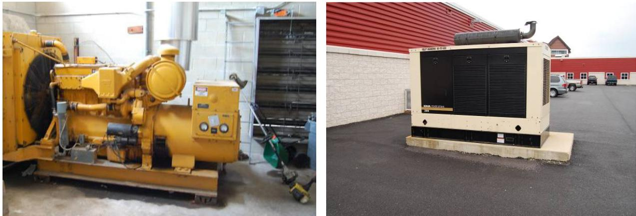
Figure 5-3 Emergency generator installed on the interior (left) and exterior (right).
