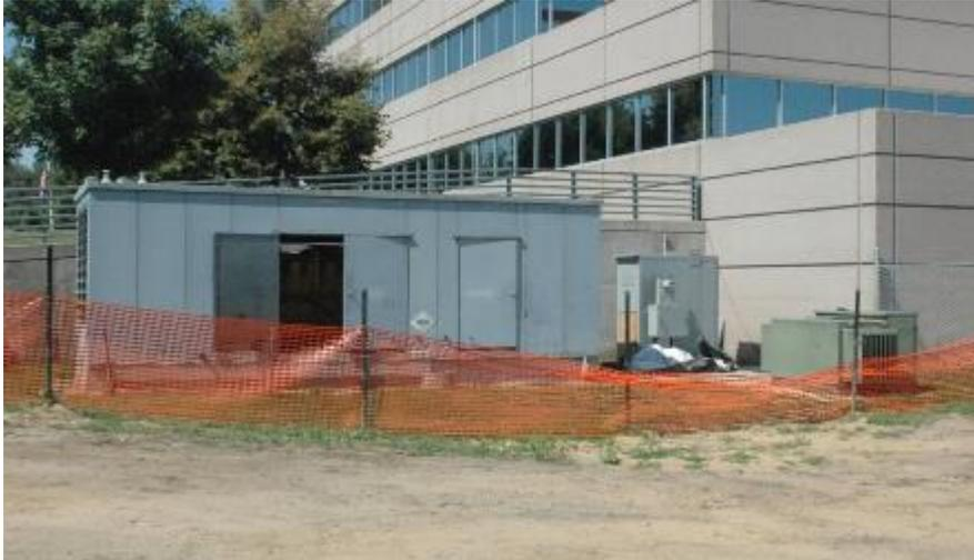
Figure 2-11 Emergency generator in an exterior enclosure in Cedar Rapid, Iowa, inundated during the 2010 Midwest floods.
