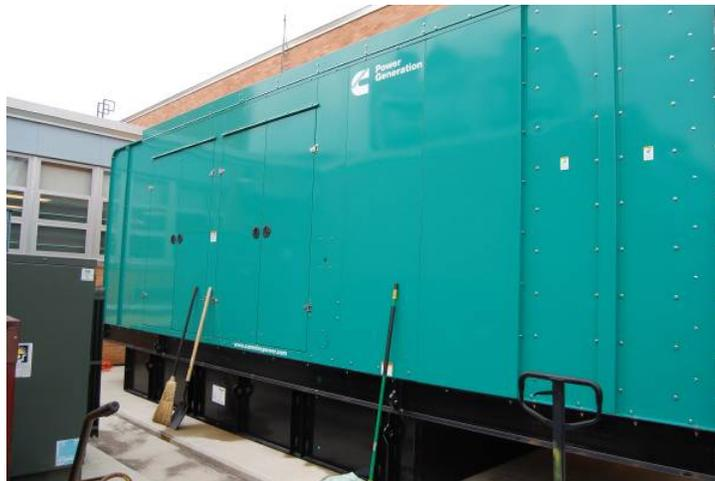
Figure 5-4 Exterior emergency generator placed in a sound-attenuating enclosure.
