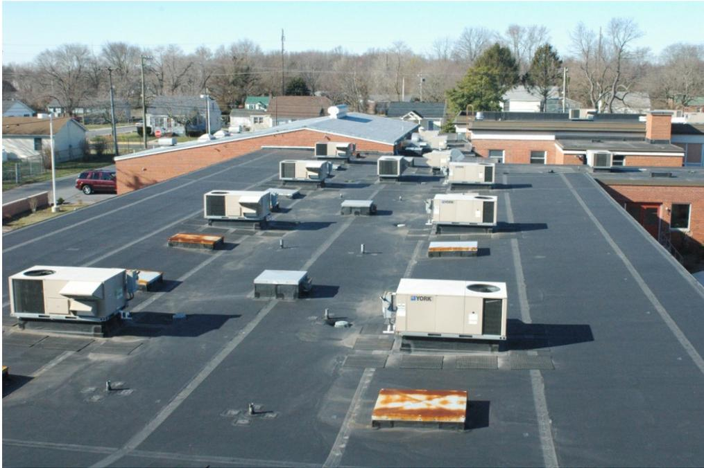
Figure 4-4 Roof-top mounted DX HVAC units.
