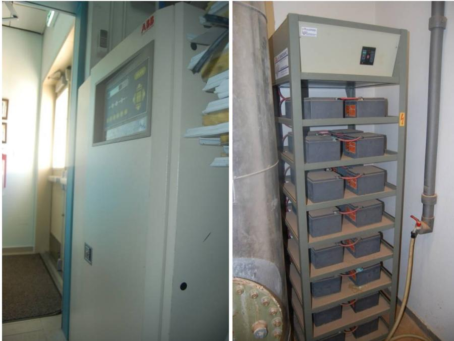
Figure 5-1 UPS system containing an inverter (left) and battery rack (right) located in a low seismic area.
