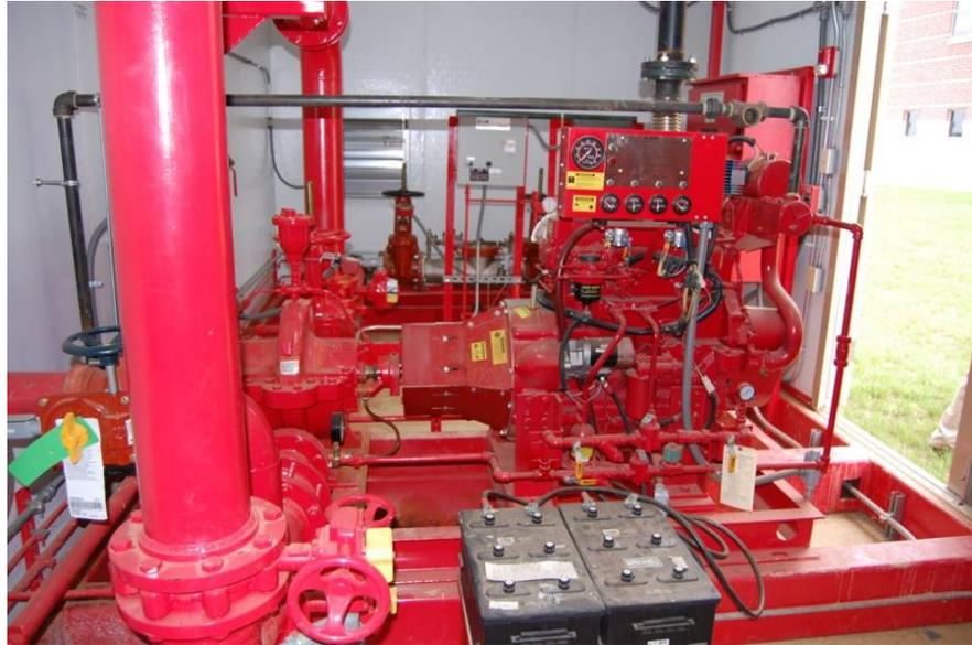
Figure 6-1 Diesel-driven fire pumps.
