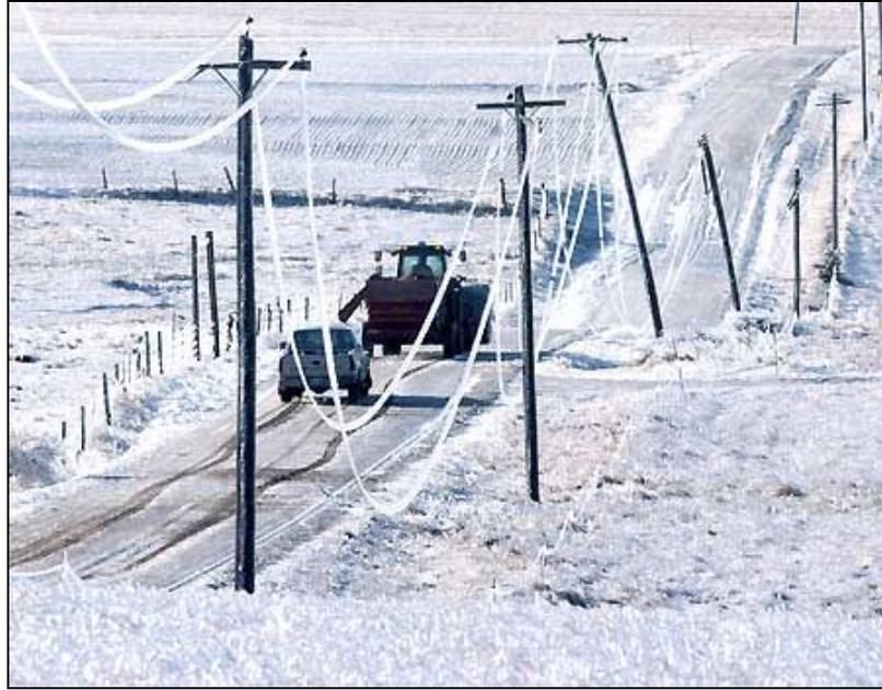
Figure 2-2 Damage to overhead distribution line caused by weight of ice accumulation (Nyether, 2014).
