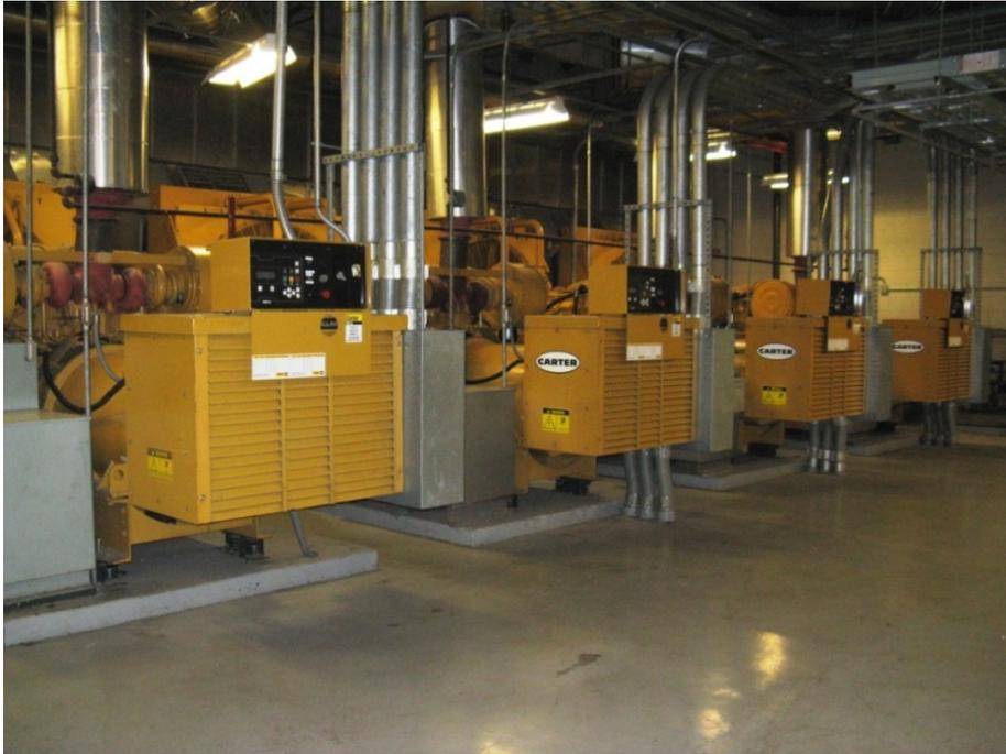
Figure 5-6 Multiple generators in parallel.
