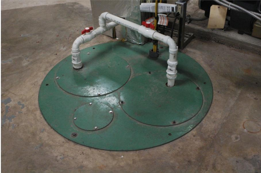
Figure 4-7 Sump cover; pump is within the sump.
