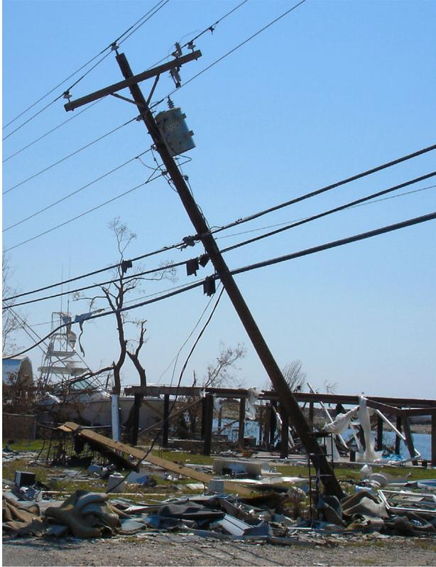
Figure 2-10 Overhead line damaged when flooding saturated soils and reduced strength of guy anchors (Deleon, 2014). Hydrodynamic loads from moving floodwaters may have contributed to failure.
