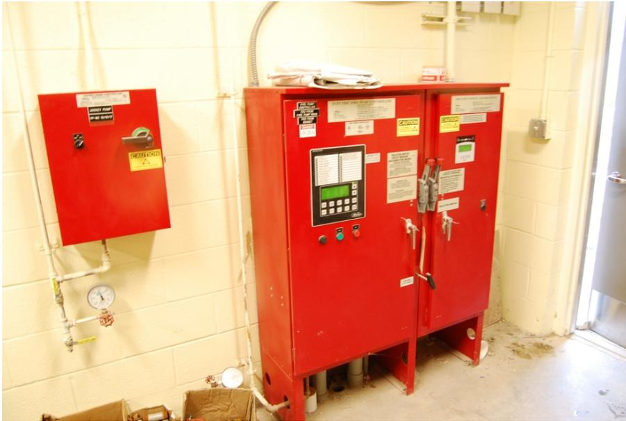
Figure 4-2 Typical fire pump controller.
