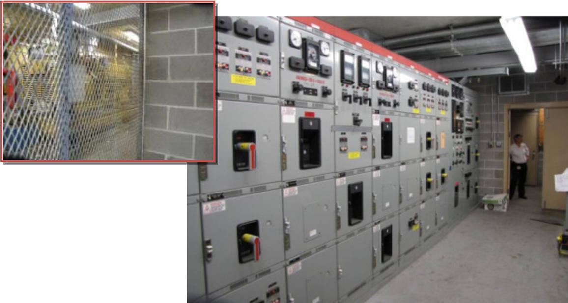
Figure 6-3 Switchgear, normal, and emergency power feeds, and associated equipment elevated to the same level as the emergency generator at UTMB, Galveston, Texas in 2010.
