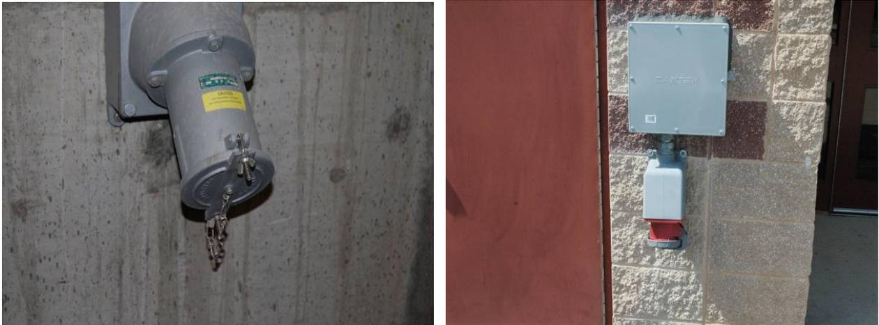
Figure 5-8 Building-mounted twist-lock plugs for connecting temporary generator cables.
