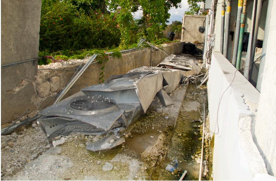
Figure 2-16 Falling debris from security wall and parapet damaged cooling equipment for servers resulting in the data center going off line in the 2011 Haiti earthquake.
