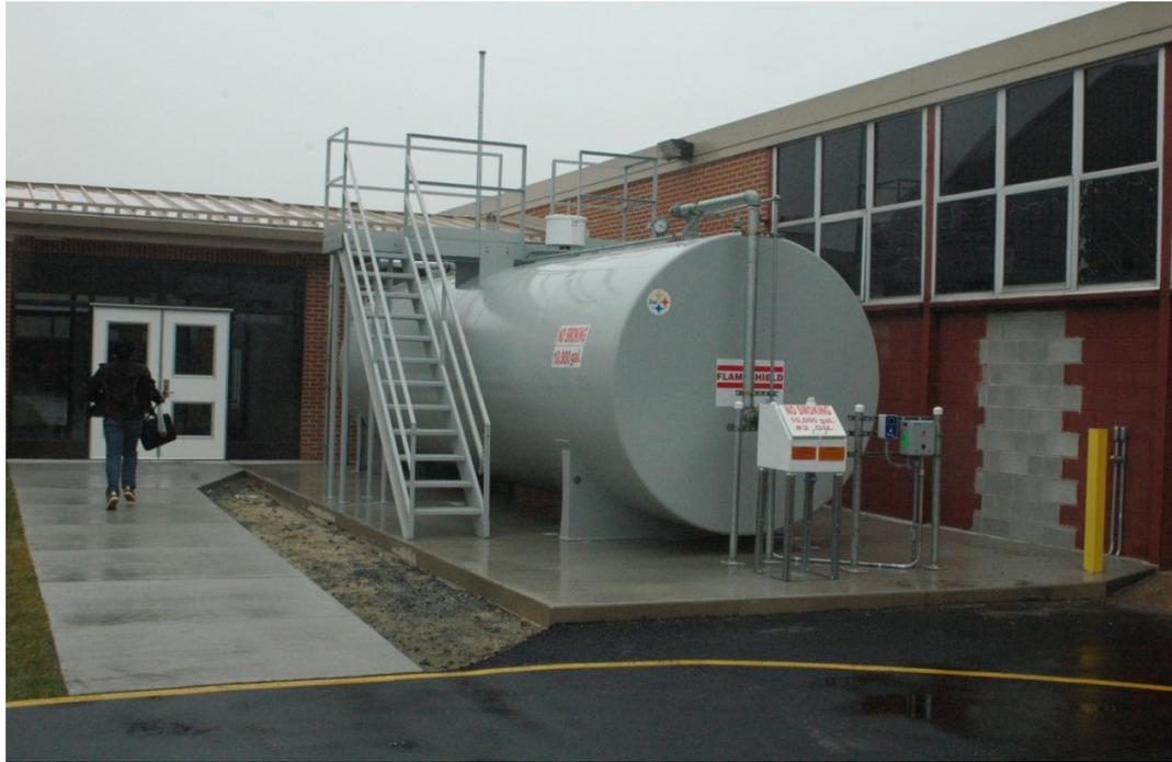
Figure 5-5 Fuel oil storage tank used for heating equipment that can supply an emergency diesel generator.
