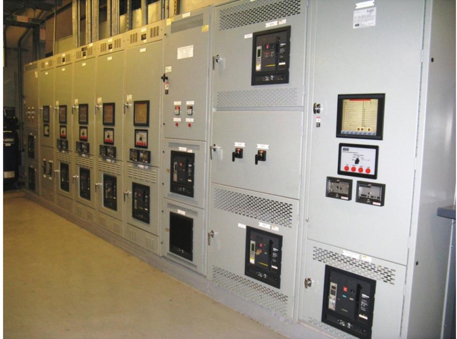
Figure 5-7 Generator synchronizing board.
