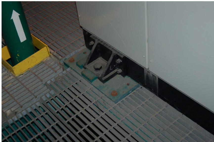
Figure 2-15 Well-anchored equipment (FEMA, 2012b).
