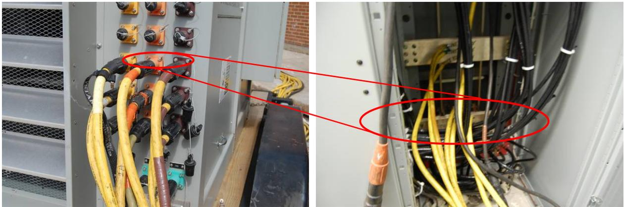
Figure 5-9 Electrical connection point for temporary generator using slip-fit connectors (left), and cables at building connection (right).
