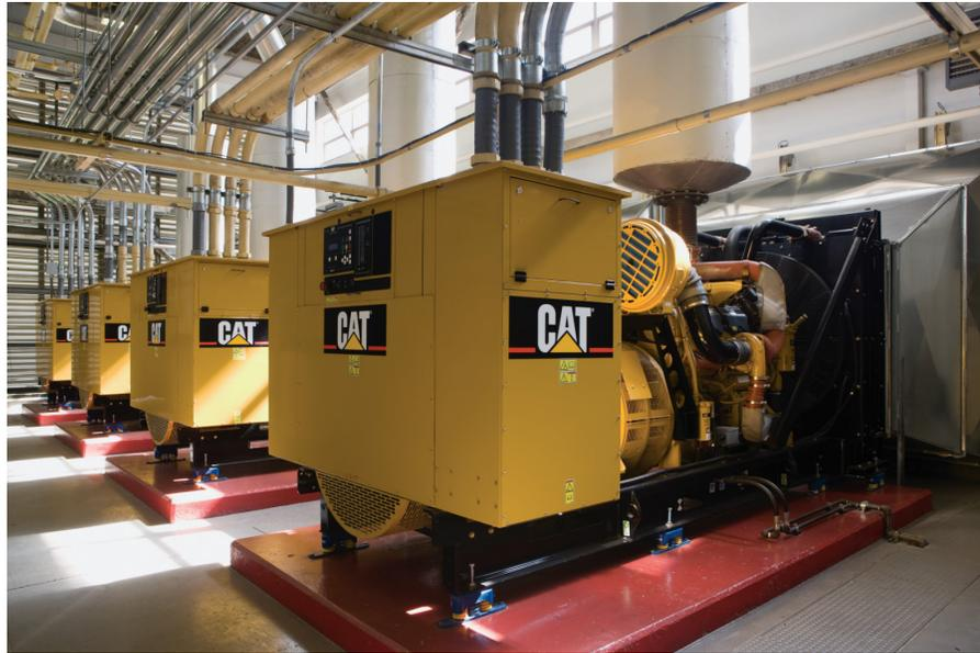
Figure 6-5 Emergency generator supported by seismically-rated vibration isolators.
