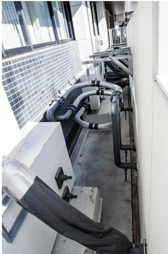
Figure 2-18 Typical flexible utility connections in base isolated building.
