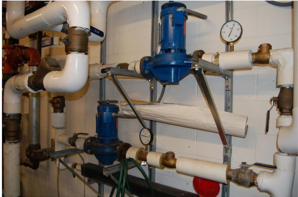
Figure 4-9 Domestic hot water circulator pumps.
