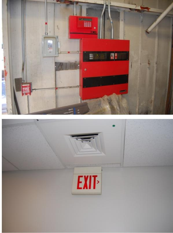
Figure 4-1 Life-safety equipment: fire alarm control panel (top) and exit signage (bottom).
