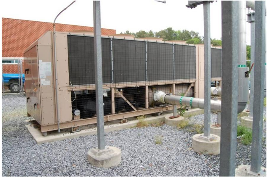
Figure 4-6 Air-cooled chiller.
