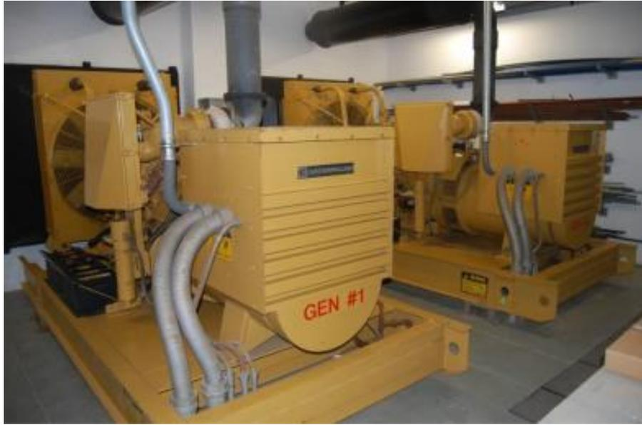
Figure 6-4 Interior generator protected from the effects of wind and wind-borne debris.
