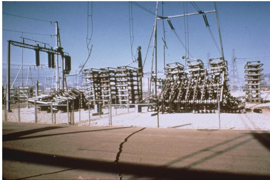
Figure 2-13 Sylmar high voltage direct current converter station damaged in the 1971 San Fernando earthquake (NOAA/NGDC, E.V. Leyendecker, U.S. Geological Survey).
