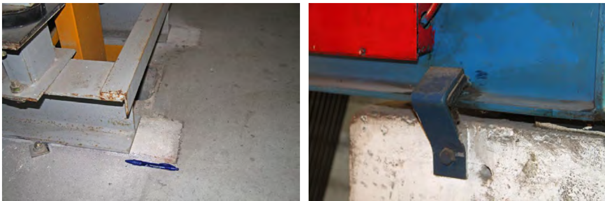
Figure 6.4.10.2-5 Details of bent bracket (left) and large displacement at the base of elevator machines (Photos courtesy of Eduardo Miranda, Stanford University).
