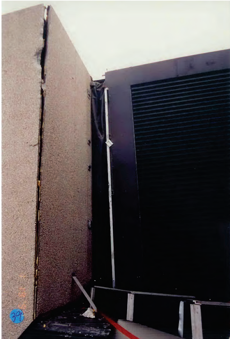
Figure 6.3.1.3-3 Precast panel damage at a building corner in the 1994 Northridge Earthquake (Photo courtesy of OSHPD).
