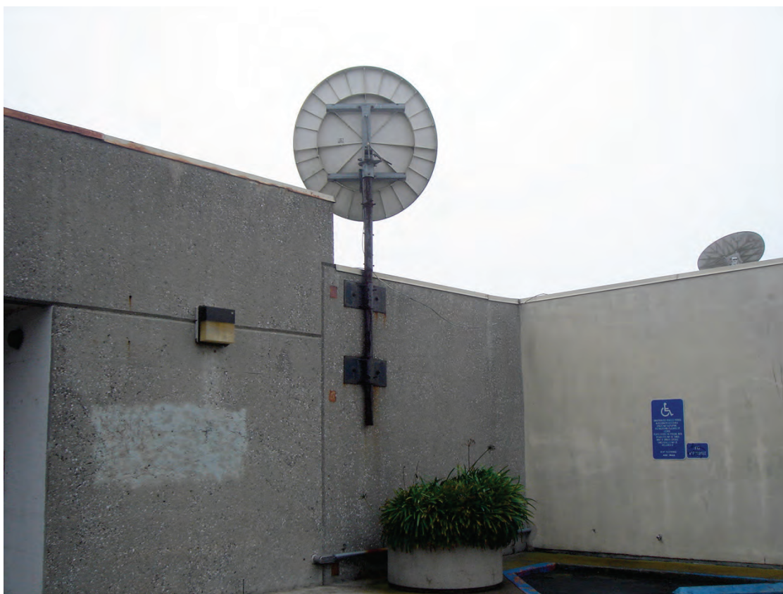
Figure 6.4.7.6-5 Antenna mast mounted to concrete wall surface at top floor of building (Photo courtesy of Maryann Phipps, Estructure). Note that two wall brackets are used to resist moments produced by wind or seismic forces. This antenna is larger than most standard residential versions.
