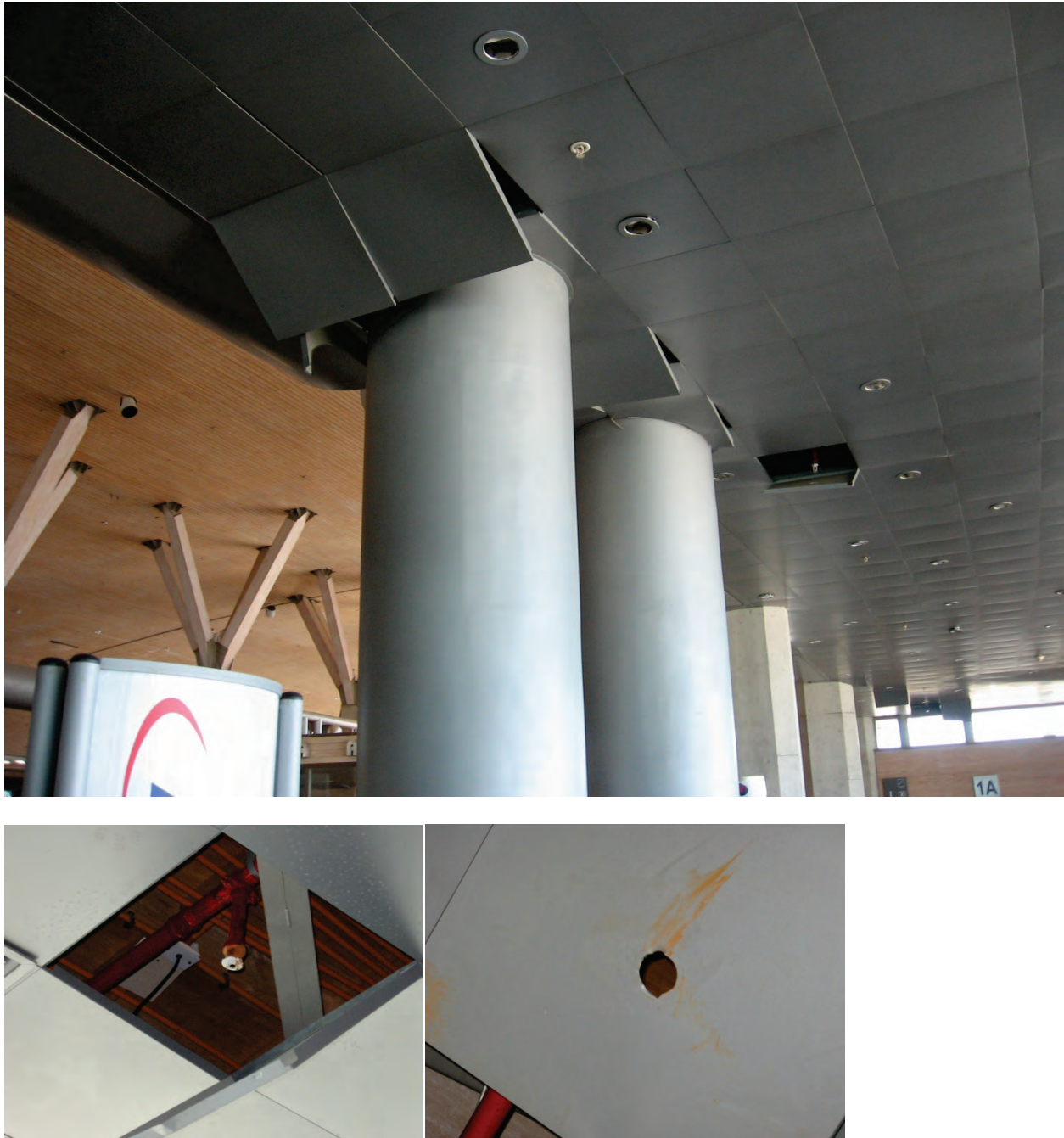
Figure 6.3.4.1-5 Damage to suspended metal panel ceiling system and fire sprinklers at Concepción airport, primarily at far end and around column obstructions in the 2010 Chile Earthquake (Photos courtesy of Rodrigo Retamales, Rubén Boroschek & Associates). The metal panel was strong enough to fail the sprinkler head shown at lower left.
