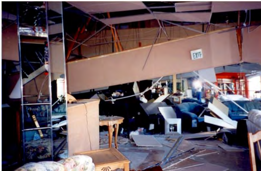
Figure 2.4.1-3 Failure of suspended ceilings and light fixtures in a furniture store (FEMA 74, 1994).
