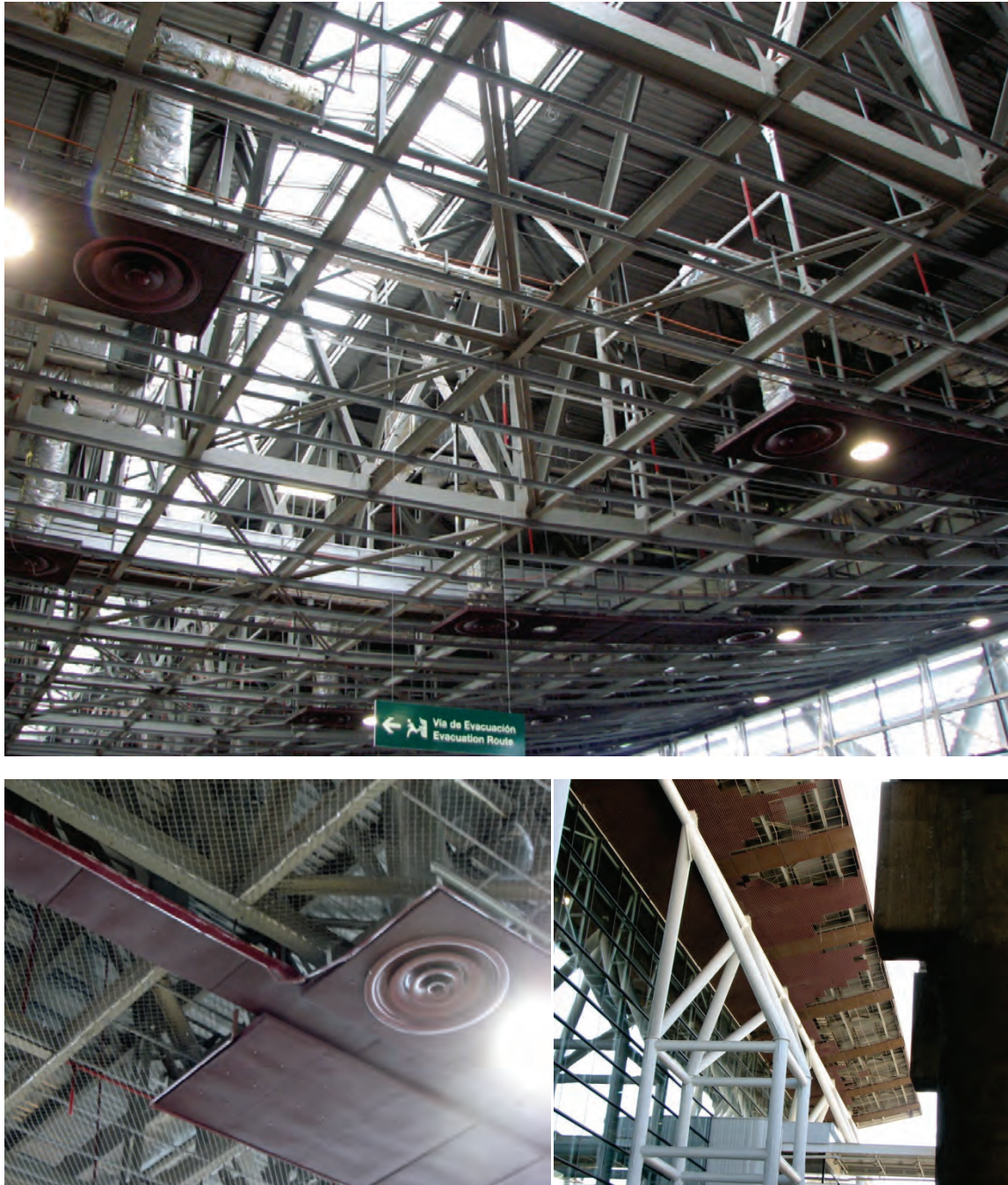
Figure 6.3.4.2-5 Extensive failure of ceiling in the main terminal of the Santiago airport in the 2010 Chile Earthquake. Metal panels with lights and diffusers hung from furring on short metal tabs; these remained in place but detail at lower left shows they also sustained some damage. Furring channels still in place throughout ceiling but majority of lightweight ceiling panels and much of the cross furring came down as shown at lower right photo of exterior soffit with same system (Photos courtesy of Antonio Iruretagoyena, Rubén Boroscchek & Associates).
