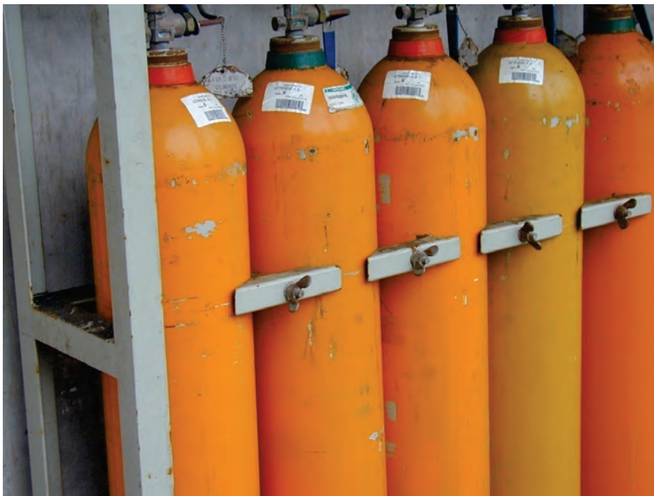
Figure 6.4.2.3-3 Detail of undamaged gas cylinder installation (Photo courtesy of Eduardo Fierro, BFP Engineers).
