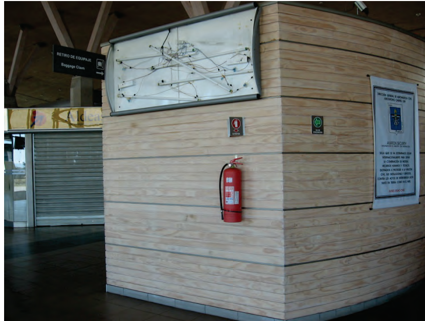
Figure 6.4.9.2-1 Numerous failures of ceilings and lights were observed at the Concepción airport in the 2010 magnitude-8.8 Chile Earthquake. Photo shows surface-mounted fixture on wall that remained in place but the lens fell and the bulbs were dislodged (Photo courtesy of Rodrigo Retamales, Rubén Boroscchek & Associates).
