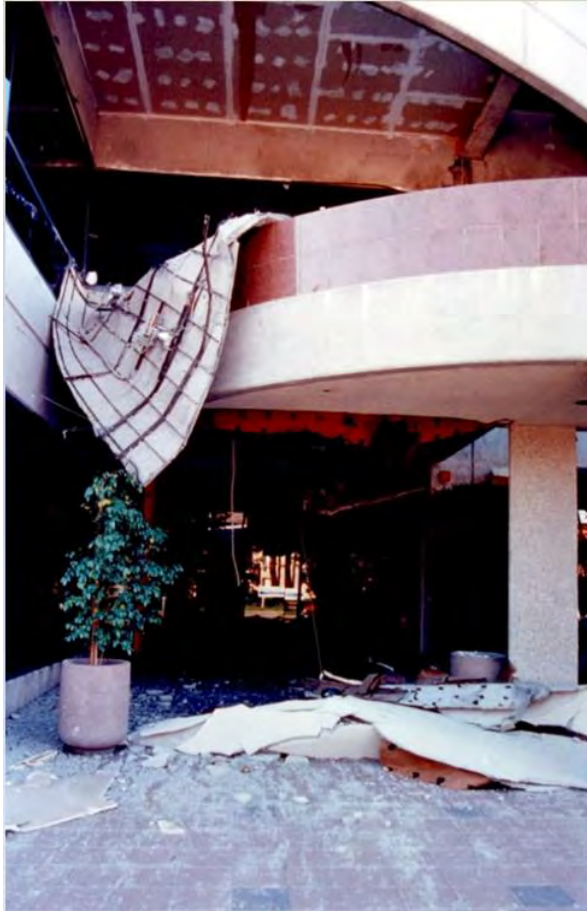
Figure 2.4.1-4 Failure of heavy stucco soffit at building entrance in the 1994 Northridge Earthquake (FEMA 74, 1994).
