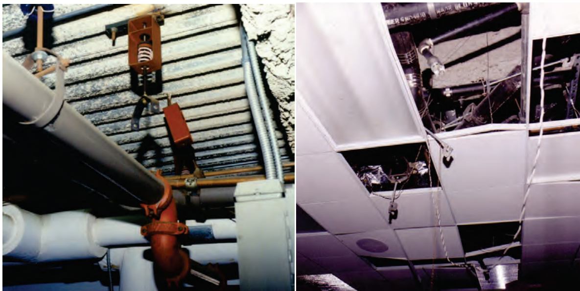
Figure 6.4.4.1-3 Damage to suspended fire protection piping from the 1994 Northridge Earthquake. Failed vibration isolators at left; failed C-clamps without beam clamp restraining straps shown at right (Photos courtesy of Mason Industries).
