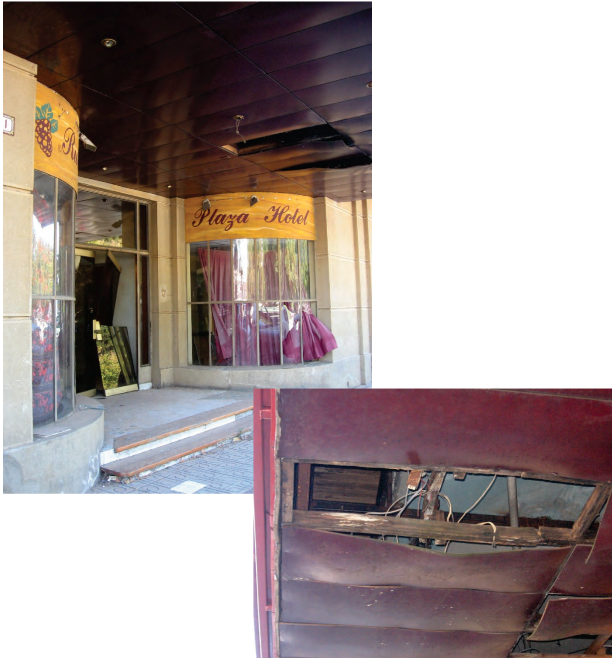
Figure 6.3.4.2-3 Damage to soffit paneling and wood framing at hotel in the 2010 Chile Earthquake; panels and wood framing show signs of prior water damage and deterioration. Note also damage to storefront glazing and glass doors (Photos courtesy of Rodrigo Retamales, Rubén Boroschek & Associates).
