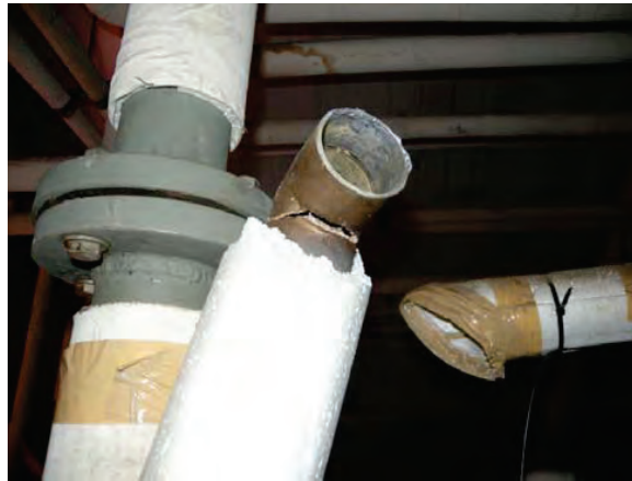
Figure 6.4.5.2-1 Broken copper hot water piping for at the San Carlos Hospital in the 2010 Chile Earthquake. Piping failure caused by movement of inadequately braced boiler shown at left (Photos courtesy of Gilberto Mosqueda, SUNY Buffalo).
