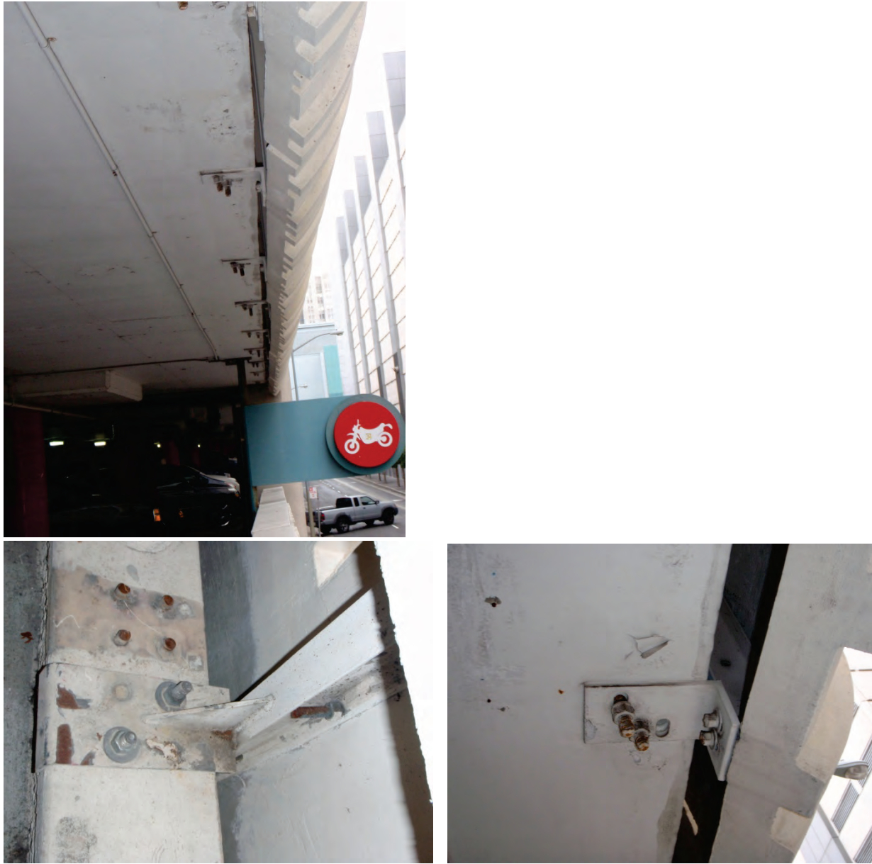
Figure 6.3.1.3-9 Precast spandrel panel in San Francisco parking garage supported by bearing connections near top of panel (left) and slotted connections at bottom of panel (right); panels have four connections each. The remnants of a previous nonductile connection detail are visible in the photo at left (Photo courtesy of Cynthia Perry, BFP Engineers).
