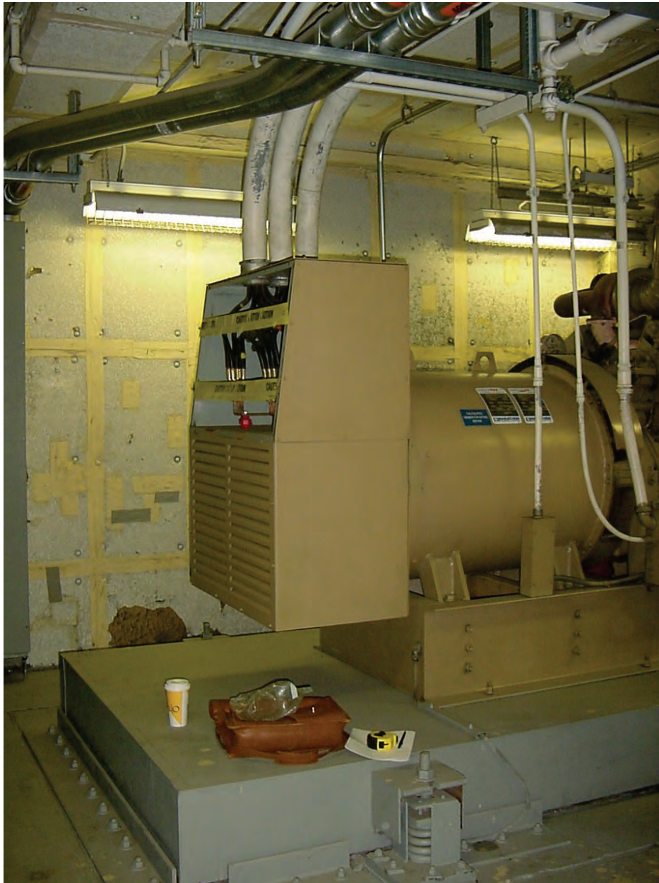
Figure 6.4.7.2-1 Emergency generator is anchored to a concrete inertia base. The inertia base is mounted on spring isolators and restrained by steel angle snubbers on all sides (Photo courtesy of Maryann Phipps, Estructure).
