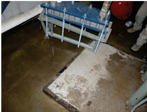
Figure 6.4.5.2-1 Broken copper hot water piping for at the San Carlos Hospital in the 2010 Chile Earthquake. Piping failure caused by movement of inadequately braced boiler shown at left (Photos courtesy of Gilberto Mosqueda, SUNY Buffalo).
