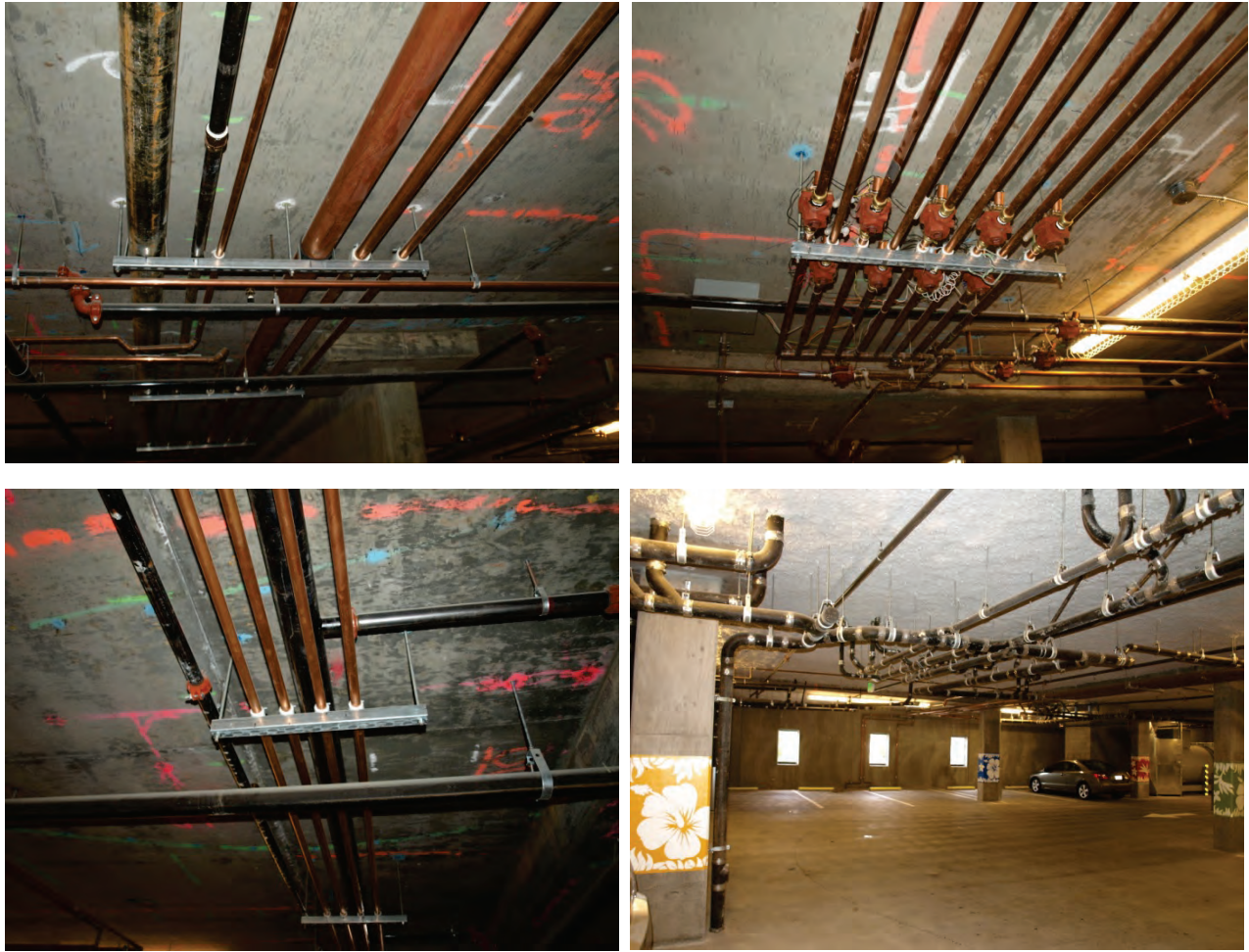
Figure 6.4.5.2-6 Piping installation in garage of mixed commercial/residential building San Francisco Bay Area completed in 2010. Note piping and trapeze supports do not have lateral restraints as all hangers were kept under 12" in length; only the sprinkler lines were laterally restrained. (Photo courtesy of Cynthia Perry, BFP Engineers).
