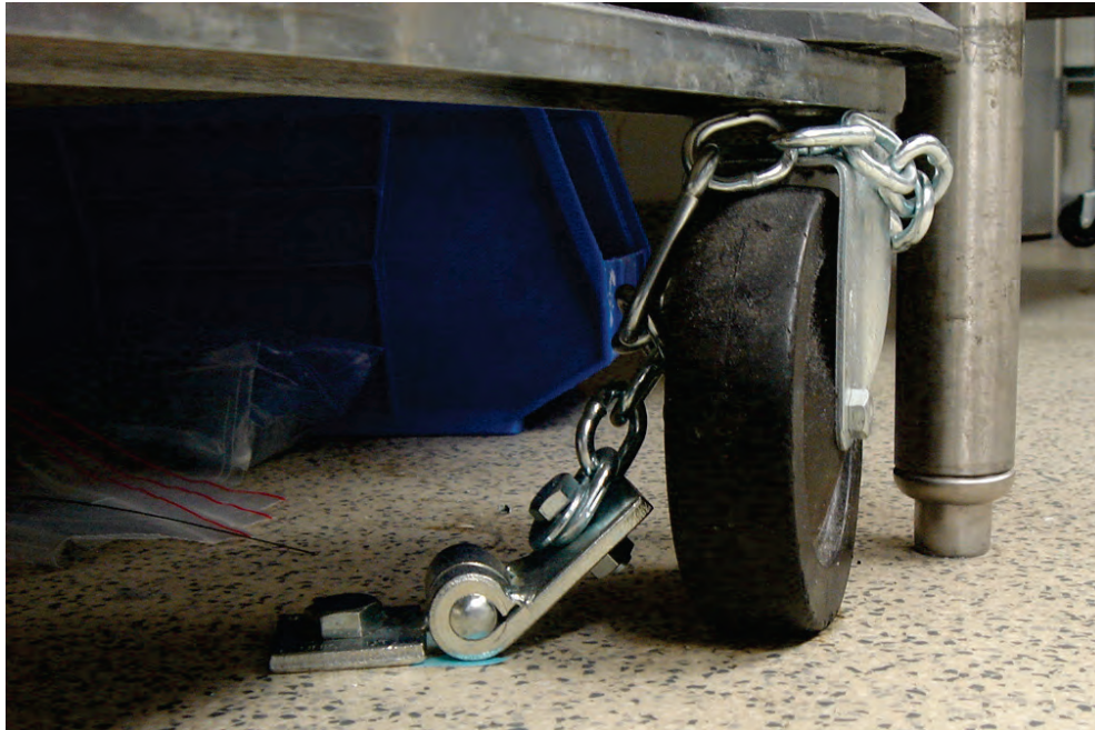
Figure 6.5.1.1-4 Alternate restraint at base of mobile shelving unit (Photo courtesy of Maryann Phipps, Estructure).
