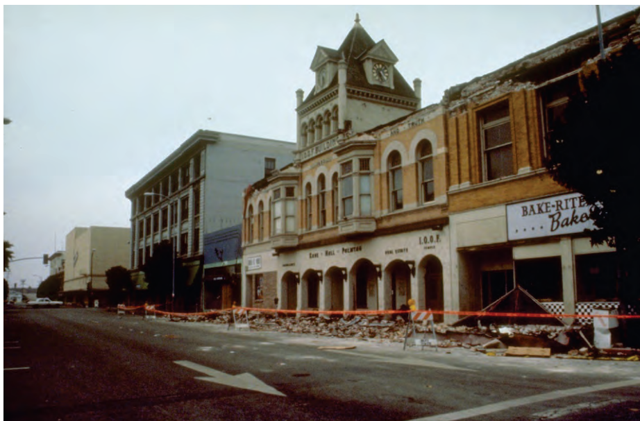
Figure 6.3.5.1-2 Unreinforced masonry parapet failures along Beach Street, Watsonville in the 1989 magnitude-6.9 Loma Prieta Earthquake (NGDC, 2009).
