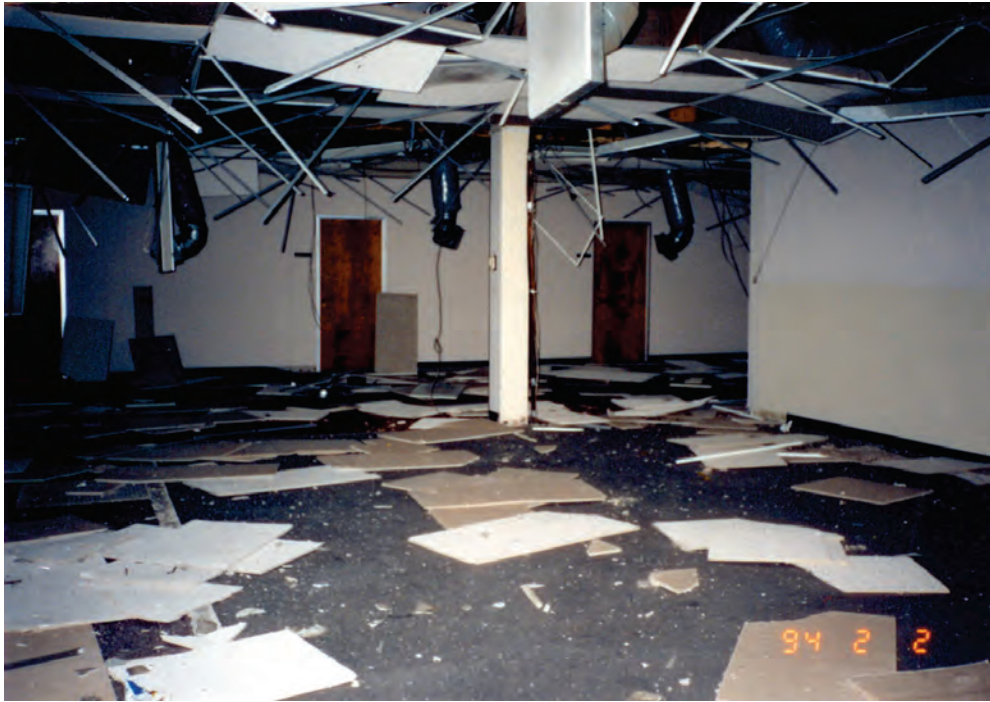
Figure 6.3.4.1-2 Failure of suspended ceiling system including lights and air diffusers in the 1994 Northridge Earthquake (Photo courtesy of Wiss, Janney, Elstner Associates).
