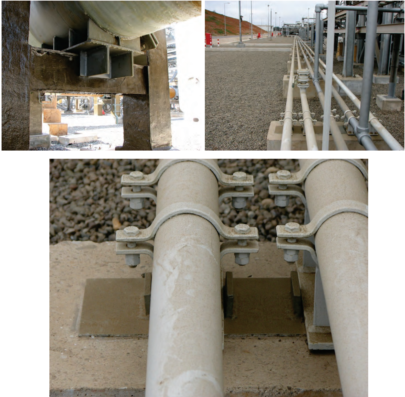
Figure 6.4.3.5-5 Floor-mounted supports for industrial piping in Chile; piping undamaged in the 2010 Chile Earthquake. The Chilean Industrial Code (Norma Chilena 2369) requires that shear forces be resisted by shear keys as shown; lower photo is detail of piping at upper right (Photos courtesy of Antonio Iruretagoyena, Rubén Boroschek & Associates).
