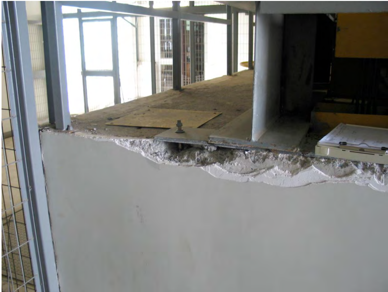
Figure 6.4.10.2-12 Anchor bolt failure of the elevator generator set due to inadequate edge distance for the bolts at the Los Angeles Regional Public Hospital in the 2010 Chile Earthquake (Photo courtesy of Bill Holmes, Rutherford & Chekene).
