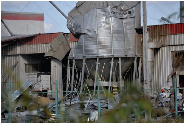
Figure 6.4.1.2-2 Damage to silos, conveyors and equipment at a grain operation in the 2010 magnitude-8.8 Chile Earthquake (Photos courtesy of Eduardo Fierro, BFP Engineers).
