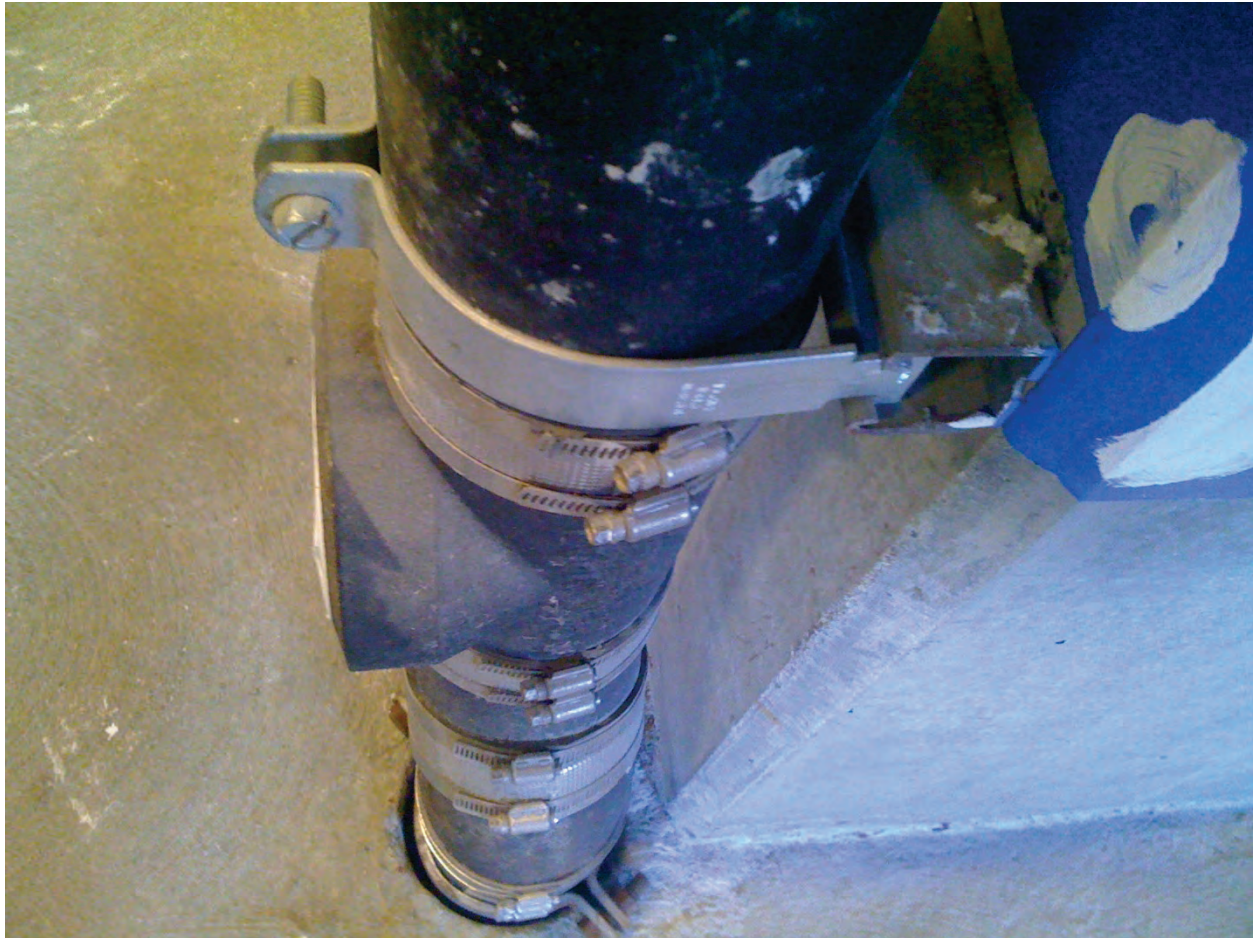
Figure 6.4.5.2-5 Poor example of sanitary sewer pipe support installed in San Francisco Bay Area in 2010; strut clamp has inadequate edge distance to end of strut and could slip off the end (Photo courtesy of Cynthia Perry, BFP Engineers).
