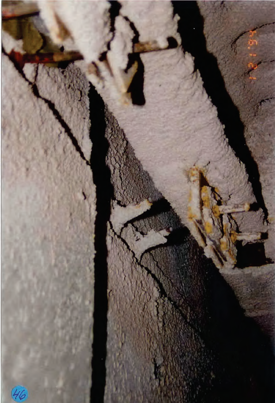
Figure 6.3.1.3-5 Close-up photo of two fractured connection bolts in a prefabricated panel in the 1994 Northridge Earthquake; corrosion of the rods may have contributed to the failure. (Photo courtesy of OSHPD).
