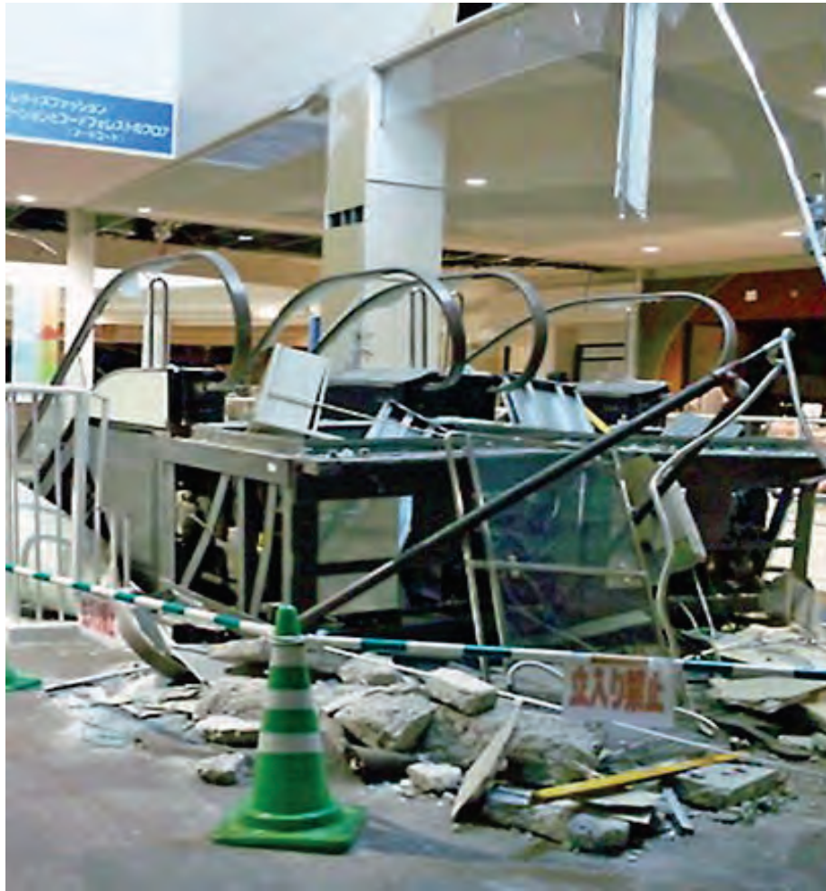
Figure 6.4.10.3-1 Photo of escalator, located in the Sendai area of Japan, which fell from the floor above onto the escalator on the floor below during the magnitude-9.0 Great Tohoku Earthquake of March 11, 2011. The probable cause of this collapse was that the relative displacements between floors exceeded the connection bearing width capacity of the escalator. This type of failure creates a serious life safety hazard (Photo source: Nekkei Architecture).
