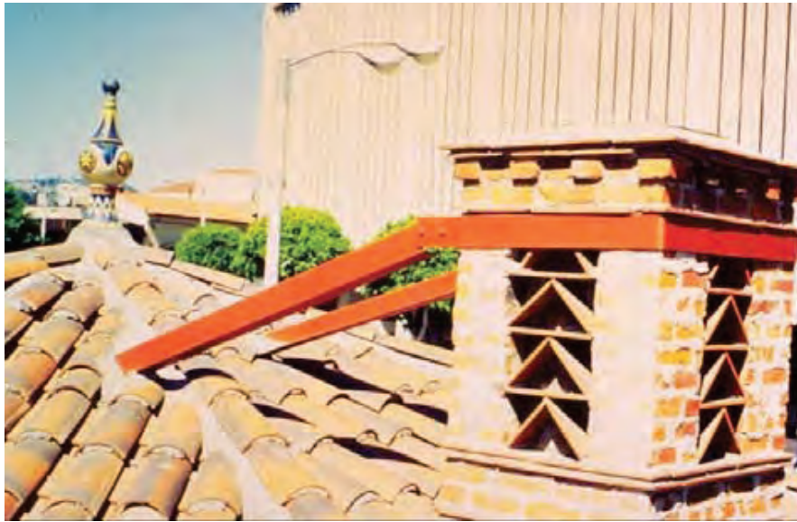
Figure 6.3.7.1-4 Braced chimney (FEMA, 2004).
