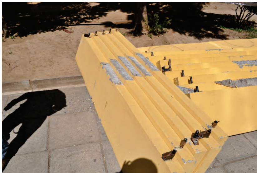
Figure 6.3.1.3-7 Numerous precast panels removed to prevent falling; detail from residential building in Rancagua, Chile above. These panels had a bearing seat at the center and supported on steel dowels at either end (Photo courtesy of Eduardo Fierro, BFP Engineers).
