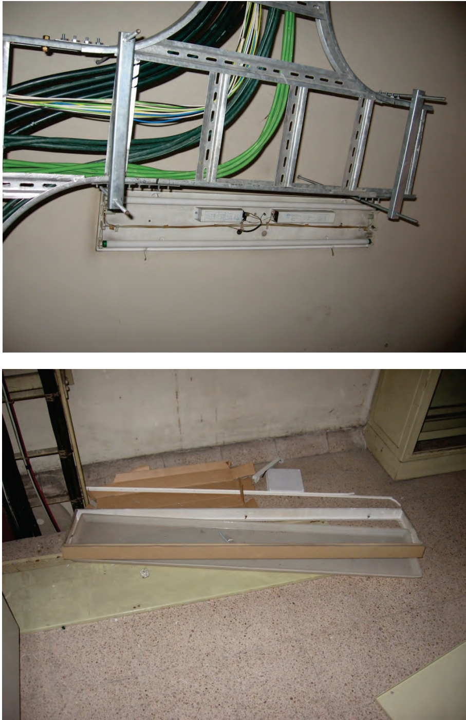
Figure 6.4.9.2-2 Overhead surface-mounted fixture anchored to underside of concrete slab damaged in the 2010 Chile Earthquake. Back of fixture housing remained anchored to the concrete slab above and the bulbs remained in place but the lens and sides of housing fell indicating that internal connections in the fixture were inadequate (Photos courtesy of Rodrigo Retamales, Rubén Boroschek & Associates).
