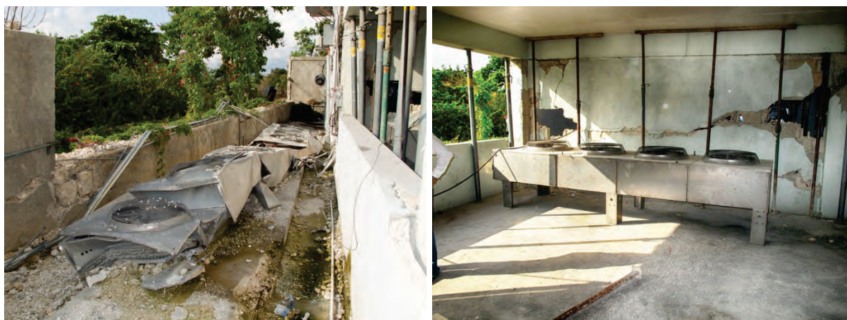
Figure 6.4.7.3-7 Heat rejection mechanical units which provide cooling for servers in cellular carrier central network facility (left photo). Collapsing security wall during the 2010 M 7.0 Haiti Earthquake crushed these units and resulted cyclical total failure of the cellular network as the servers hit temperature limits, shut down, rebooted and heated up again. System stability was restored by replacing the damaged units with temporary ones (right photo). Example of how the reliability of a critical facility essential system is both dependent upon adequate seismic restraints and a location which is free of structural and nonstructural falling hazards (photos courtesy of Philip J. Caldwell).
