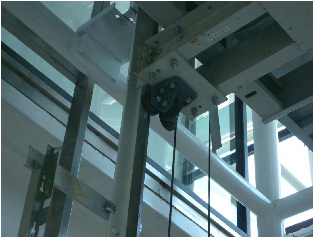
Figure 6.4.10.2-9 Derailed car roller assembly of the guide rail at the Santiago airport in the 2010 Chile Earthquake (Photo courtesy of Gilberto Mosqueda, SUNY Buffalo). The three rollers are supposed to travel along three sides of the stem of the T-shaped steel guide rail.
