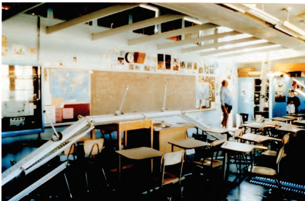
Figure 6.4.9.3-1 Failure of a strip of pendant light fixtures at Dawson Elementary School library as a result of the 1983 magnitude-6.4 Coalinga Earthquake. Note that in this case the support stems failed at the ceiling connection and the stem came down with the lights (Gary McGavin, NGDC, 2009).
