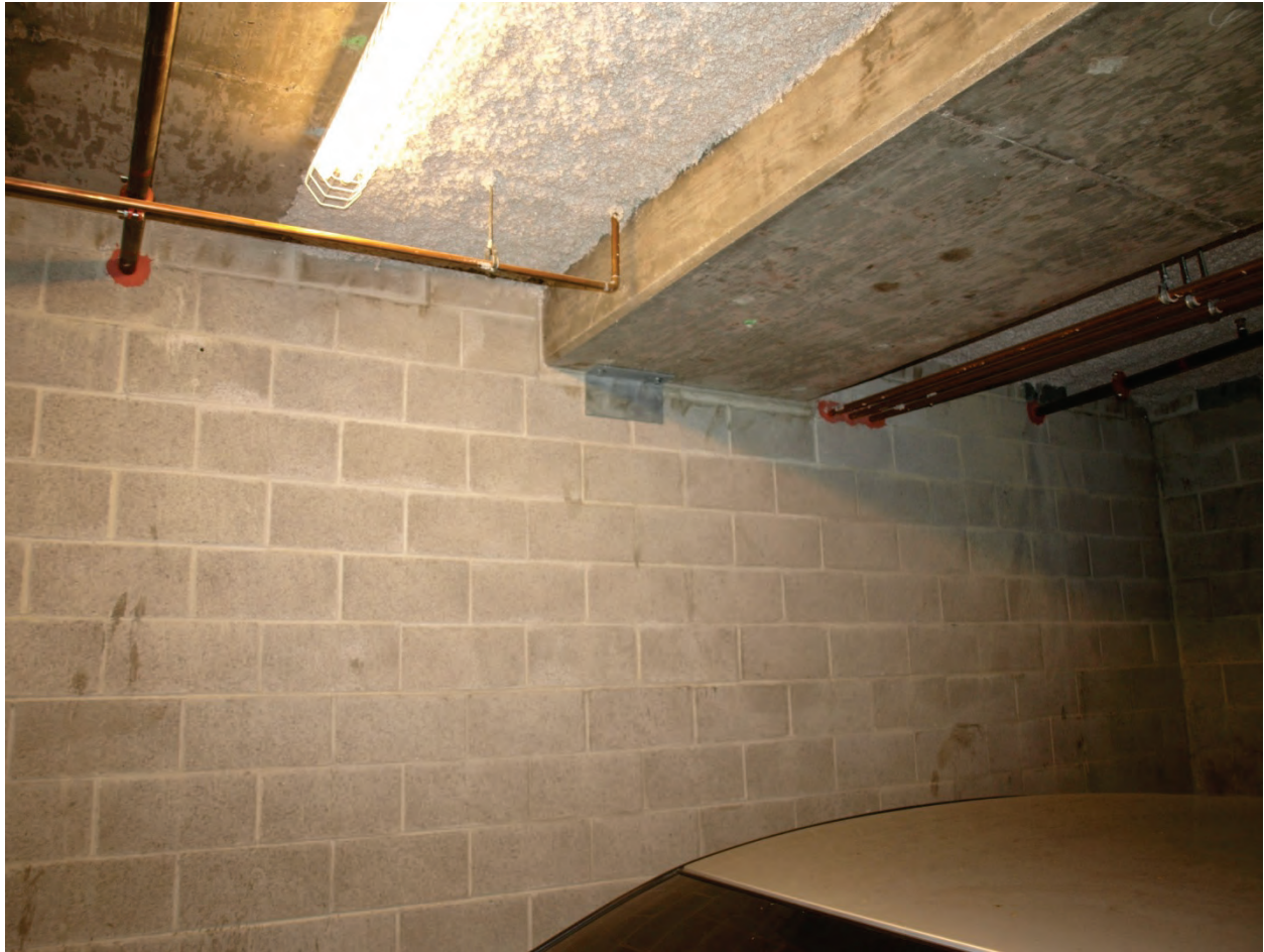
Figure 6.4.3.8-6 Series of pipe penetrations through a full-height CMU partition wall. Note pipe suspended from floor above; partition anchored to floor below and detailed with steel clip angles intended to provide lateral restraint for the wall but allow relative slip between the wall and slab above. The hangers will move with the floor above and the pipe at penetration will move with the wall. Lateral restraints are located immediately above floor (Photo courtesy Cynthia Perry, BFP Engineers).
