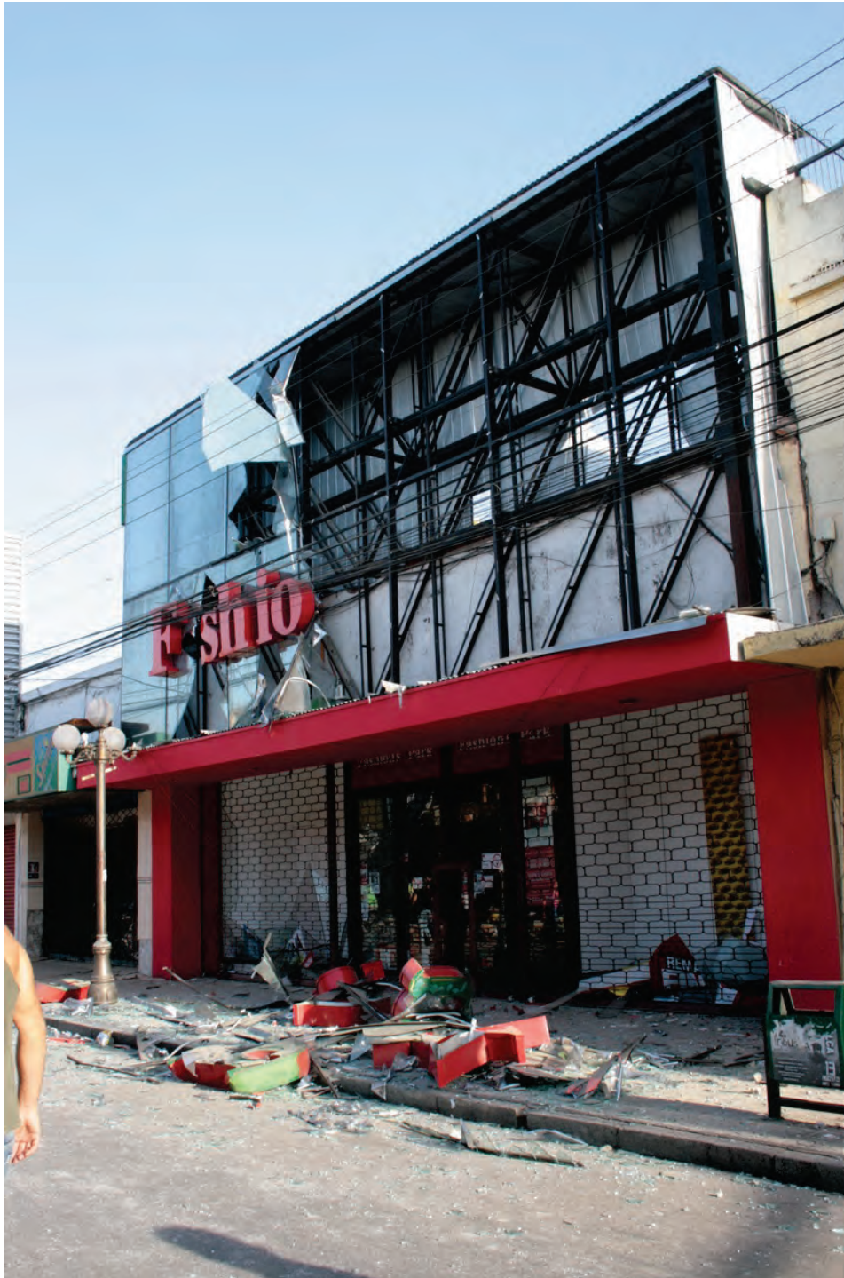
Figure 6.3.1.4-4 Glazing damage, due in part to pounding with the structure at right during the 2010 Chile Earthquake (Photo courtesy of Antonio Iruretagoyena, Rubén Boroscheck & Associates).
