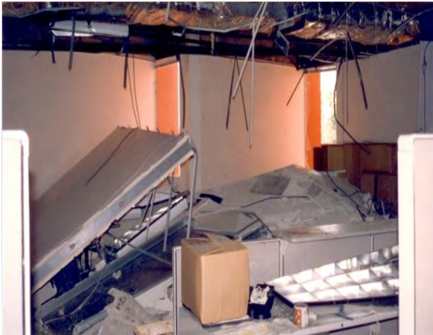
Figure 2.4.1-1 Failure of office partitions, ceilings, and light fixtures in the 1994 Northridge Earthquake (FEMA 74, 1994).
