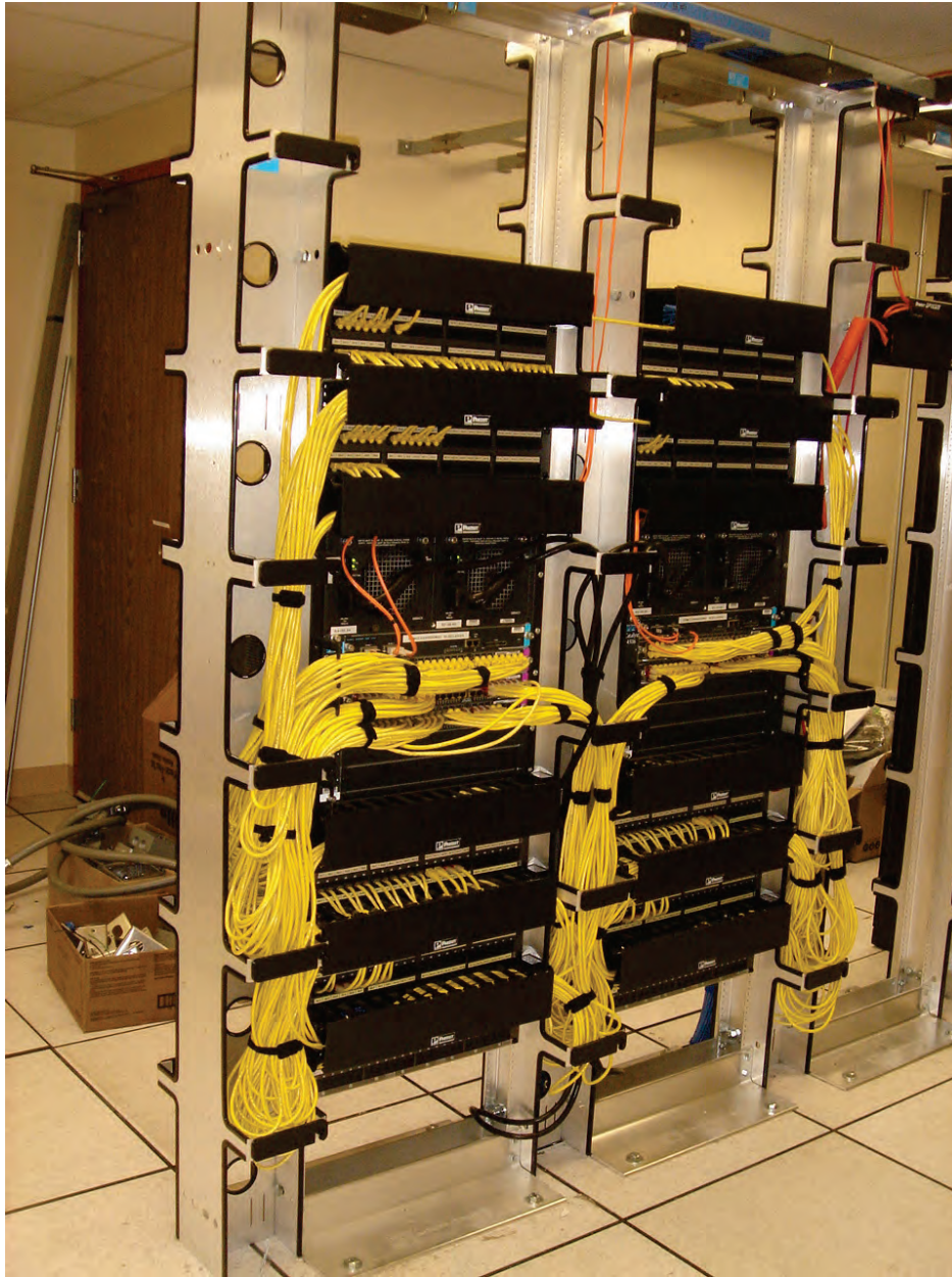
Figure 6.5.3.1-5 Data rack bolted through access floor to supplemental strut bracing below (Photo courtesy of Maryann Phipps, Estructure).
