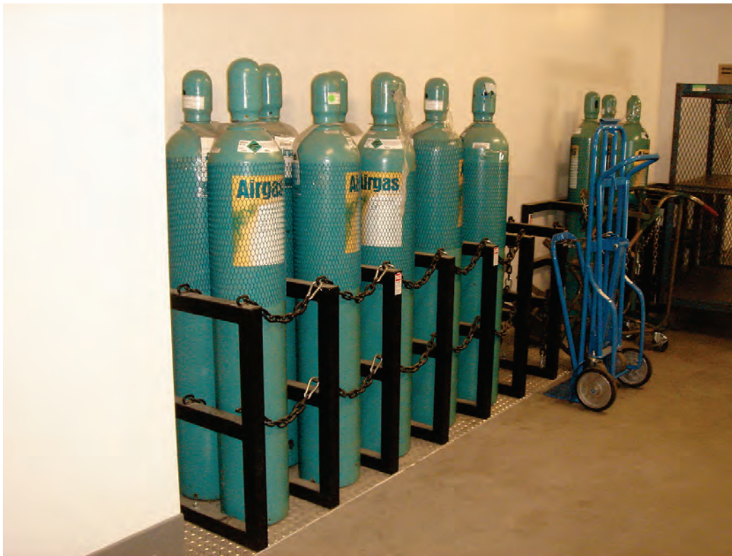
Figure 6.4.2.3-7 Detail of enclosures for airgas tanks in a hospital; chains attached with quick release hooks (Photo courtesy of Maryann Phipps, Estructure).
