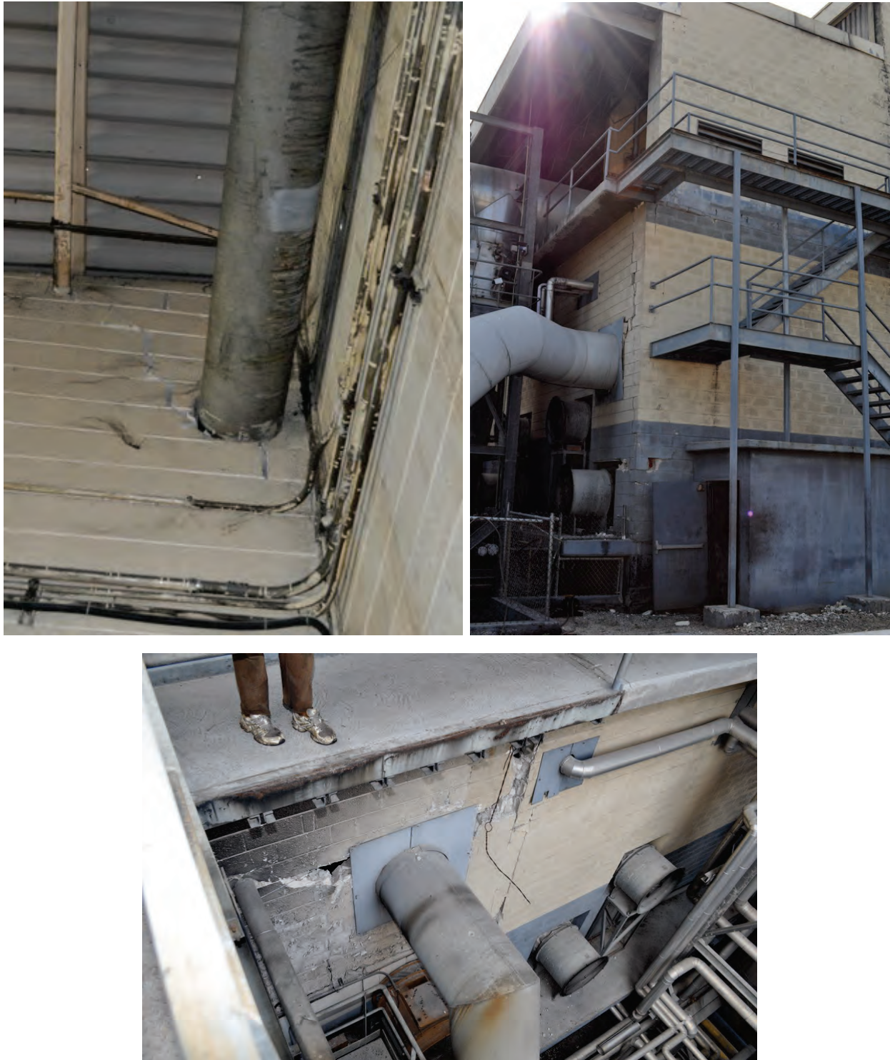
Figure 6.4.3.8-3 Wall penetrations for piping and ducts contributed to damage to unreinforced masonry walls at an industrial facility in the 2010 magnitude-7 Haiti Earthquake (Photos courtesy of Eduardo Fierro, BFP Engineers). The piping and ducts were not damaged but the walls cracked and will need to be repaired.
