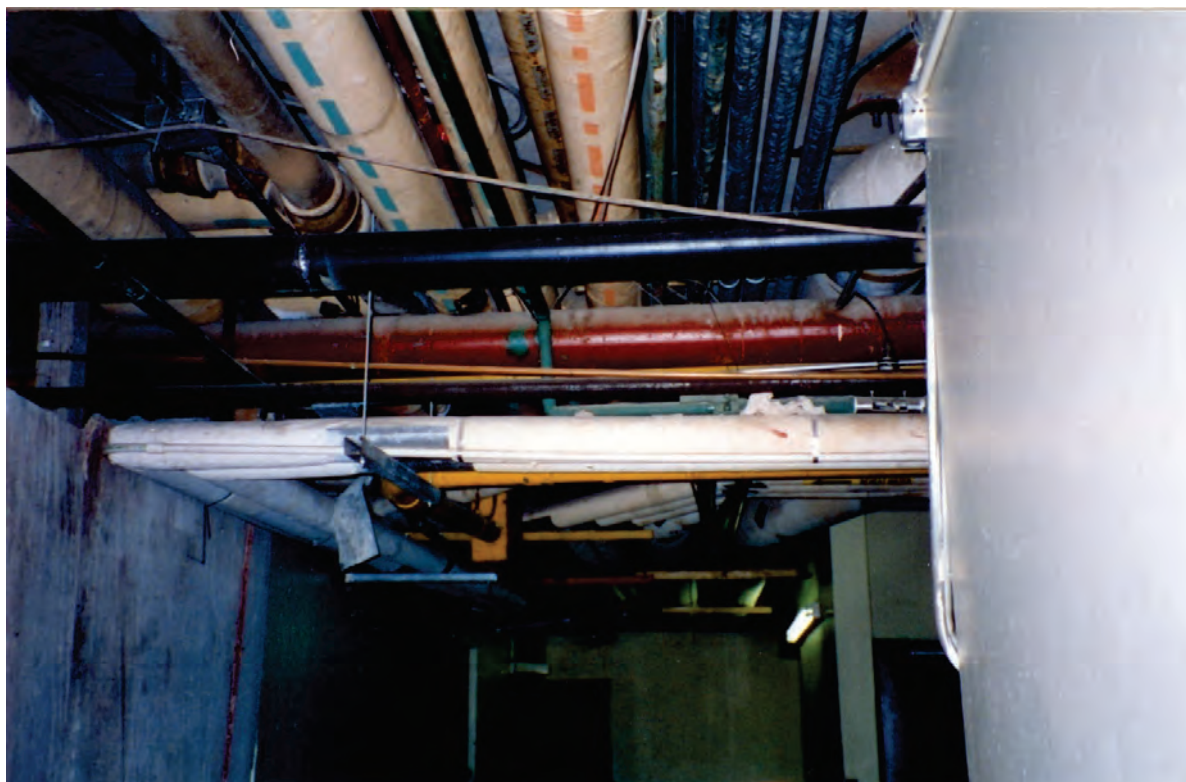
Figure 6.4.8.1-1 Unbraced suspended piping and conduit (Photo courtesy of Wiss, Janney, Elstner Associates).
