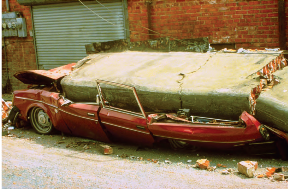
Figure 6.3.5.1-1 URM parapet fell and smashed two cars in the 1992 magnitude-7.2 Petrolia Earthquake. A parapet at same location in Ferndale, California failed in 1906 and killed two cows (NGDC, 2009).
