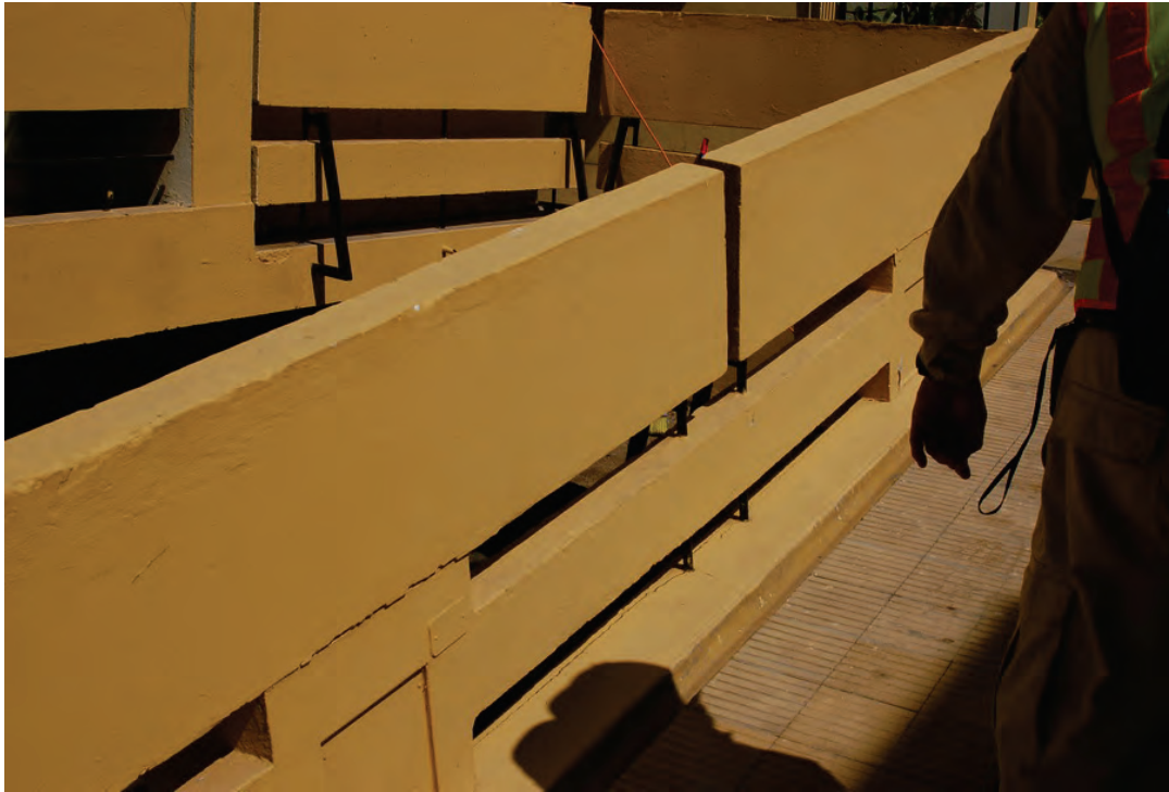
Figure 6.3.1.3-6 Residential building with precast concrete corridor and balcony railing panels. Some panels were damaged and subsequently many were removed to prevent falling. Location in Rancagua, Chile 154 miles northeast of the epicenter; estimated PGA of 0.3g during the 2010 magnitude-8.8 Chile Earthquake (Photo courtesy of Antonio Iruretagoyena, Rubén Boroscchek & Associates).
