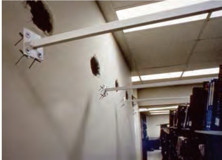
Figure 6.5.2.2-2 Failure of overhead transverse bracing for bookshelves were anchored to gypsum board partition in the 1984 magnitude-6.2 Morgan Hill Earthquake (Photo courtesy of Santa Clara County Office of Emergency Services). The anchors were not attached to wall studs, only to gypsum board.
