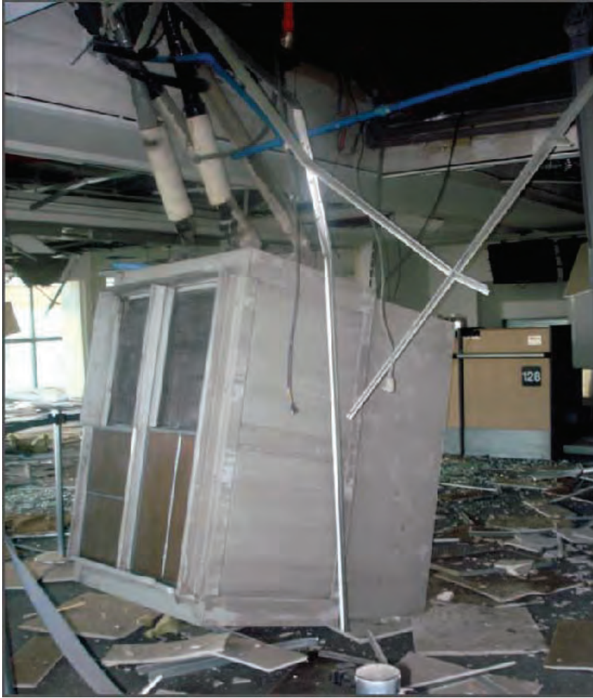
Figure 6.4.1.5-3 Suspended HVAC equipment came down at the Santiago airport terminal in the 2010 magnitude-8.8 Chile Earthquake (Photo courtesy of Gokhan Pekcan).
