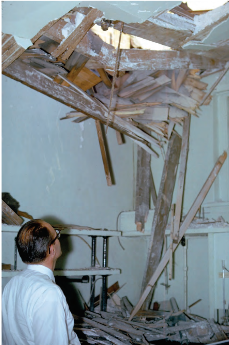
Figure 6.3.5.1-3 Damage to roof framing caused by failure of overhanging brick masonry during the 1962 magnitude-5.8 Cache Valley, Utah earthquake (Photo courtesy of PEER Steinbrugge Collection, No. S828).
