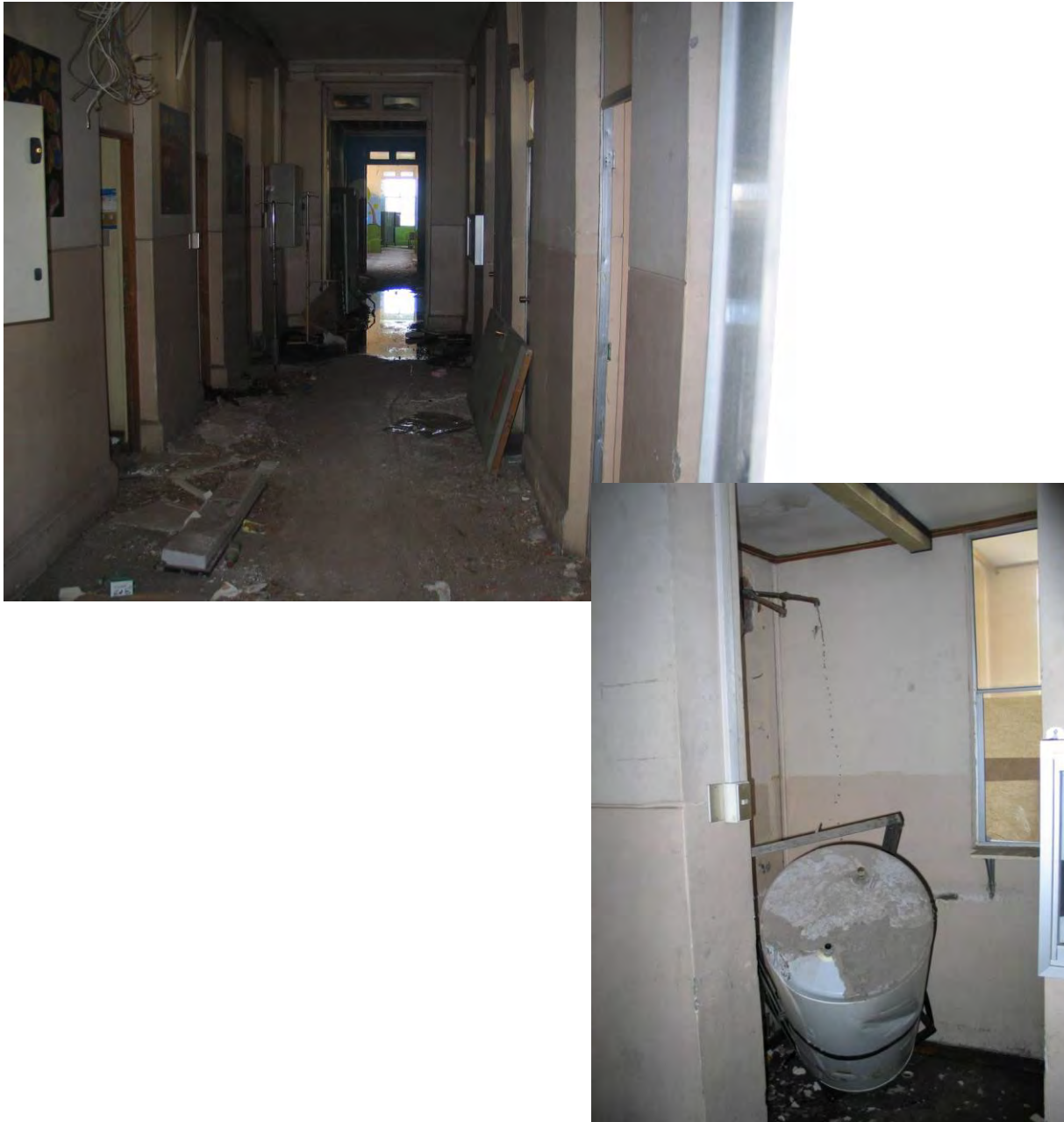
Figure 6.4.2.4-2 Water damage at the Talca Hospital in the 2010 magnitude-8.8 Chile Earthquake; water leaking from tank at right. This building was closed due to nonstructural damage, dominated by water damage (Photos courtesy of Bill Holmes, Rutherford & Chekene).
