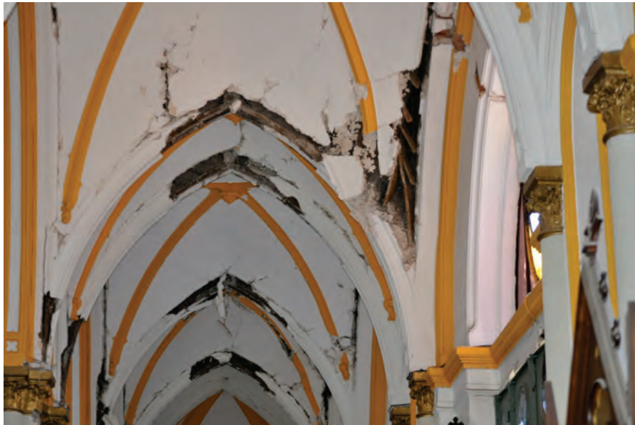
Figure 6.3.4.3-1 Damage to ornate wire lath and plaster ceiling in the 2010 magnitude-8.8 Chile Earthquake (Photo courtesy of Eduardo Fierro, BFP Engineers). Wire lath is attached to arches or to wood furring suspended from the roof framing.
