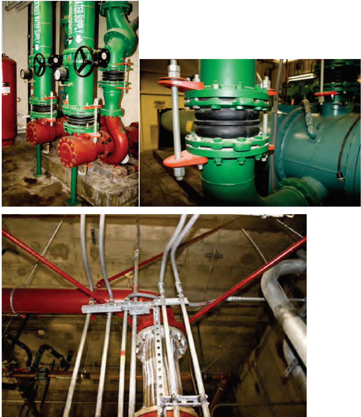
Figure 6.4.3.3-2 Examples of flexible couplings that performed well in the 2010 magnitude-7 Haiti Earthquake; the building suffered relatively minor damage (Photo courtesy of Tom Sawyer, Engineering News Record).
