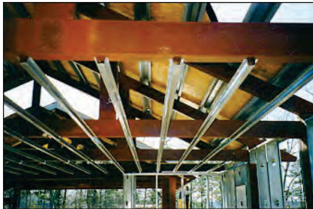
Figure 6.3.4.2-6 Mitigation examples with 1-1/2" hat channels at 16" on centers screwed in place with #12 self drilling screws and furring strips ready to receive gypsum board (Photo courtesy of Excalibur Steel). No special seismic details are required for this type of ceiling where the gypsum board is well secured directly to furring strips.
