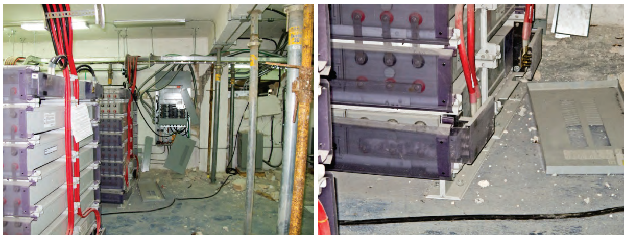
Figure 6.4.7.3-6 Battery room for central network cell phone carrier after 2010 M 7.0 Haiti Earthquake. Three-story building which contained the UPS (uninterruptable power supply) and battery room was newly constructed and suffered near collapse structural damage which required structural demolition and replacement. Note that high mass batteries with integral structural system was rigidly anchored and sustained no damage or loss of operation despite building structural system displacing enough to shear support columns. Cellular carrier representative advised that the central network support functionality was maintained during Earthquake (photos courtesy of Philip J. Caldwell).
