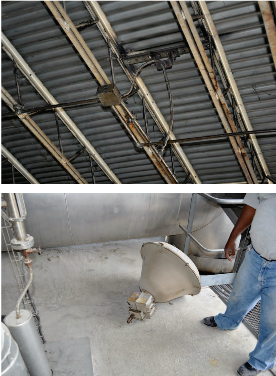
Figure 6.4.9.3-3 Failure of pendant light fixture in the 2010 magnitude-7 Haiti Earthquake; stem of fixture broke and conduit pulled loose (Photos courtesy of Eduardo Fierro, BFP Engineers).
