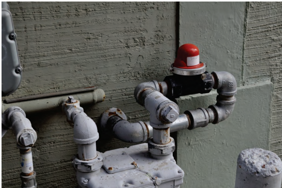
Figure 6.4.5.1-8 Two examples of seismic shut-off valves in San Francisco Bay Area. Top photo at Marine Mammal Center; lower photo at six unit apartment building in Oakland (Photos courtesy of Cynthia Perry, BFP Engineers).
