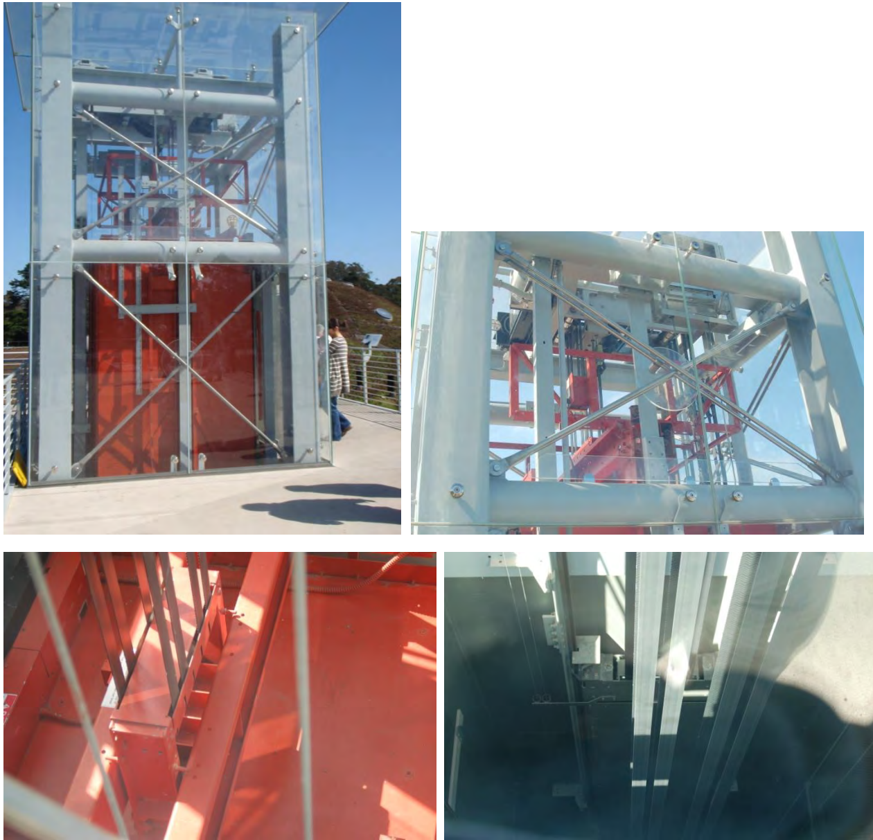
Figure 6.4.10.2-13 Small "machine-roomless" traction elevator with flat belts at the Academy of Sciences, San Francisco, California (Photos courtesy of Eduardo Fierro, BFP Engineers). Clockwise: Overview of elevator at roof; view of guide rails and sheaves; top of cab showing belts; view down shaft at belts, counterweight, guide rails and guide rail brackets.
