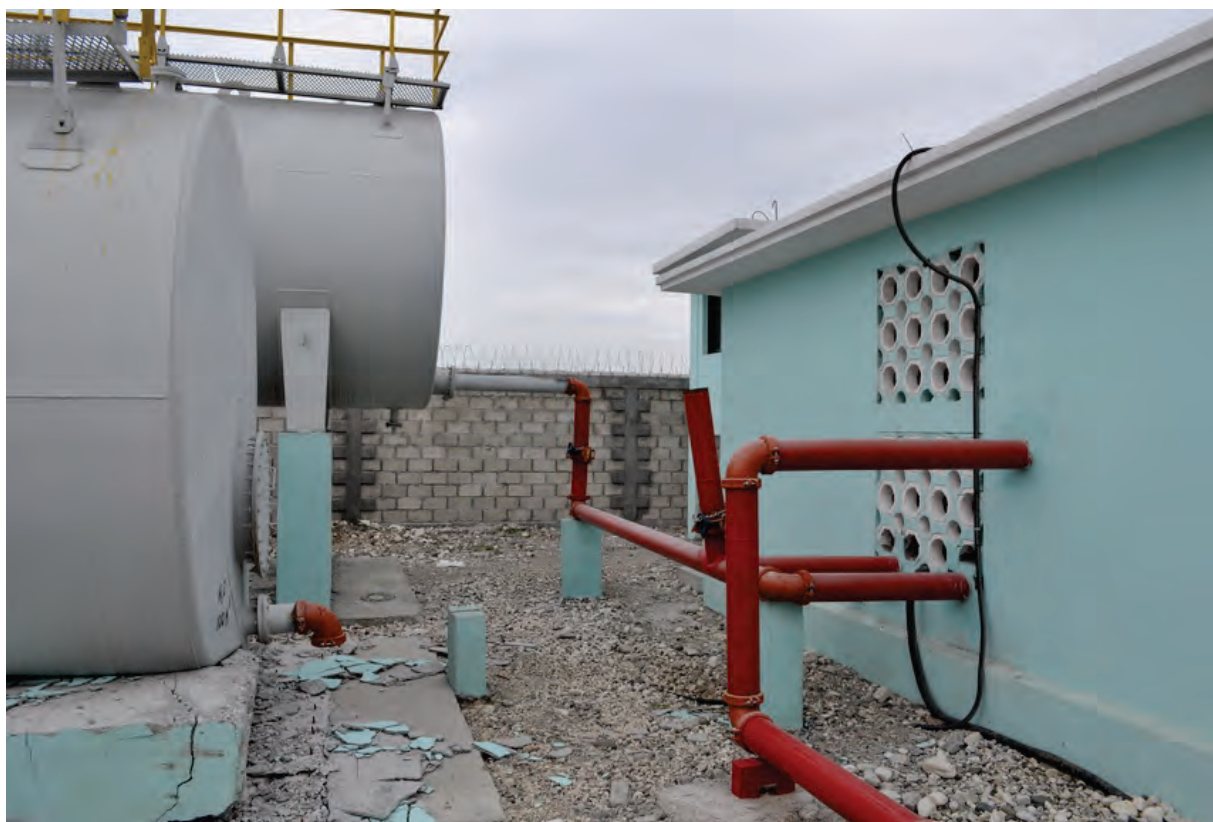
Figure 6.4.4.1-4 Collapse of water tank at left and broken piping disabled the fire protection system at this power plant in Port-au-Prince and led to the temporary plant closure in the 2010 magnitude-7 Haiti Earthquake (Photo courtesy of Eduardo Fierro, BFP Engineers).
