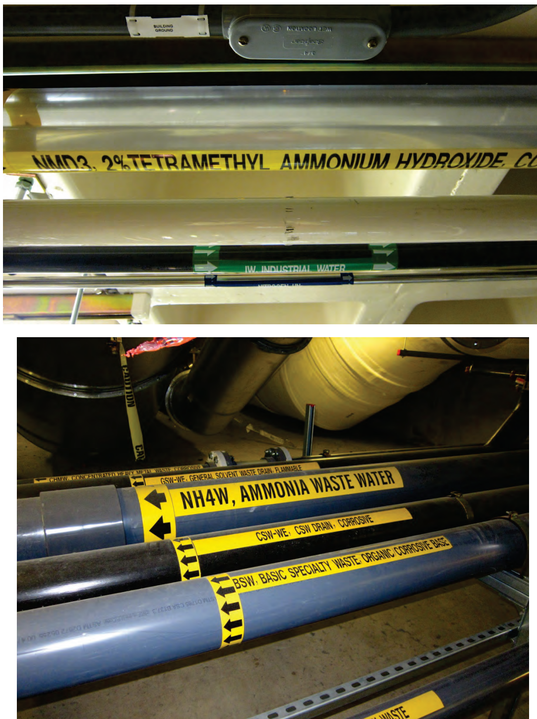
Figure 6.4.5.1-5 Two examples of double walled piping used for secondary containment of hazardous fluids. Preassembled double walled pipe with centering devices or spacers separating the inner and outer pipe is available commercially, but as shown here, the outer pipe was installed and leak tested prior to pulling the inner pipe through. Note the yellow color coded labels indicate reactive materials; flow direction also marked prominently (Photos courtesy of Jeffrey Soulages, Intel Corporation).
