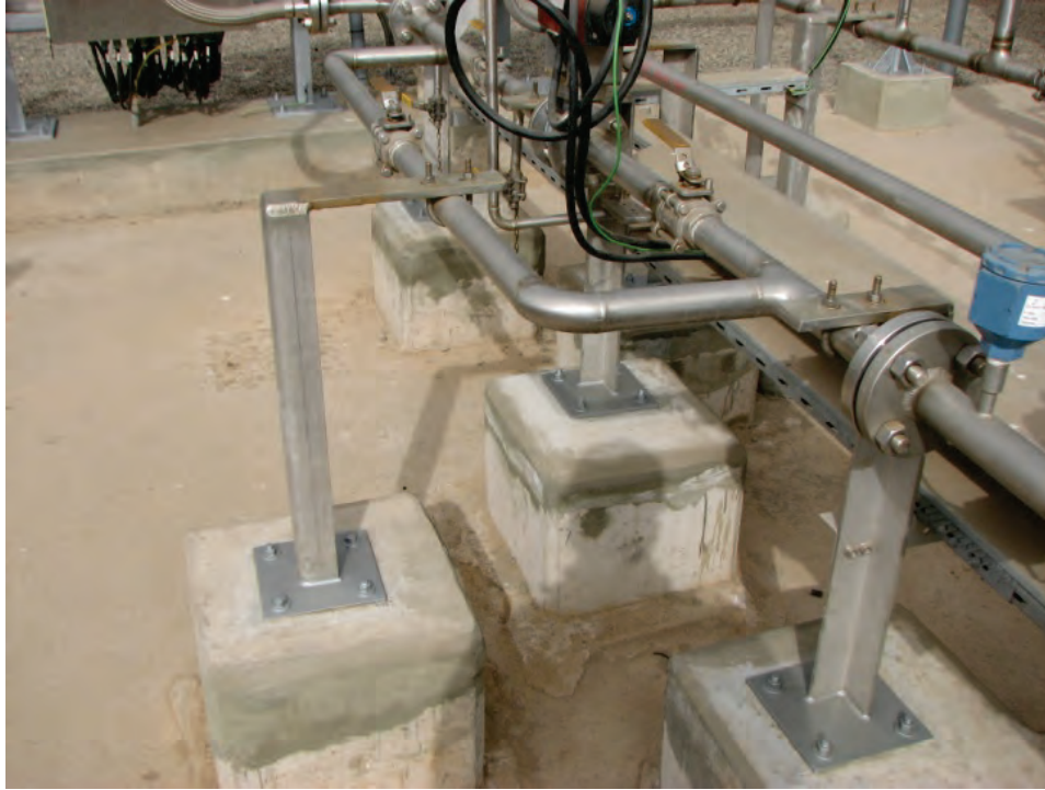
Figure 6.4.3.5-4 Floor/ground-mounted supports for industrial piping in Chile; piping undamaged in the 2010 magnitude-8.8 Chile Earthquake. Pipe supports include concrete pedestal, base plate, and built-up welded support stand. (Photos courtesy of Antonio Iruretagoyena, Rubén Boroschek & Associates).
