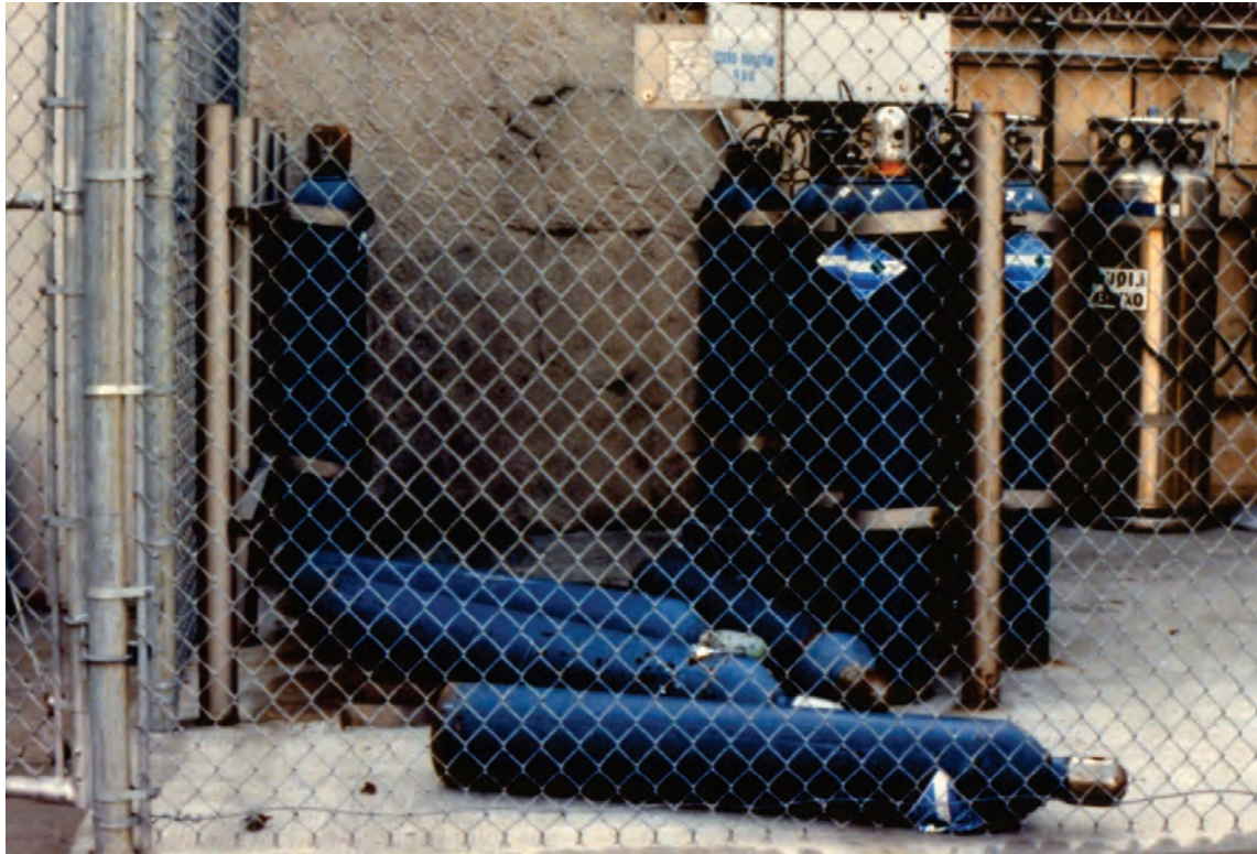
Figure 6.4.2.3-1 Unanchored tanks inside fenced enclosure in the 1994 magnitude-6.7 Northridge Earthquake (Photo courtesy of OSHPD).
