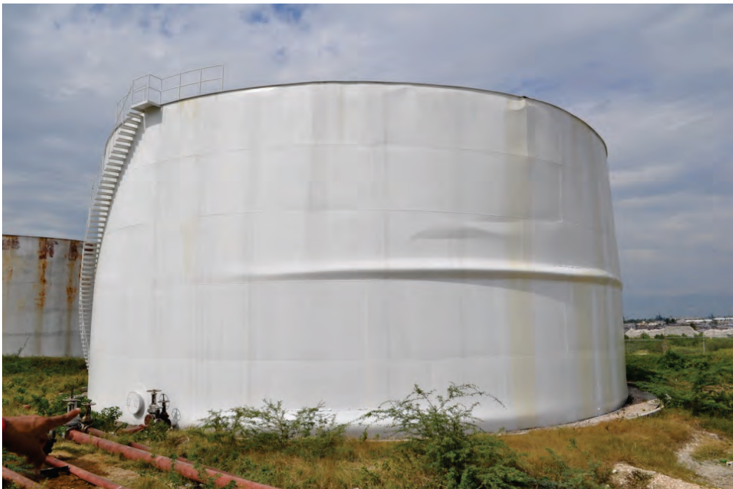
Figure 6.4.2.2-3 Tank with “elephant’s foot” and “elephant knee” in Port-au-Prince in the 2010 magnitude-7 Haiti Earthquake (Photo courtesy of Eduardo Fierro, BFP Engineers).
