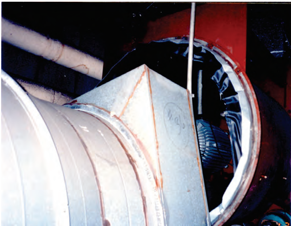
Figure 6.4.1.5-2 Sheet metal duct separated from suspended fan unit (Photo courtesy of Wiss, Jenney, Elstner Associates).
