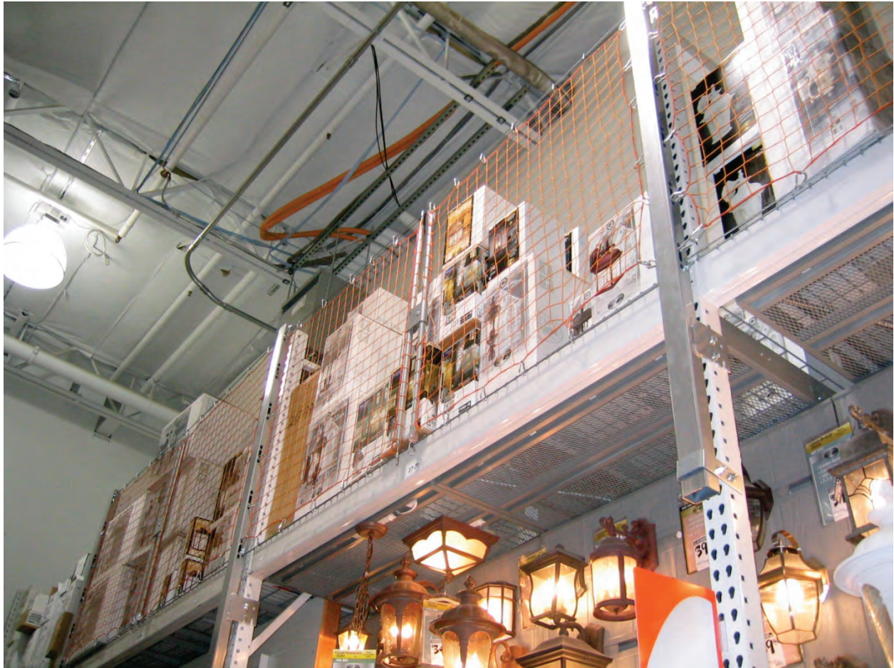
Figure 6.5.1.2-6 Photo showing netting used to keep storage on upper portions of steel storage racks in a big box hardware store (Photo courtesy of Mike Mahoney, FEMA).
