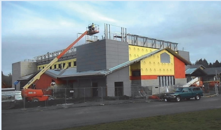
Figure TS-4 Ocosta Elementary School's heavily reinforced vertical evacuation structure under construction in Westport, Washington (Magistrale, 2015).
