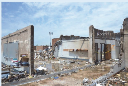
Figure TO-13 Damaged hallway where seven fatalities occurred (most of the debris has already been removed). This hallway area was a “designated area of safety” (NIST, 2013).
