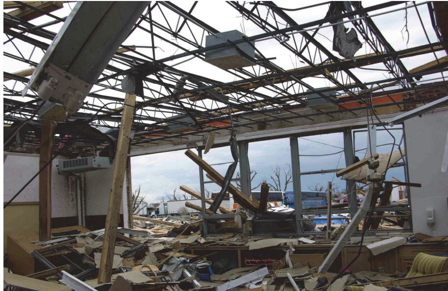
Figure TO-4 Wind-borne debris in a classroom in Greensburg, Kansas in 2007. Note that all of the exterior windows are broken and the roof deck was blown off. (Photo source: Thomas Smith, FEMA)
