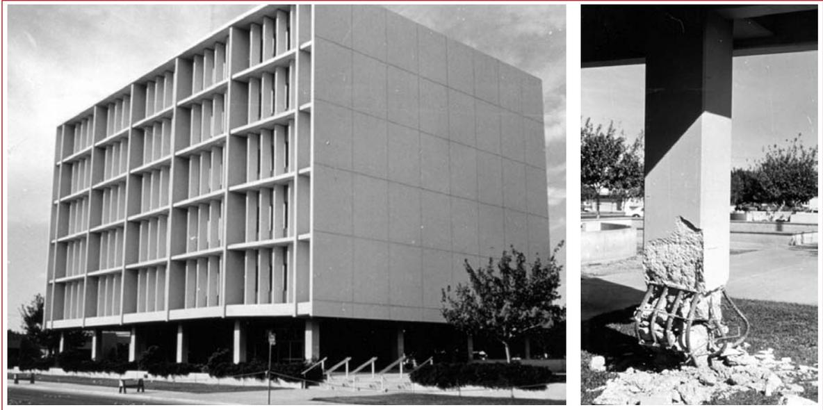
This six-story structure had several types of irregularity including end shear walls that stopped below the second floor and a first story with less strength and stiffness than the stories above. As a result, earthquake energy dissipation and damage were concentrated in the first story columns, a condition that could not be repaired and required demolition of the building after the earthquake. In a more severe earthquake, this type of damage could have caused the building to collapse.
