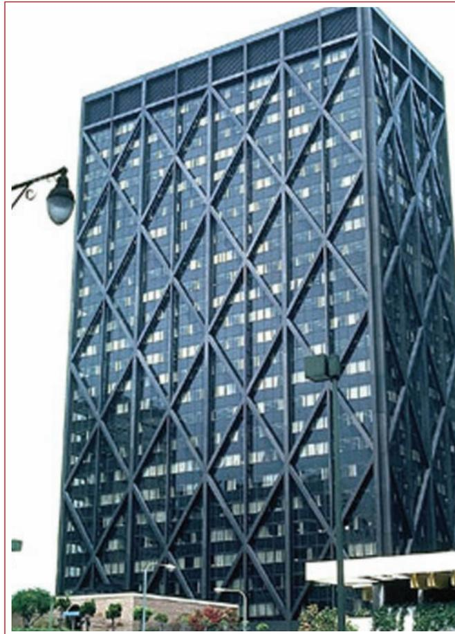
Figure 24 A high-rise braced frame building in San Francisco, California.
