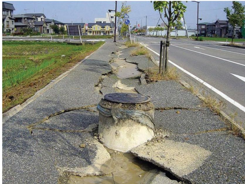
Figure 6 Top photo shows liquefaction-induced settlement of apartment buildings in the 1964 earthquake in Nigata, Japan (photo courtesy of the University of Washington). The bottom photo shows one of many manholes that floated to the surface as a result of soil liquefaction caused by the 2004 Chuetsu earthquake near Nigata, Japan (photo courtesy of Wikimedia Commons).
