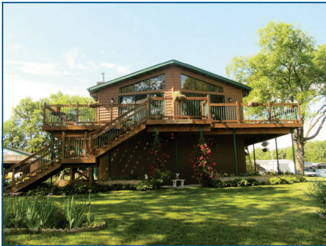
Figure 3: Elevated Residence within SFHA in Cedar Falls, Iowa (Photo courtesy of City of Cedar Falls, Iowa)
