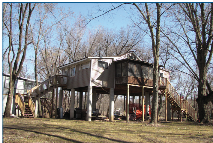
Figure 8: An elevated house on concrete columns which originally had a slab on grade, Linn County, Iowa. (Photo courtesy of Linn County, Iowa Planning & Development)
