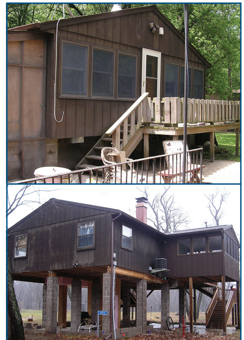
Figure 1: This house located in Linn County, Iowa was elevated resulting in reduced flood risk and lower flood insurance premiums. The original condition is shown on the top and the elevated structure is shown below. (Photos courtesy of Linn County, Iowa Planning & Development)
