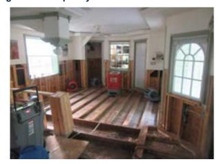
Figure 31. Sleeper System Installed Over a Concrete
