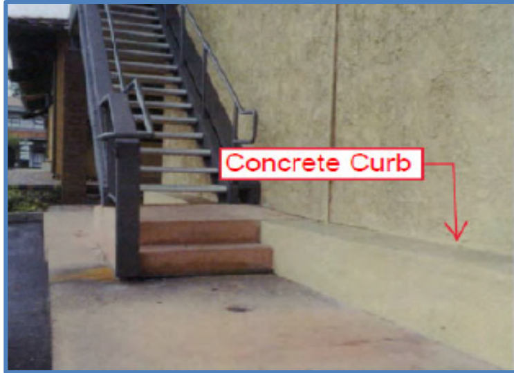
Figure 21: Not an Acceptable Retrofit Option to Modify the LAG
