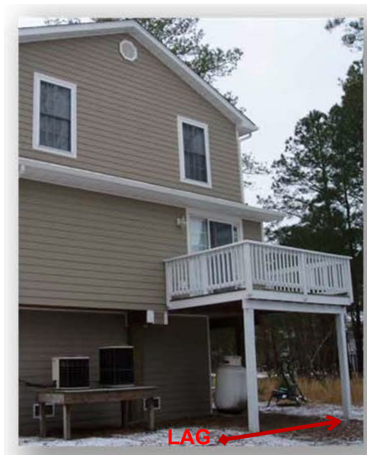
Figure 2: LAG - Structure with Attached Deck
