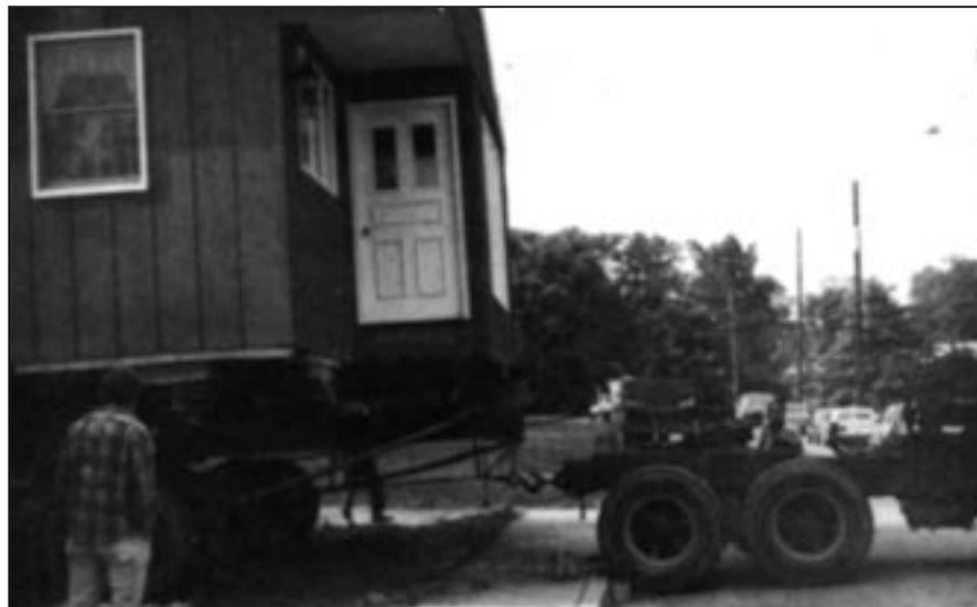
At the new site, the moving contractor positions the house over the partially completed foundation and supports the house on cribbing so the trailer wheels can be removed. As in the house elevation process described in Chapter 5, the house is lifted on hydraulic jacks to the desired height and the foundation is completed below it (see Figure 7-4). The house is then lowered onto the foundation, all utilities are connected, and any necessary backfilling and landscaping is completed.
