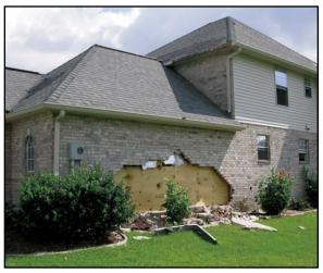
Figure 1. Failed brick veneer. Plastic foam wall sheathing was installed over the wood studs (plywood was temporarily installed after the brick failure).
