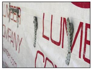
Figure 4. These four ties were never embedded into the mortar joint.
