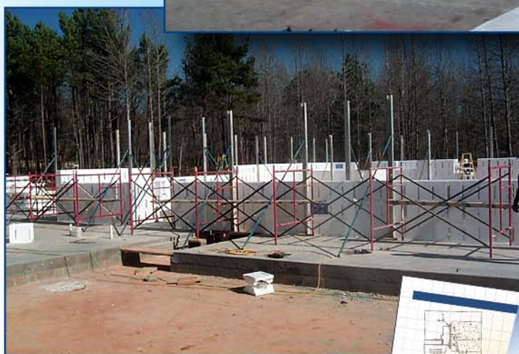
Erection of the reinforced ICF walls.
