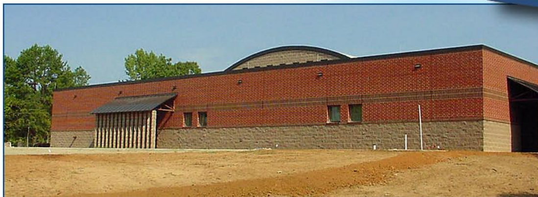
Completed reinforced ICF walls.
