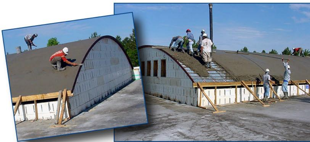
Construction of the steel-truss roof system.
