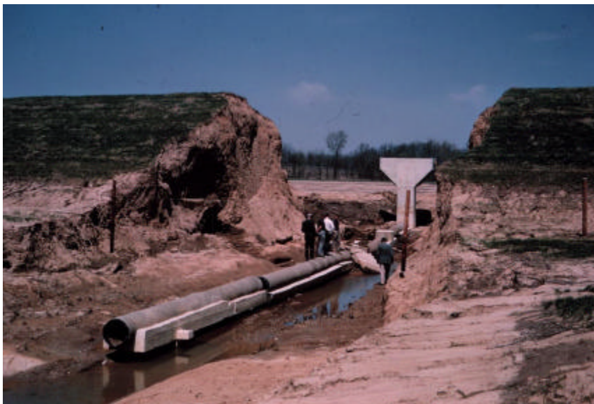
Figure 3 – Obion Creek #36 – looking upstream into reservoir
