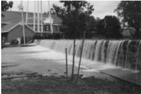
Overtopping of the Washington Forge Pond Dam in August 2000. Dam has masonry downstream face.
