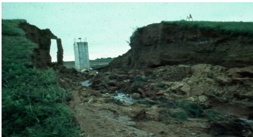
Clayton County Waste Water Pond Dam 1982
