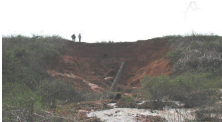
Pritchard's Lake Dam Morgan County March 2001
