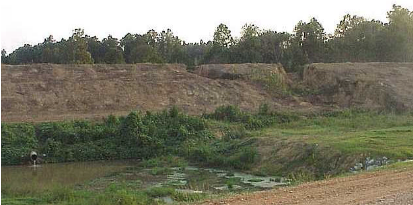
Figure 4 – Ascalmore #11 – looking upstream, note pipe outlet on left
