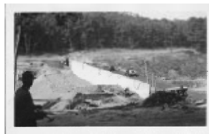
Construction of core wall at West Branch Reservoir Dam
