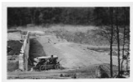
Construction of core wall at West Branch Reservoir Dam
