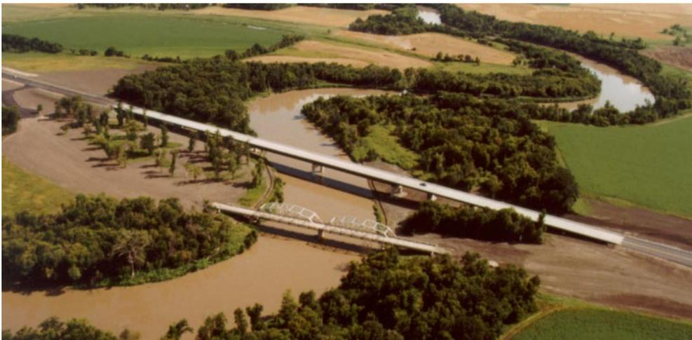
*New bridge (top) is 11 feet higher and three times longer than the old bridge (bottom), which has since been demolished. (Right side of photo is North Dakota.) Photo courtesy of Randy Aarestad, Halstad, Minnesota.*
