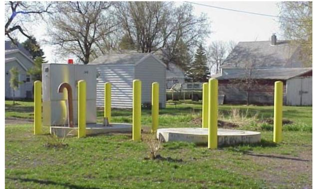
*A new master lift station has been built away from the river in an area that now can be better protected from flooding. Removing the old lift station from the edge of the riverbank also enables the city to construct temporary dikes to keep floodwaters getting into town.*
