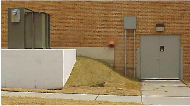
*In addition to elevating electrical equipment (left), engineers also outfitted 24 major doors and windows (right) with special metal shields that can be attached ahead of time to keep out floodwaters.*
