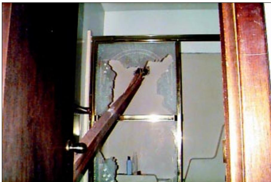
**FIGURE 6-22:** A 10-ft long 2-in by 6-in missile penetrated the exterior wall of an apartment in this multi-family house, which was sheathed with hardboard panels. The missile, which was generated from the vortex of a strong tornado, then penetrated the gypsum board and plastic tile tub enclosure, the tempered glass shower door, and the interior partition near the door frame. At the interior partition, it pierced through a stud and projected a few inches into the hallway (Figure 6-23).
