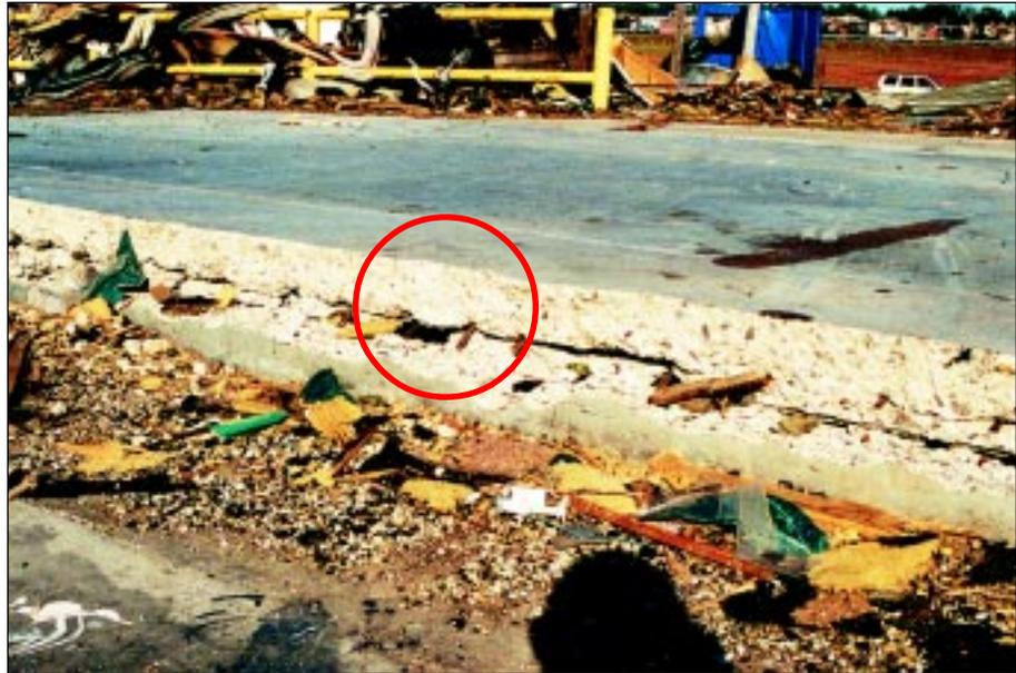
approximately 200 yards from a violent tornado vortex near Del City, Oklahoma. As can be seen in Figure 5-16, the wall was heavily reinforced at the foundation level. However, lack of support at the top of the wall permitted the wall to blow outward and collapse.
