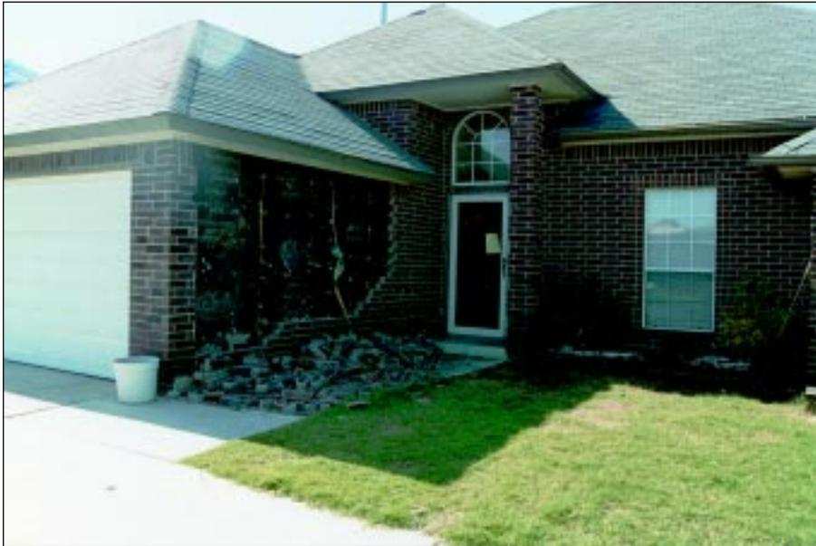
**FIGURE 4-38: Failure of brick veneer wall, collapsed on the ground. This home, located outside Oklahoma City was on the periphery of a violent tornado.**
