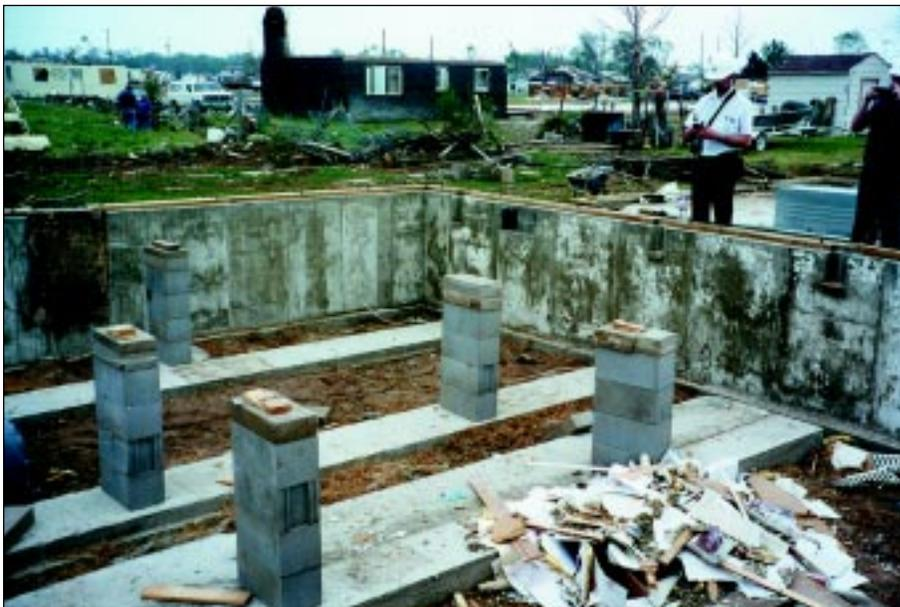
**FIGURE 4-55:** *Lack of bolts or positive connectors present between the chassis and foundation of a double-wide manufactured house, Haysville, Kansas. The floor framing of the house was still resting on the foundation after the tornado passed.*
