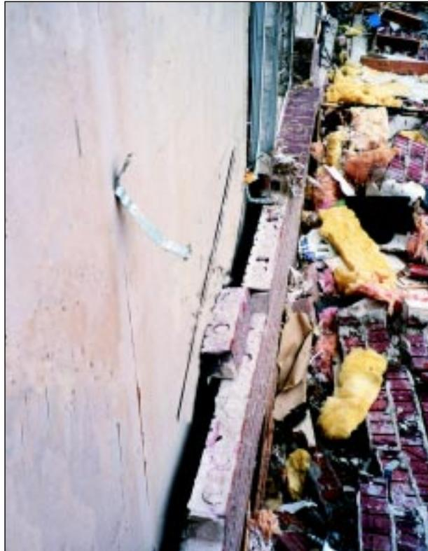
**FIGURE 4-37:** *Failure of brick veneer wall, Del City, Oklahoma.*
