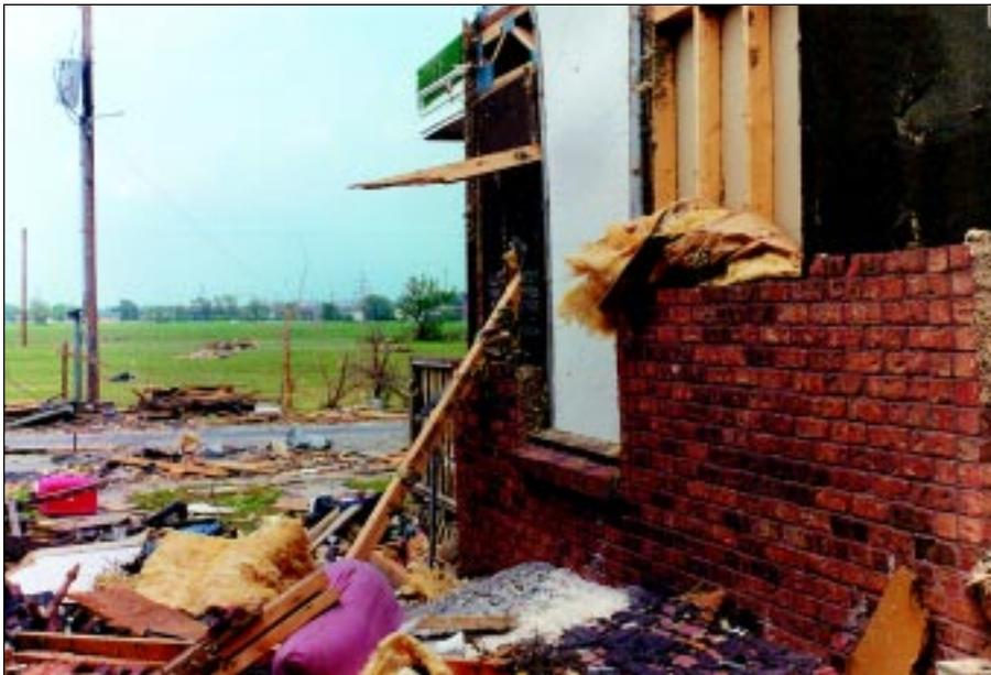
**FIGURE 4-45: Failure of brick veneer at a multi-family housing unit in Wichita, Kansas. This building experienced inflow winds from a strong tornado.**
