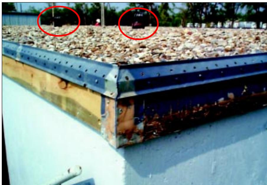
**FIGURE 6-14:** Ballast roof covering on a community shelter in Wichita, Kansas was a potential source of deadly windborne missiles to those seeking to access the shelter. Circles identify covers protecting roof penetrations intended for ventilation, but unable to provide adequate resistance to windborne debris.
