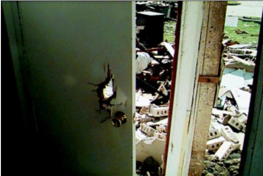
**FIGURE 4-27: A missile penetrated this exterior door in Del City, Oklahoma. Interior hollow-core doors typically offer even less missile protection than common exterior doors.**
