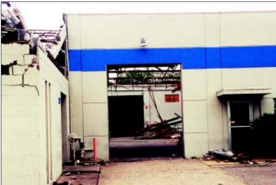
**FIGURE 5-19:** The tilt-up precast concrete walls in this building did not fail when the roof system failed. The masonry walls shown at the left of the photo were damaged. Note: many roof joists are still in place. Building was located in Wichita, Kansas, and was hit by weak tornado vortex.
