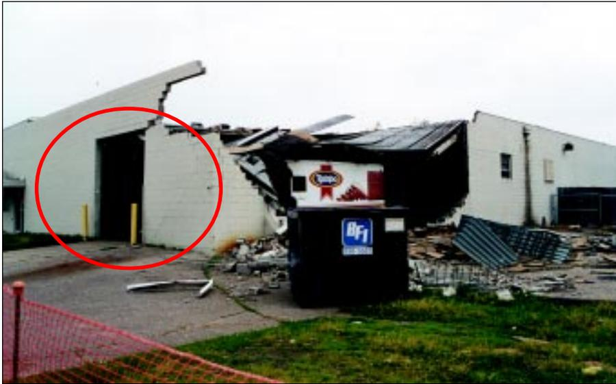
**FIGURE 5-30: Failure of roof and walls on structure due to increased loads caused by initial failure of a rollup door, Wichita, Kansas.**
