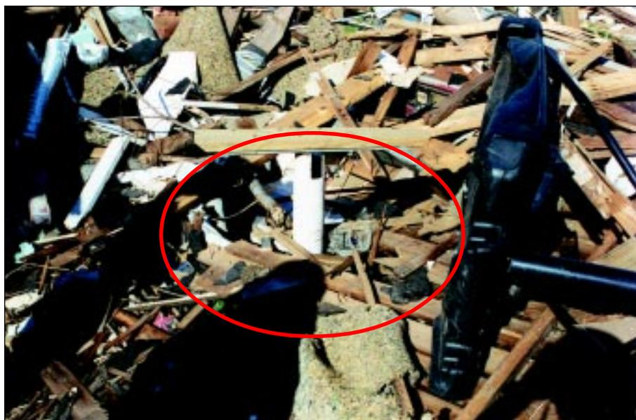
**FIGURE 6-17:** Heavy gauge ventilation pipe for a belowground shelter in Oklahoma withstood considerable debris impact.
