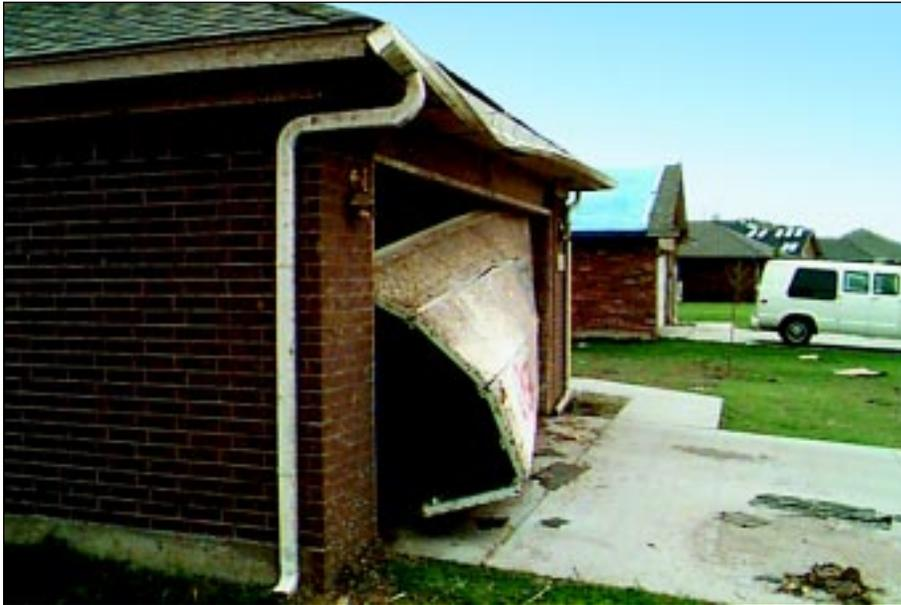
**FIGURE 4-18:** This double-width garage door failed under a suction load in Moore, Oklahoma.
