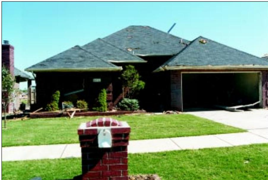
**FIGURE 4-24:** A view of home G with a garage door that failed due to positive (inward) acting wind loads.
