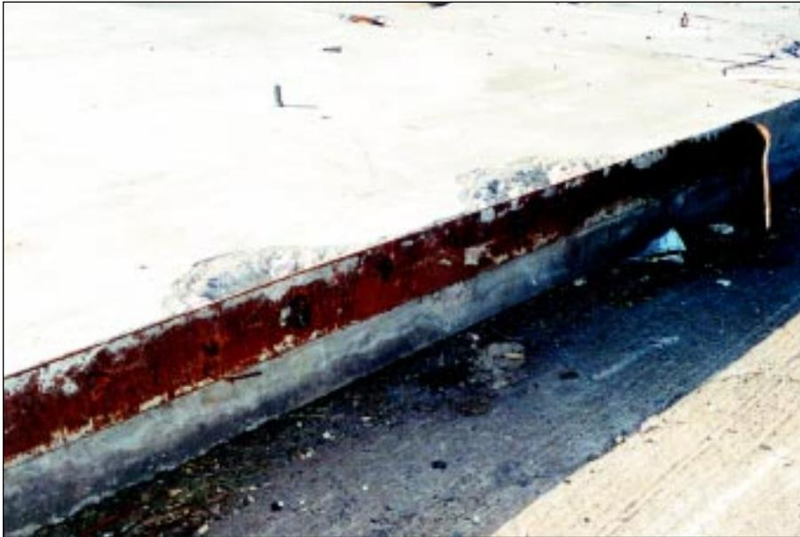
**FIGURE 5-18:** Top of failed tilt-up wall.
