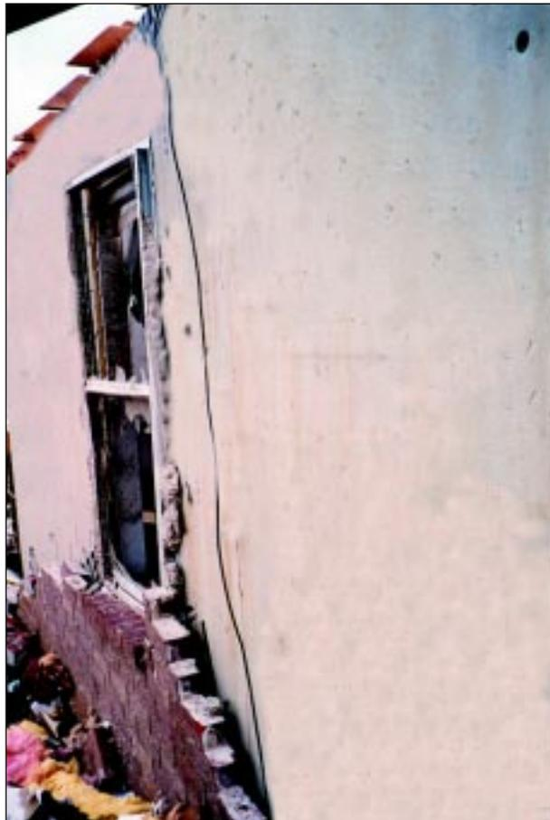
**FIGURE 4-35: Inadequate bonding of mortar to galvanized brick ties contributed to this masonry failure at a home in Bridge Creek, Oklahoma.**
