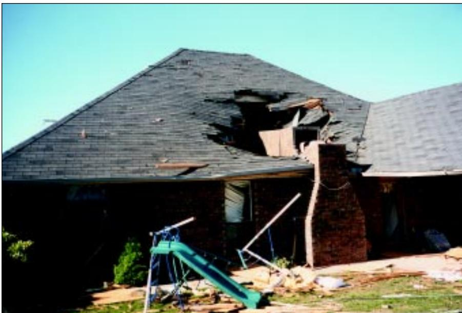
**FIGURE 4-42:** Failure of brick chimney onto top of home located along the periphery of a violent tornado, Moore, Oklahoma.
