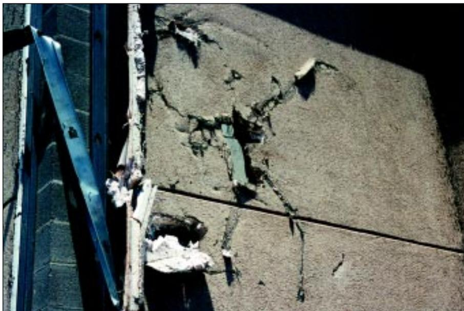
**FIGURE 6-37:** *This EIFS wall system was penetrated by numerous windborne missiles.*
