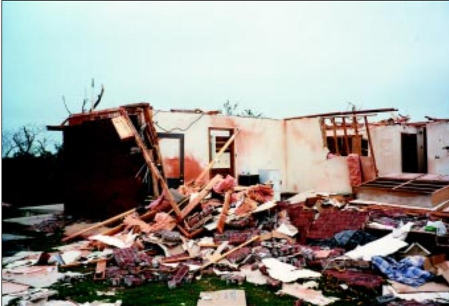
**FIGURE 4-32:** Failure of brick masonry veneer construction. The vortex of the strong tornado that caused the winds at this site passed approximately 300 feet from this building in Bridge Creek, Oklahoma.
