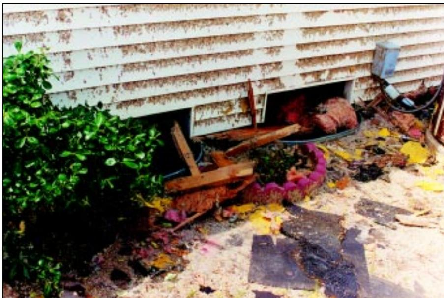
**FIGURE 6-26:** *Basement windows of a single-family residence, showing vulnerability to debris.*
