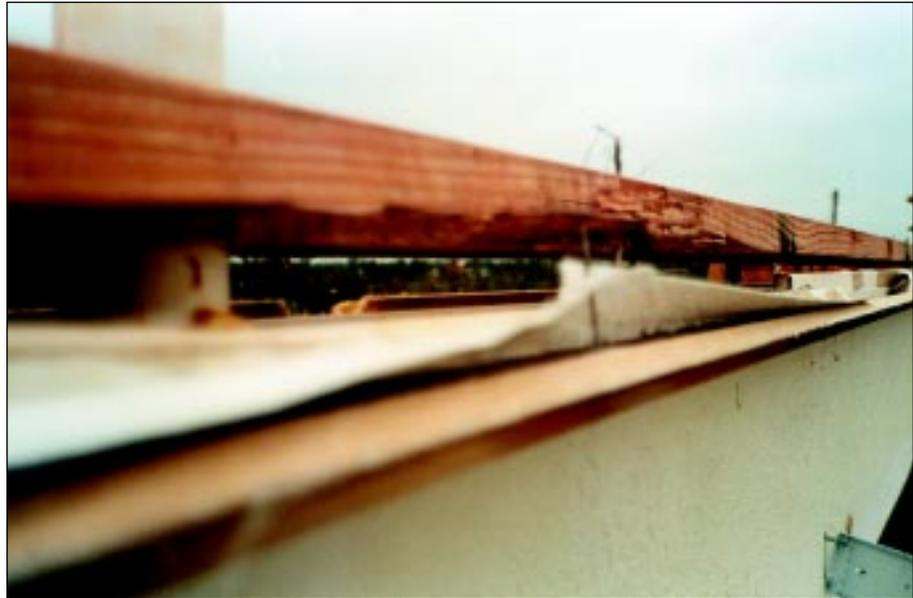
**FIGURE 4-9:** Failures of the connection of the double-top-plate to the supporting studs below at a home in Moore, Oklahoma. This home was located along the periphery of a violent tornado.
