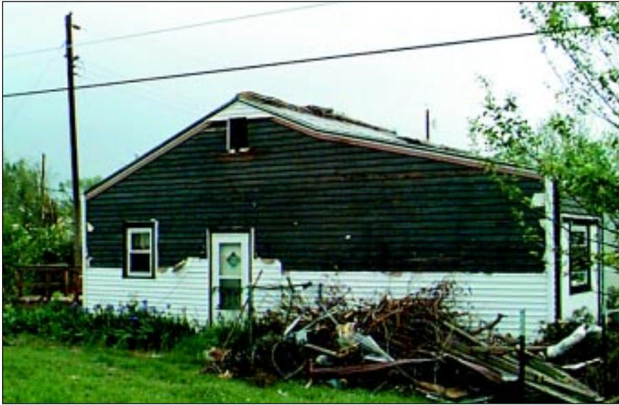
**FIGURE 4-16:** The vinyl (white) that was installed over wood siding experienced damage; however, the wood siding was undamaged. The home was located along the periphery of a violent tornado in Wichita, Kansas.
