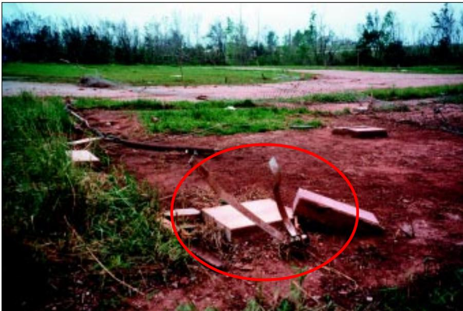
**FIGURE 4-48:** Failed straps at the anchorage of a manufactured home in Bridge Creek, Oklahoma. This site was 300-400 feet from a violent tornado vortex.
