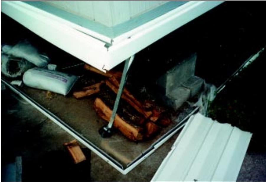
**FIGURE 4-58:** View of anchor strap and attachment indicating lateral shifting of a manufactured home, Haysville, Kansas. This home was located along the periphery of a violent tornado.
