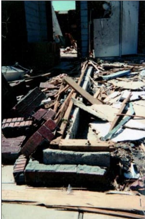
**FIGURE 4-13:** Failure of this bottom plate to wall stud connection occurred at this home outside Oklahoma City, Oklahoma. The vortex of a violent tornado passed very close to this home.
