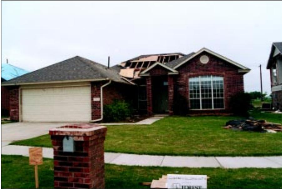
**FIGURE 4-29:** Front of home in Figure 4-28 where several pieces of roof sheathing failed.
