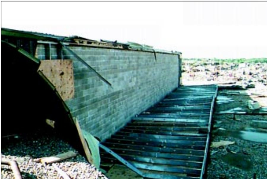
**FIGURE 5-28:** *This metal-clad wall covering collapsed and in other areas it was blown completely away.*
