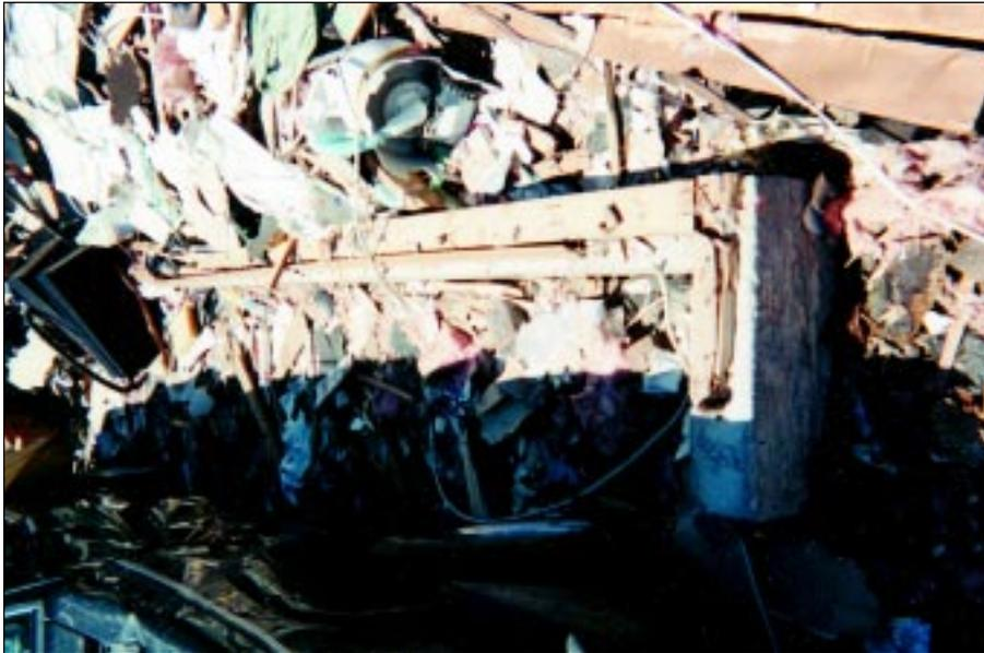
**FIGURE 4-10:** Wall framing to bottom plate failure. This house in Del City, Oklahoma, experienced a direct hit from the vortex of a violent tornado.
