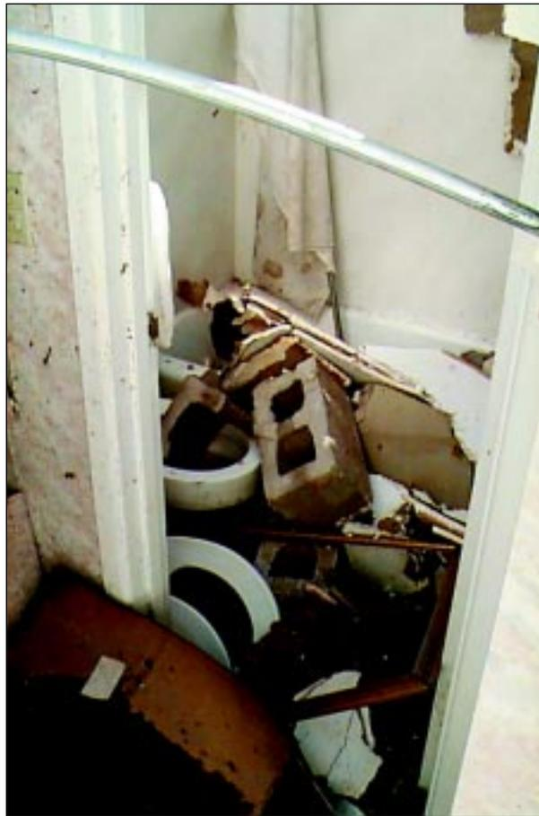
**FIGURE 6-39:** *The roof and ceiling over this interior bathroom blew off. CMU from a firewall a few feet away blew into the bathroom, which was located on a motel's second floor in Midwest City, Oklahoma. This bathroom would not have provided a safe refuge.*
