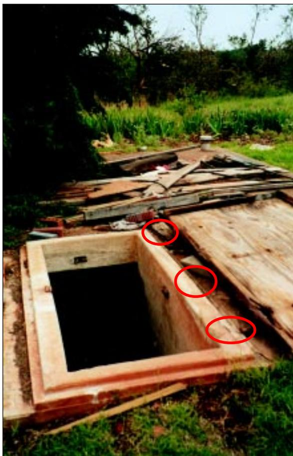
**FIGURE 6-11:** Door to underground shelter with rotting wood and corroded hinges.
