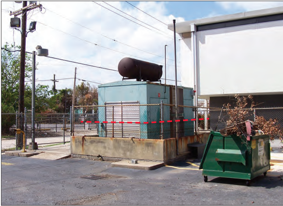
Figure 8-13. Flooded emergency generator at hospital in New Orleans (note flood line in red)
