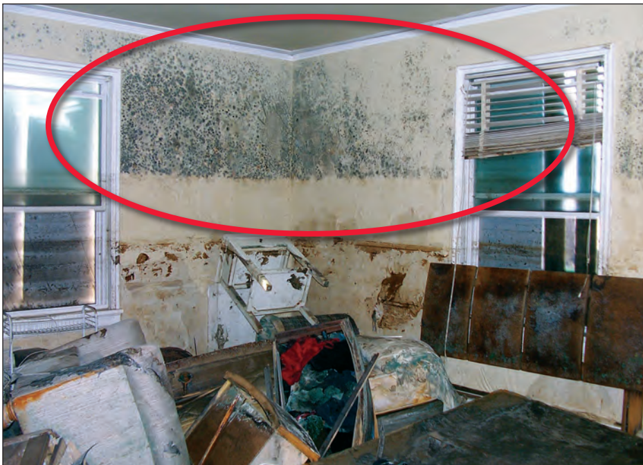
Figure 8-10. Typical interior flood damage to residential building in New Orleans, showing extensive mold growth (circle)
