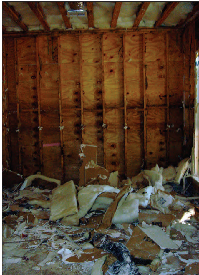
Figure 8-9. Exposed wall studs and sheathing boards in 2-year-old New Orleans residential building, showing no significant deterioration from long-duration flooding.
