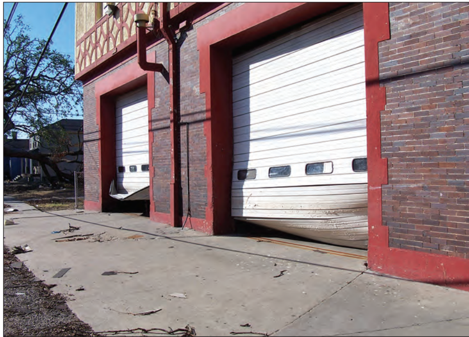
Figure 8-12. Damage to garage bay doors at fire station in New Orleans. The door on the right was pushed in by flooding; the door on the left appears to have been pulled open from the outside by looters.
