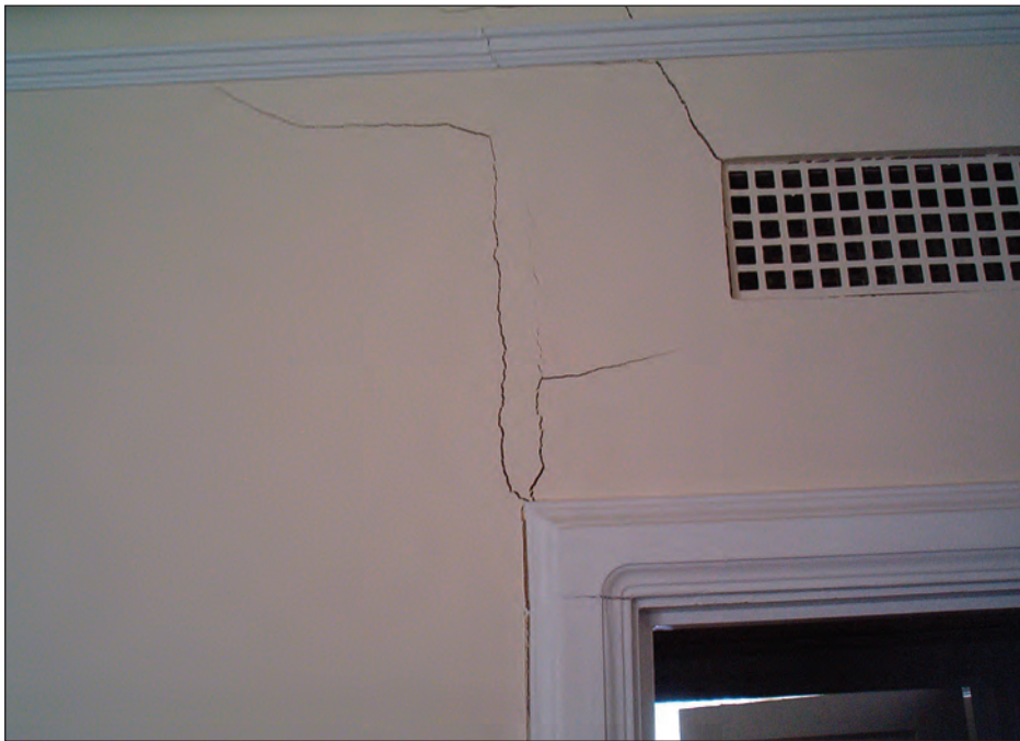
Figure 8-7. Settlement cracks in upper floor wall of New Orleans residence due to subsidence/differential settlement of underlying foundation soils during long-duration flooding
