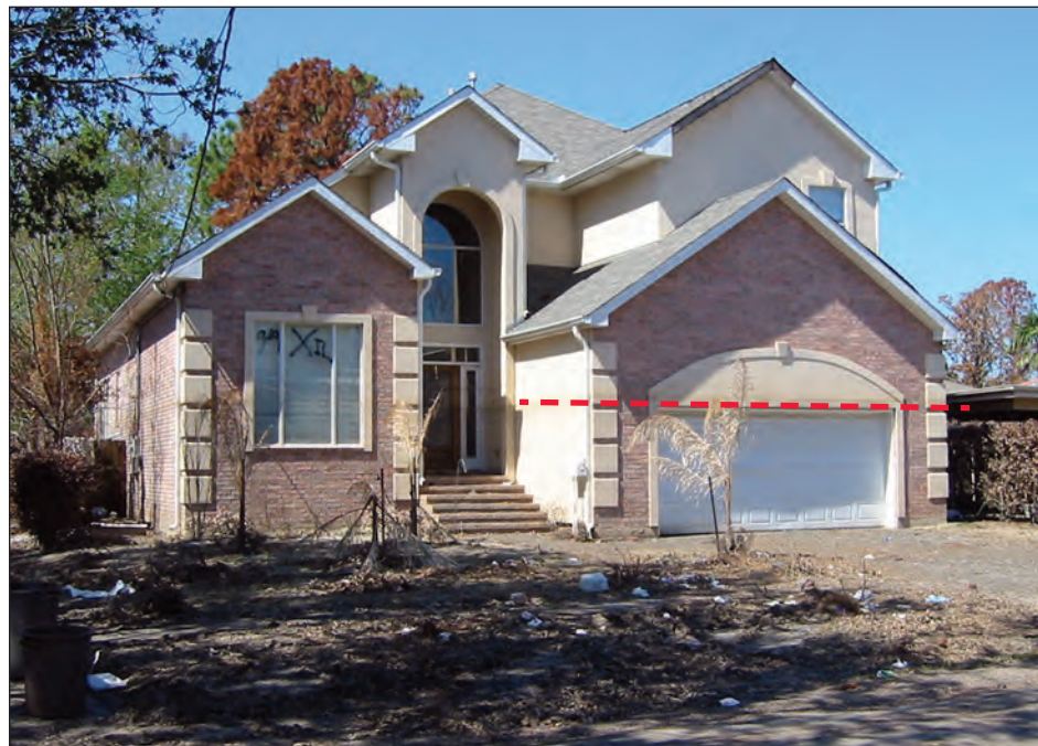
Figure 8-3. Residential building constructed approximately 1 foot above the BFE in accordance with current codes. Note flood depths were even with the top of the garage door, or about 3-5 feet above the first floor (red line).
