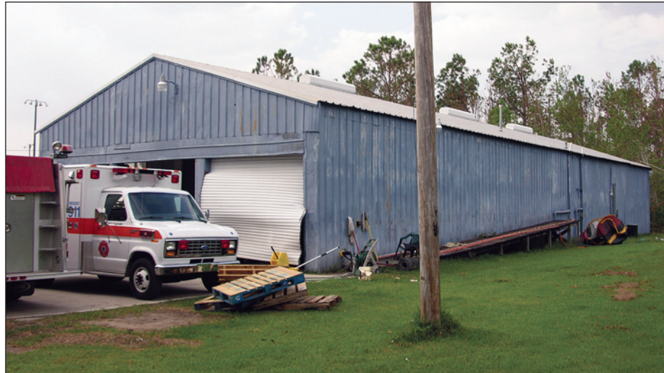
Figure 7-11. General view of the Cuevas Volunteer Fire Department. Note the damaged apparatus bay door (estimated wind speed: 130 mph. Pass Christian, Mississippi).
