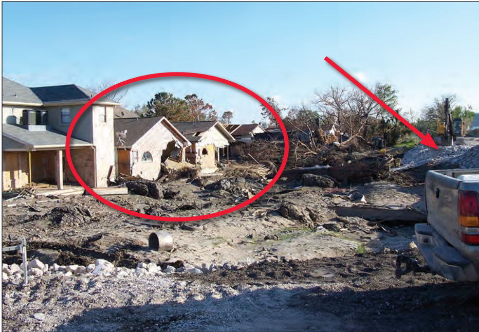
Figure 8-6. Structural damage to residential buildings (circle) in New Orleans located immediately behind the site of 17th Street Canal levee breach (arrow)
