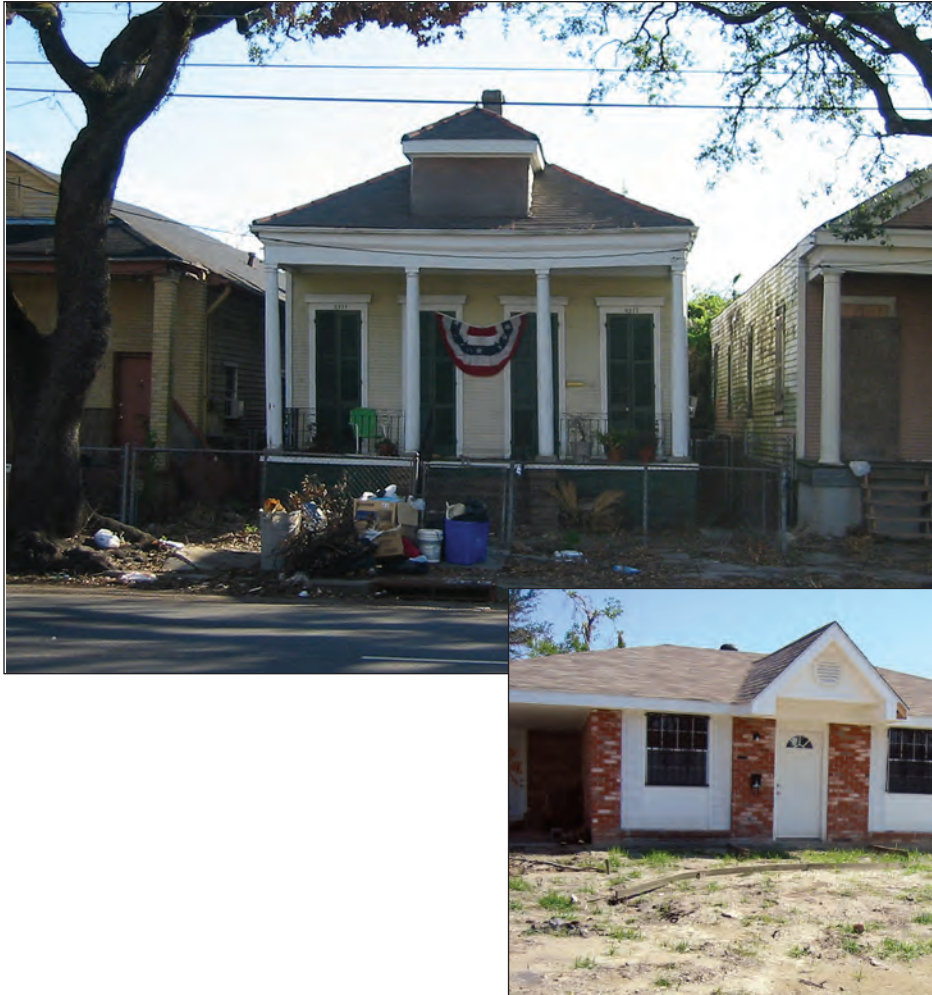
Figure 8-4. Comparison of building techniques in New Orleans. The older residence on the upper left has the first finished floor constructed several feet above grade. The newer residence on the lower right is constructed with a slab-on-grade foundation.
