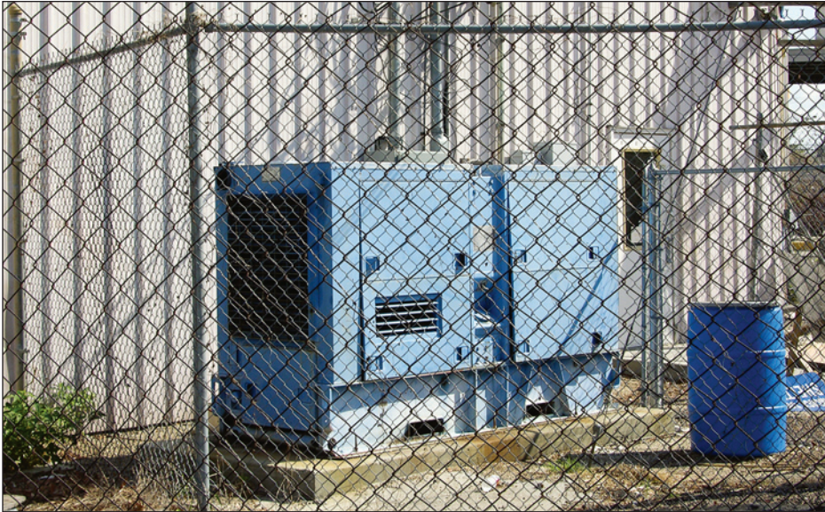
Figure 7-5. The EOC's emergency generator was exposed and inundated by floodwater (Bay St. Louis, Mississippi).
