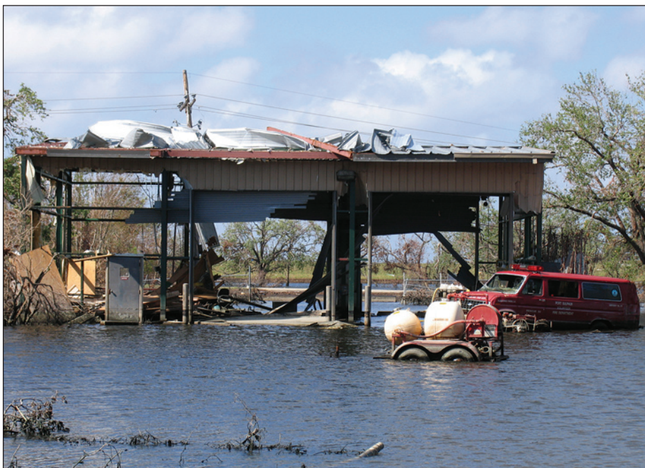
Figure 7-15. General view of the Port Sulphur Volunteer Fire Department showing damage caused by storm surge and wind. Note the inundated apparatus in the foreground (estimated wind speed: 125 mph. Port Sulphur, Louisiana).
