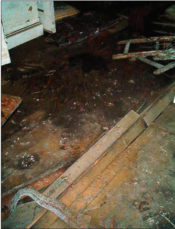
Figure 8-15. Flood residue and buckled floor observed on General Diaz Street. A sample of the flood residue was collected for analysis.
