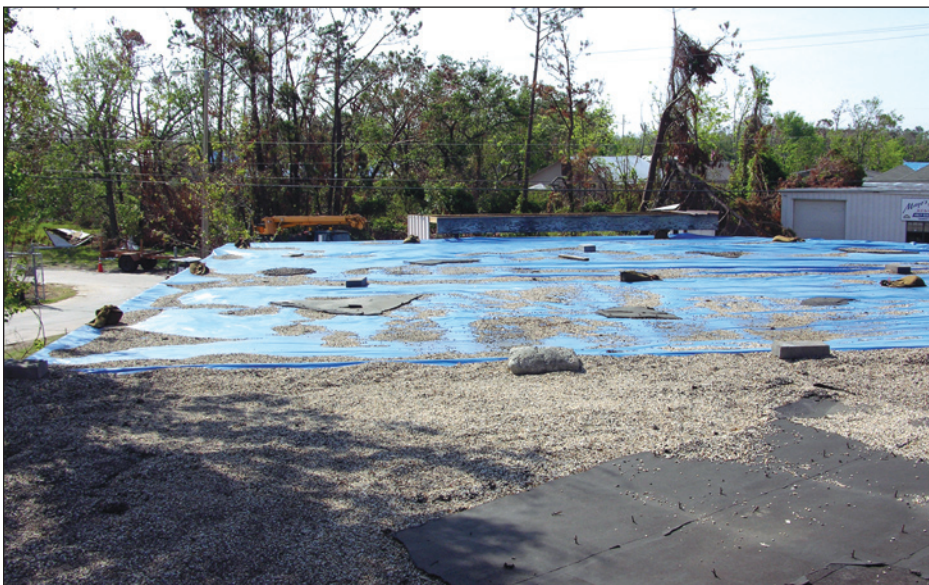
Figure 7-6. The blue tarp was used as an emergency repair where the roof membrane blew off the EOC. Although the membrane's base sheet fasteners were too far apart, the failure initiated with lifting and peeling of the metal edge flashing (estimated wind speed: 125 mph. Bay St. Louis, Mississippi).
