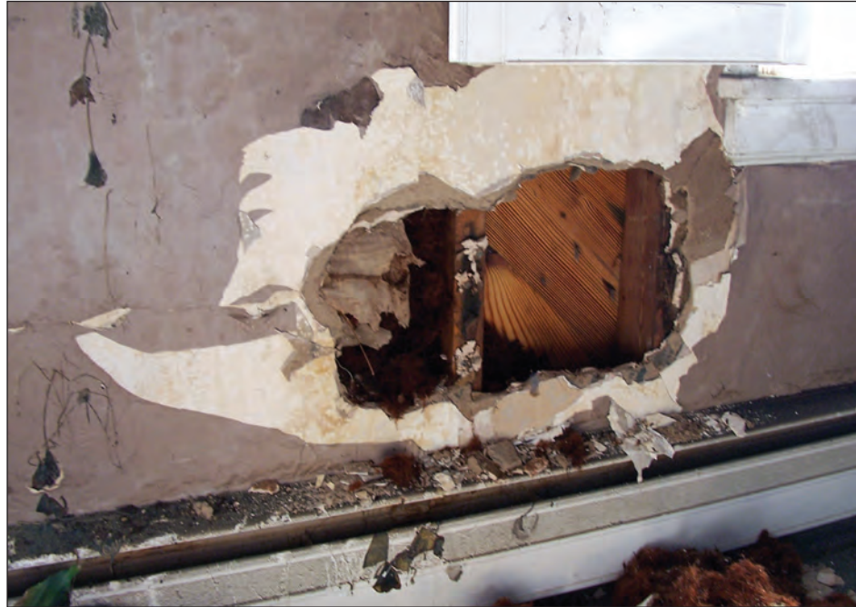
Figure 8-9. Exposed wall studs and sheathing boards in 2-year-old New Orleans residential building, showing no significant deterioration from long-duration flooding.
