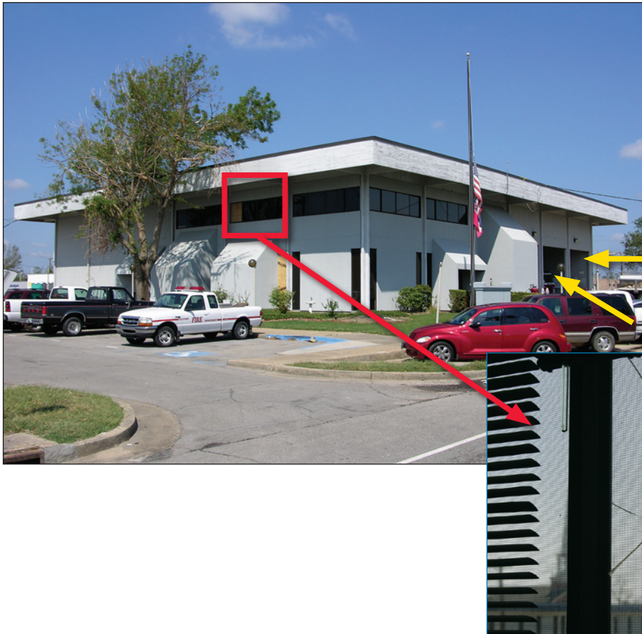
Figure 7-8. General view of Gulfport Fire Station #1. Three of the sectional doors blew in (yellow arrows), and four windows were broken on the left side of the building (square/inset) (estimated wind speed: 130 mph. Gulfport, Mississippi).
