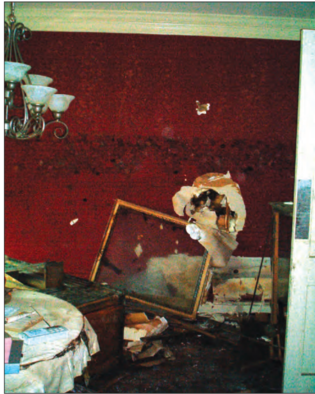
Figure 8-16. Samples were collected from wall materials both above and below the waterline as shown on this wall of a house on Memphis Street. Where practical, samples were collected from surfaces that were already substantially damaged or scheduled for tear-out.
