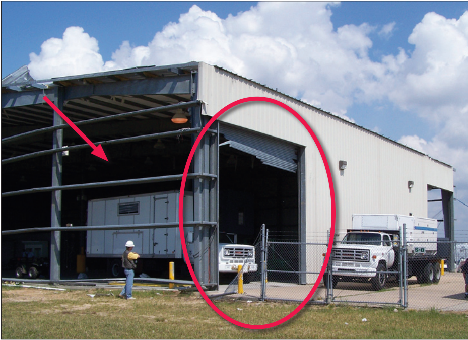
Figure 7-22. Wind damage to the southwest corner of the airport cargo building. Note the pressure damaged rolling door (circle) and the west wall panels removed by combined internal and external pressures (arrow) (estimated wind speed: 130 mph. Gulfport, Mississippi).
