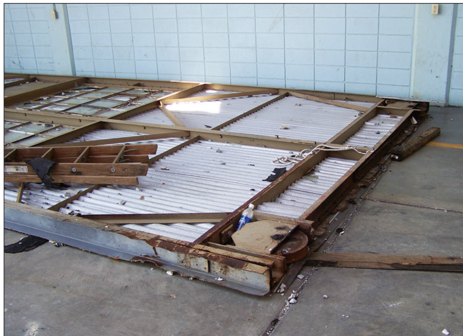
Figure 7-25. Sliding door blown into hangar (estimated wind speed: 130 mph. Gulfport, Mississippi)
