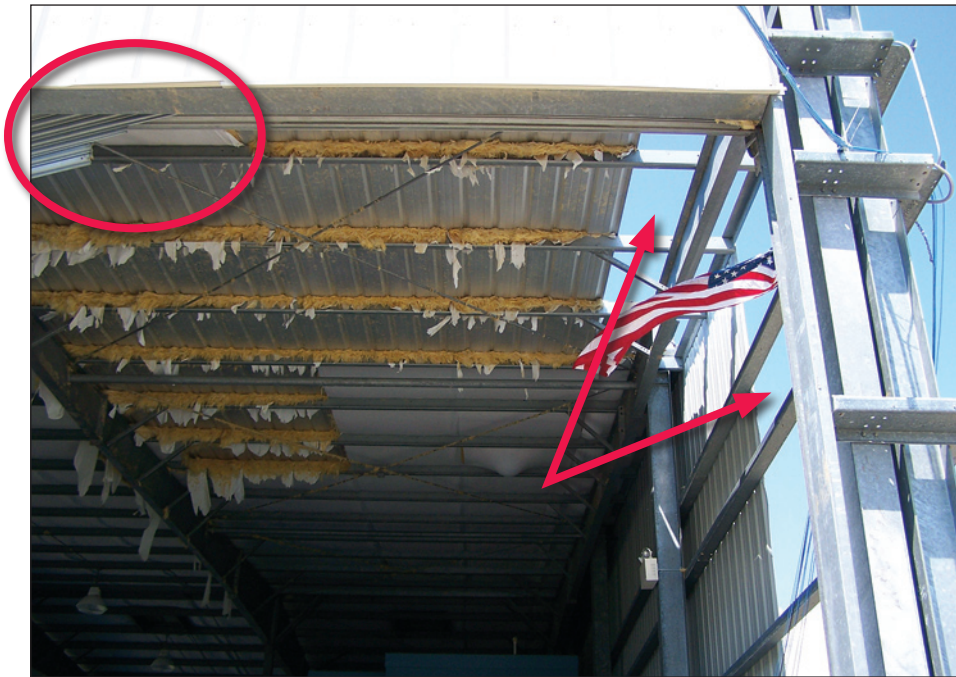
Figure 7-23. Roof and wall panel damage at the airport cargo building. Note the damaged rolling door at the southeast corner (circle) and roof and wall damage (arrows) (estimated wind speed: 130 mph. Gulfport, Mississippi).
