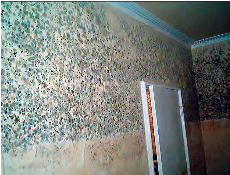
Figure 8-19. The mold growth on the walls was generally much more vigorous above the floodwater level than below it. Sediments, heavy metal contamination, and oil film residue, as well as material moisture content and lack of exposure to air during flooding, may contribute to minimizing the fungal growth on the saturated wall materials.
