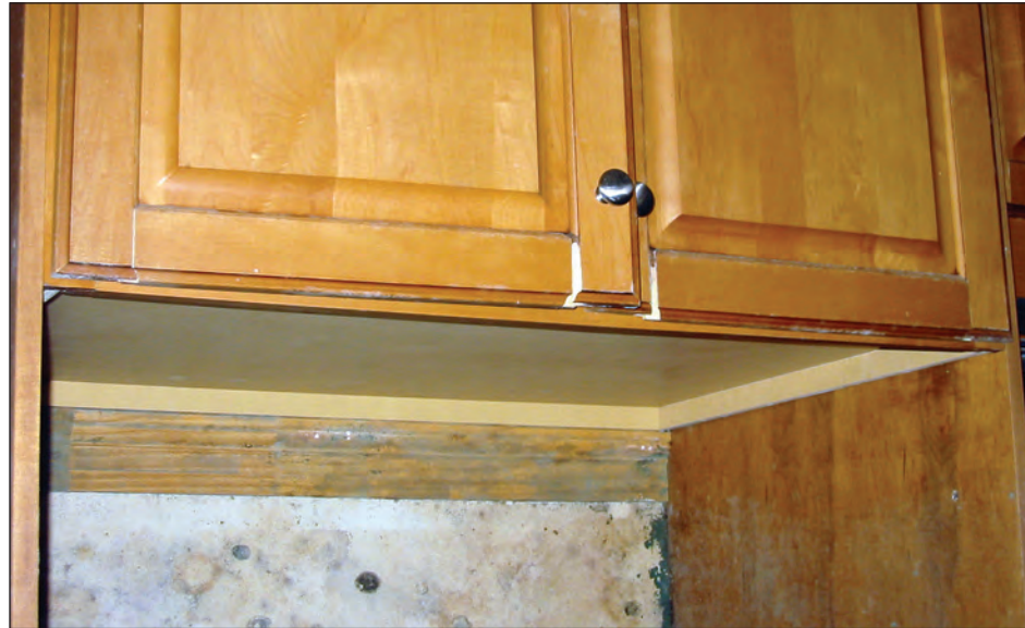
Figure 8-14. Kitchen cabinet doors above the flood level were damaged from the excessive moisture in the house from long-duration flooding.
