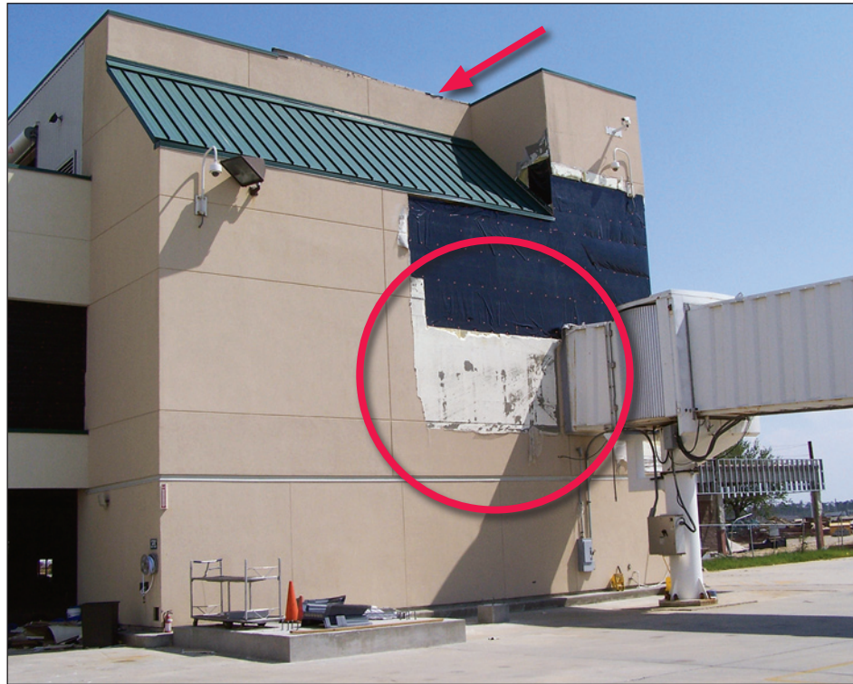
Figure 7-20. Damaged terminal gate at the Gulfport-Biloxi International Airport. Note the damaged roof coping (arrow) and the wind damaged EIFS (circle) (estimated wind speed: 130 mph. Gulfport, Mississippi).
