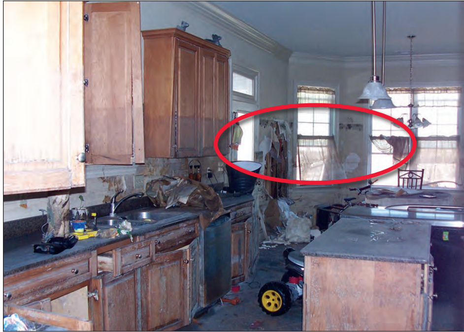
Figure 8-11. Typical interior flood damage to residential building in New Orleans, showing light mold growth (compare to Figure 8-10)
