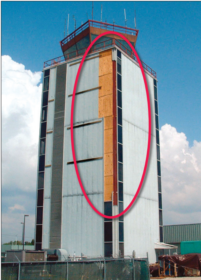
Figure 7-19. Airport control tower. Note damaged glazing and cladding (circle) (estimated wind speed: 130 mph. Gulfport, Mississippi).
