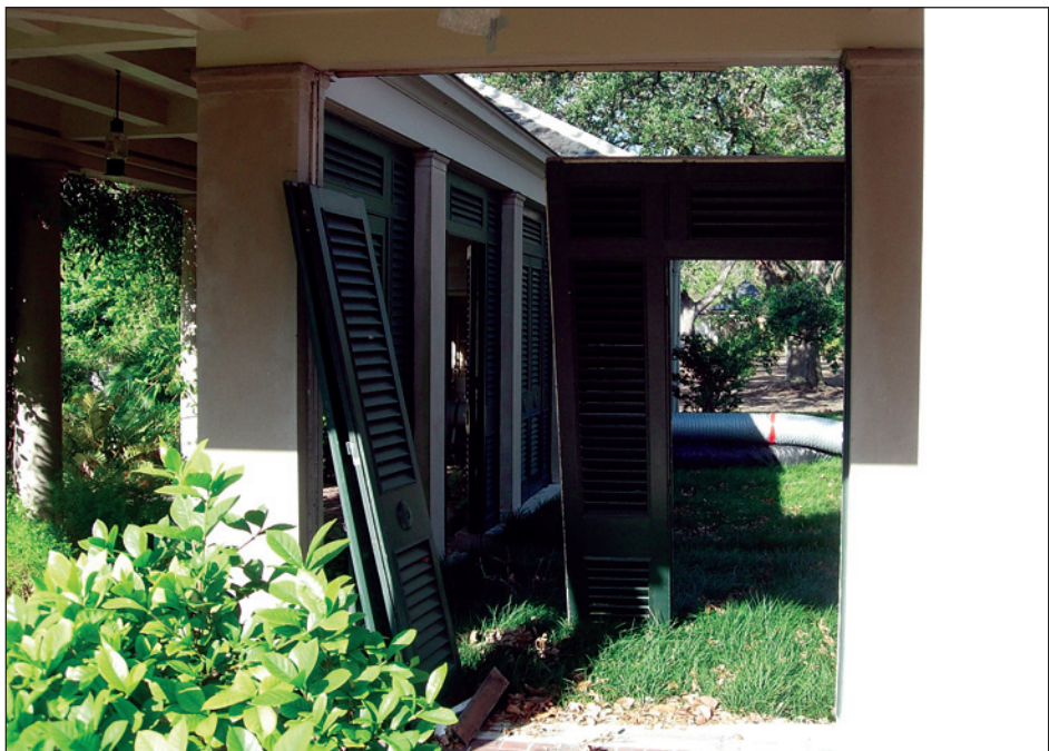
Figure 6-22. View of wind damage to shutters of Longue Vue after Hurricane Katrina (New Orleans, Louisiana)
