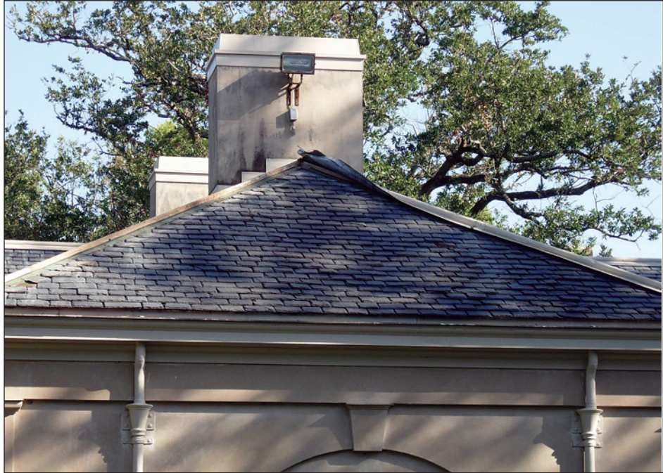
Figure 6-21. View of wind damage to flashing along rake of Longue Vue after Hurricane Katrina (New Orleans, Louisiana)
