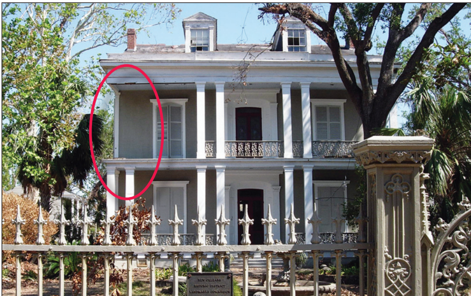
Figure 6-16. Wind damage to the second floor columns of the Benachi House. Note missing columns (circle) (New Orleans, Louisiana).
