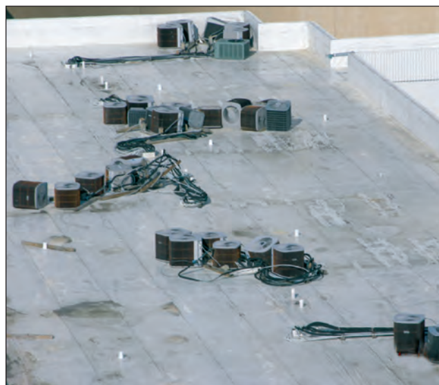
Figure 6. Sleeper-mounted condensers displaced by high winds.
