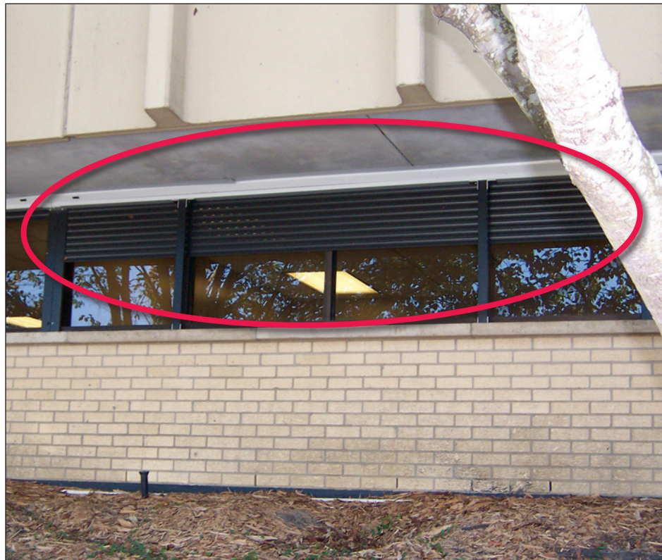
Figure 9-12. Closeup of the roll-down metal shutters on the Harrison County Courthouse building. Note the partially lowered shutters on the middle windows (circle) (estimated wind speed: 130 mph. Gulfport, Mississippi).
