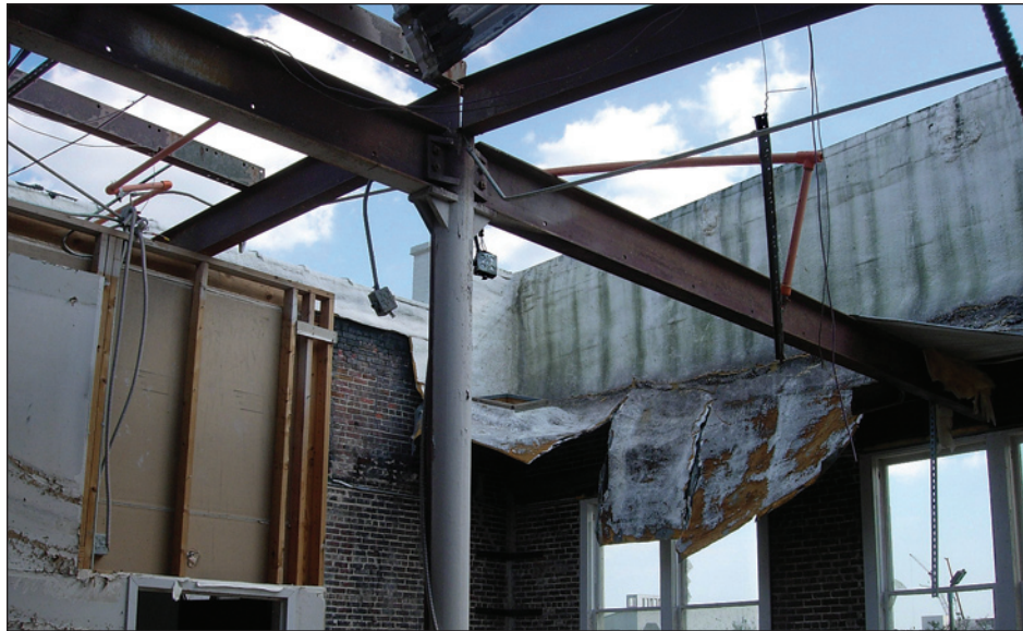
Figure 6-14. Interior view of the Kress Building showing roof torn away (Biloxi, Mississippi)
