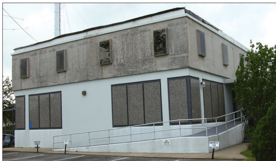
Figure 9-15. Exterior view of the Jackson County EOC. Note the polycarbonate shutters over the windows (estimated wind speed: 105 mph. Pascagoula, Mississippi).
