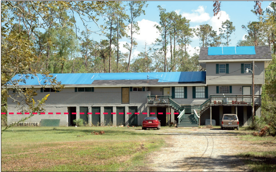
Figure 9-5. Post-Katrina photo of an HMGP-elevated house. Note the estimated water line associated with Hurricane Katrina (red line) (Lacombe, Louisiana).
