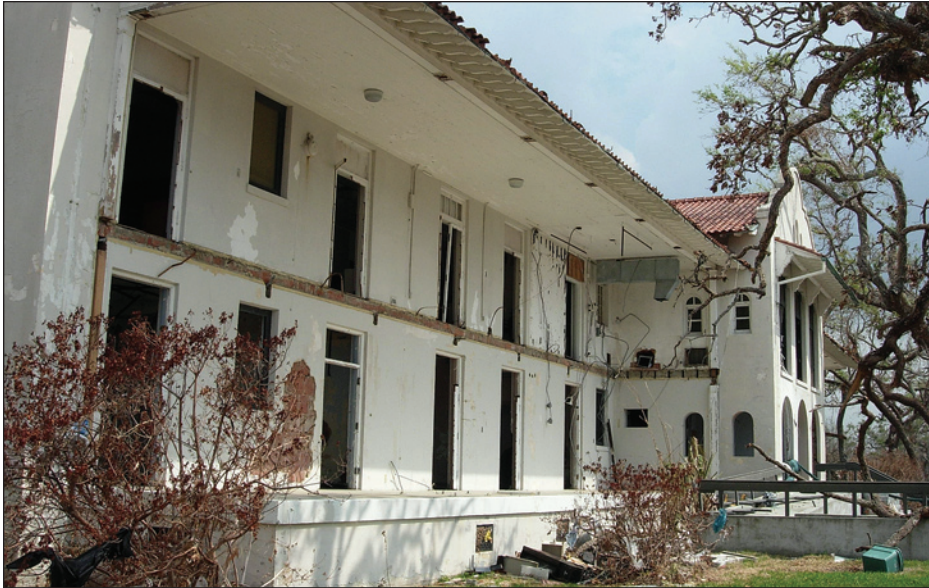
Figure 6-15. Loss of the entire second floor porch and roof supports to flooding; the main roof stayed successfully intact due to integral framing of the roof structure (Gulfport, Mississippi).
