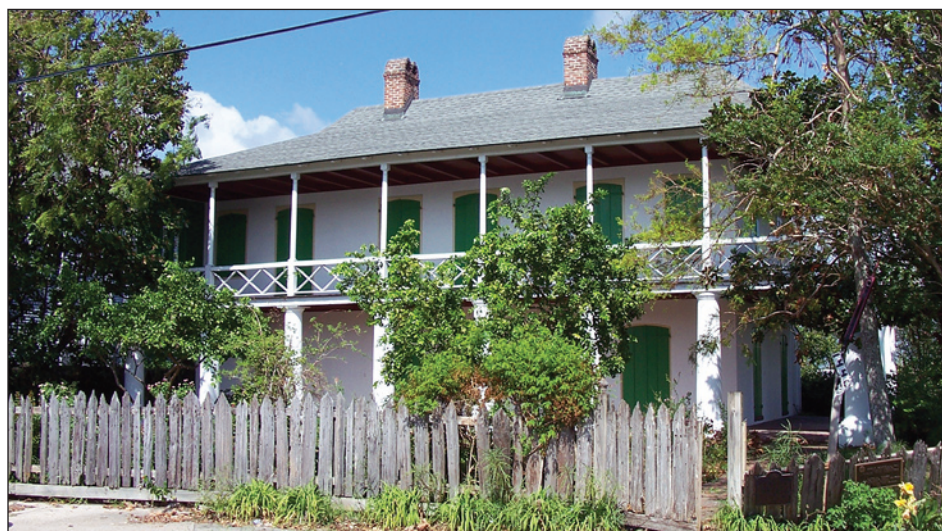
Figure 6-18. Front elevation of Pitot House showing damage to the front wood fence. The house survived very well, with no evidence of flood damage and little wind damage (New Orleans, Louisiana).
