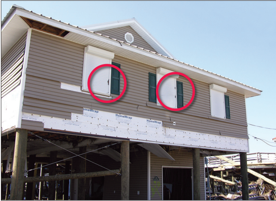
Figure 9-19. The black area at the left window and the two black areas at the middle window (circles) are pieces of asphalt shingle debris. Had the windows not been protected by shutters, they would have likely been broken by windborne debris (estimated wind speed: 125 mph. Shell Beach, Louisiana).
