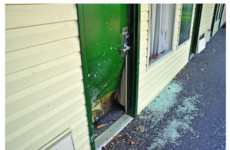
Figure B8-18: This metal door was damaged by wind-borne debris generated by a weak tornado. The bottom hinge was damaged, but the single latch was able to resist the modest wind and impact load. The door was on the verge of failing. (St. Louis, Missouri, 2013 tornado)
