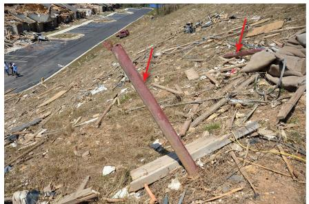
Figure B8-14: Steel porch column debris from an apartment complex where columns that were 7 feet 9 inches long and 4¼ inches in diameter (see red arrows) had a significant upward trajectory and flew approximately 230 feet (Tuscaloosa, Alabama, 2011 tornado)
