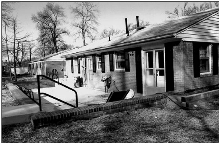
Figure 6-55. Brick-faced residential floodwall and access stairs
