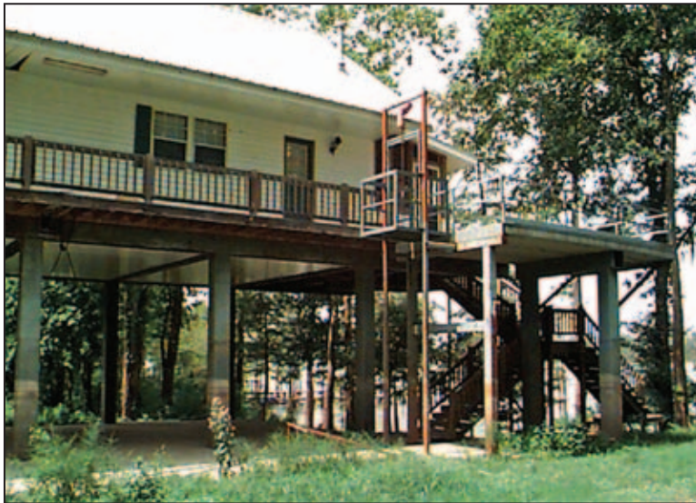
Figure 6-28. House elevated on timber piles
