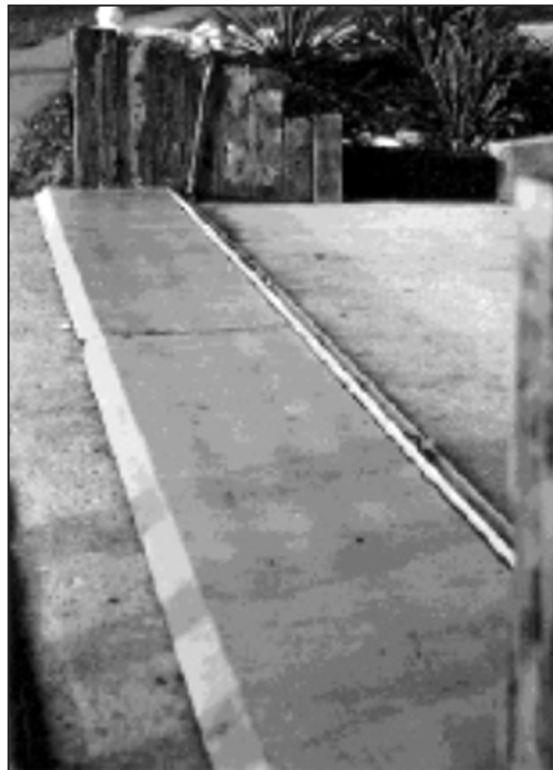
Figure 5D-4. A shield hinged at its bottom could prevent low-level flooding from entering a garage or driveway.
