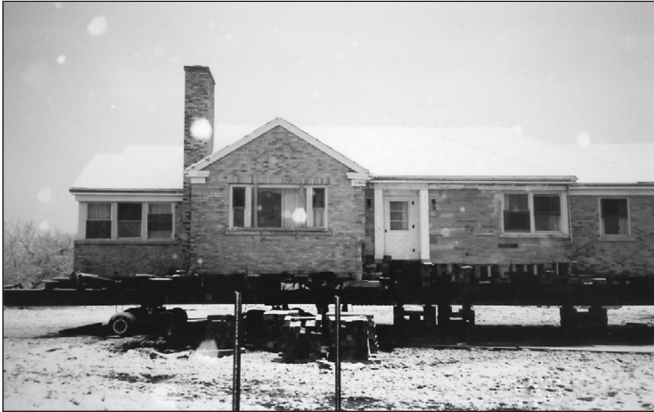
Figure 1-7. Structure placed on a wheeled vehicle for relocation to a new site
