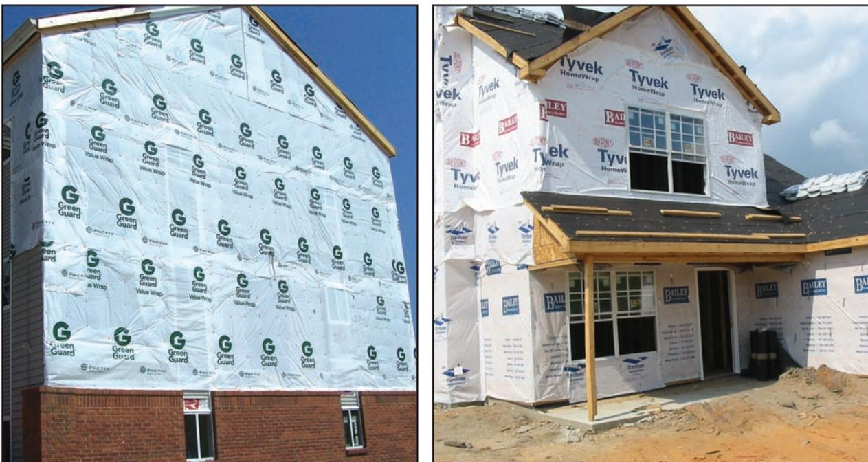
Figure 9-1 and 9-2. Examples of moisture barrier systems. (Source: FEMA 549)
