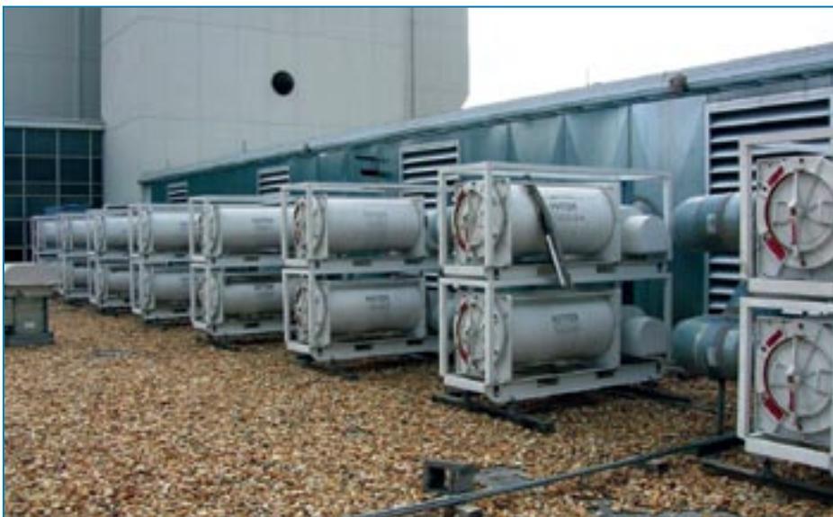
**Figure 4-8:** Radial-flow adsorbers in multiple 1,000-cfm housings in a 16,000-cfm system serving a hospital.
