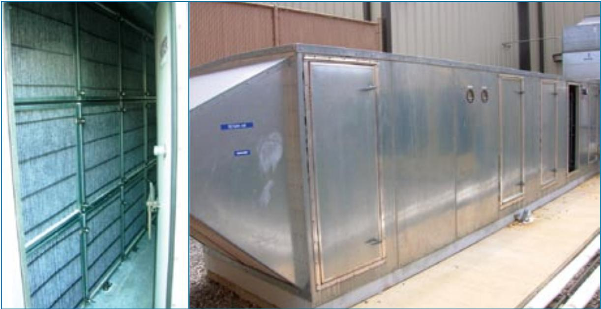
**Figure 4-6:** 9,000-cfm filter unit incorporating pleated adsorbers.
