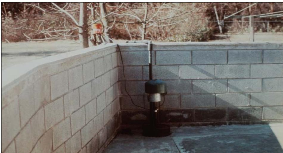
**Figure 5-7. Small patio floodwall with sump pump**
