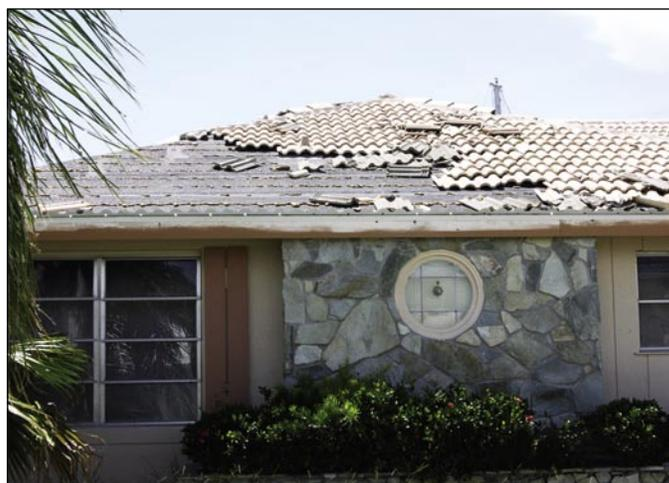
**Uplift loads and resistance:** Calculate uplift loads and resistance in accordance with the “Design and Construction Guidance” section below. Load and resistance calculations should be performed by a qualified person (i.e., someone who is familiar with the calculation procedures and code requirements).
