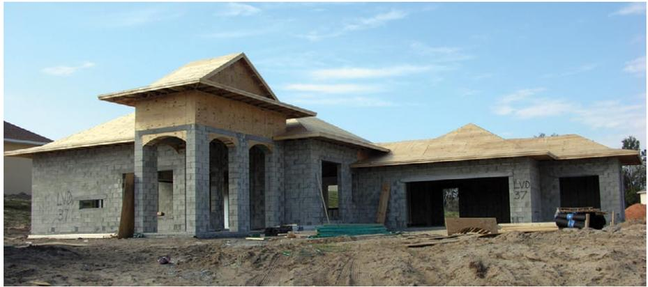
**CMU was used for the exterior walls at this house under construction (New Smyrna Beach, FL).**
