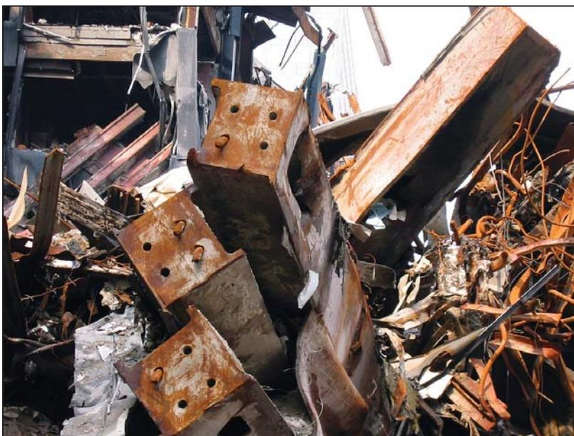
Figure B-1 Exterior column end plates.
