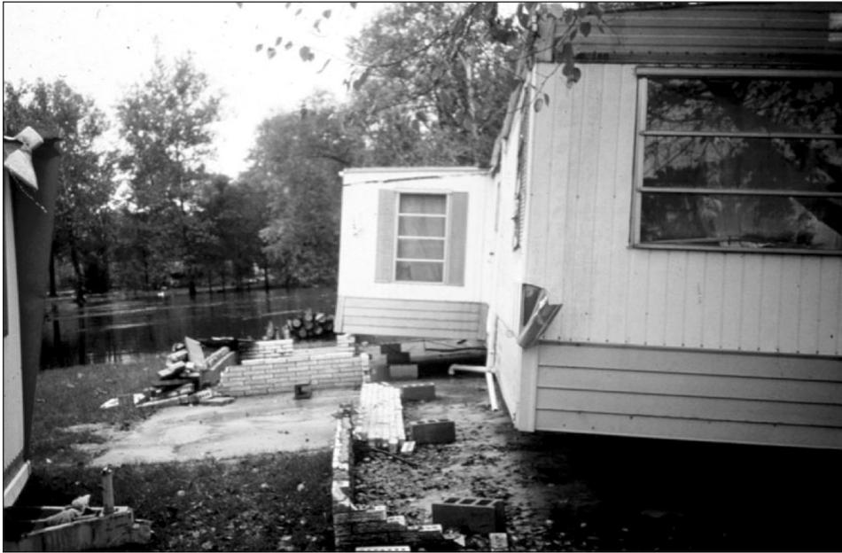
Figure 9-1. A home that was partially submerged and displaced from its foundation by hydrostatic forces. Although it appears the openings are too high, the bottoms of the openings are less than 1 foot above the top of the interior slab.
