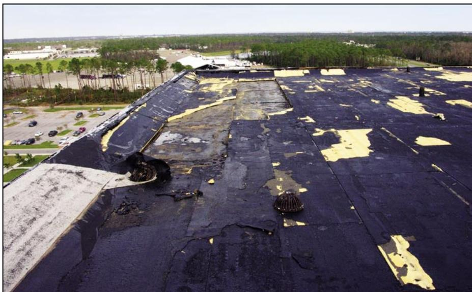
**Figure 6-3.** General view of upper roof of the Pensacola Naval Hospital. Note the missing insulation boards near the corner of the roof. (Pensacola)
