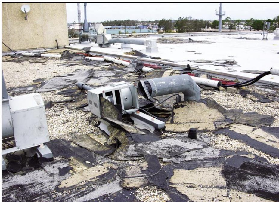
Figure 6-1. General view of the roof membrane and rooftop equipment damage at the Escambia County Sheriff's Office/EOC. The roof at the upper right is on the new addition. The mineral surfaced BUR landed on an aggregate surfaced BUR. (Pensacola)
