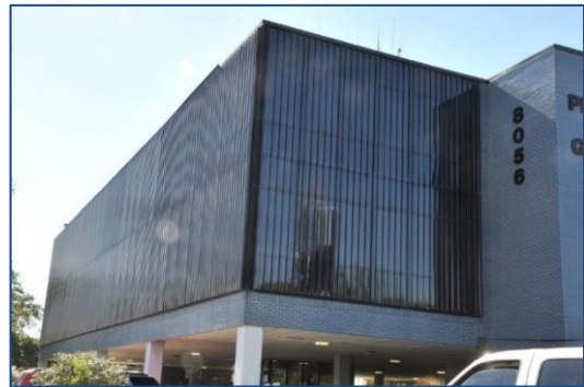
Government building outfitted with storm panels that can withstand winds up to 120 mph.
