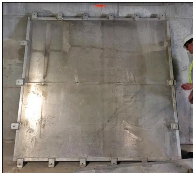
**Figure 1: Large (6 feet high x 6 feet wide) metal flood panel requiring special equipment for installation**
