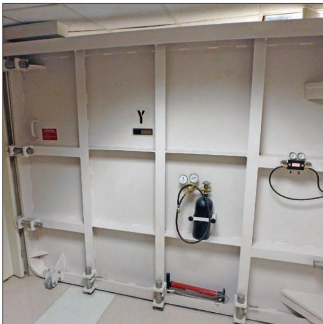
**Figure 7: Flood gate with an air tank and a hand pump as a redundancy measure to inflate gaskets**
