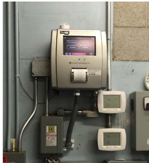
Fig 3 Fuel Monitoring System
