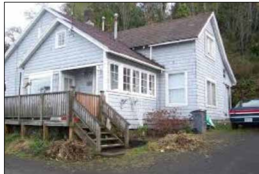
Figure 4: Back and west side of the house
