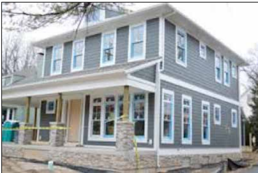
Figure 3: Front and east side of the building
